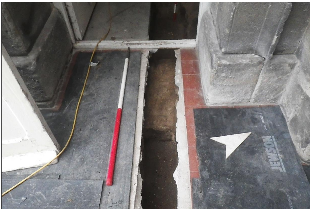
Plate 2: ceramic tiling and concrete floor in the lean-to structure and passage with wall footing 1000 visible beneath.
