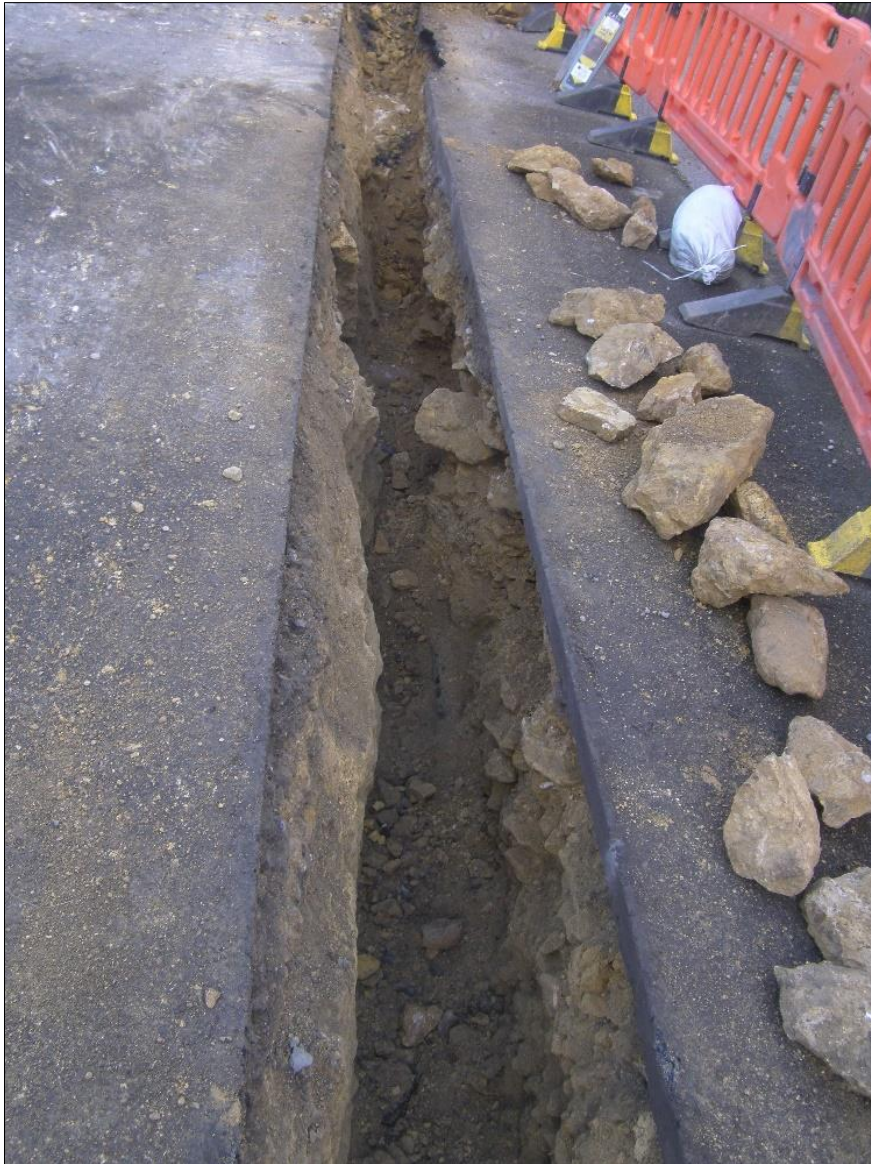
Plate 1: the 1930s rock-cut pipe trench under excavation.
