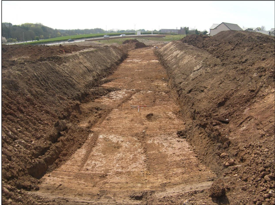
Plate 1: Street footprint excavated through 2.5m overburden, looking south-west
