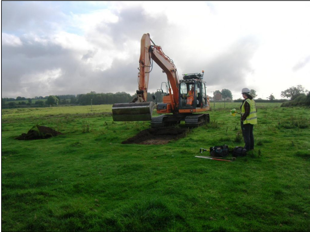
Plate 1: Mechanical stripping of topsoil and subsoil
