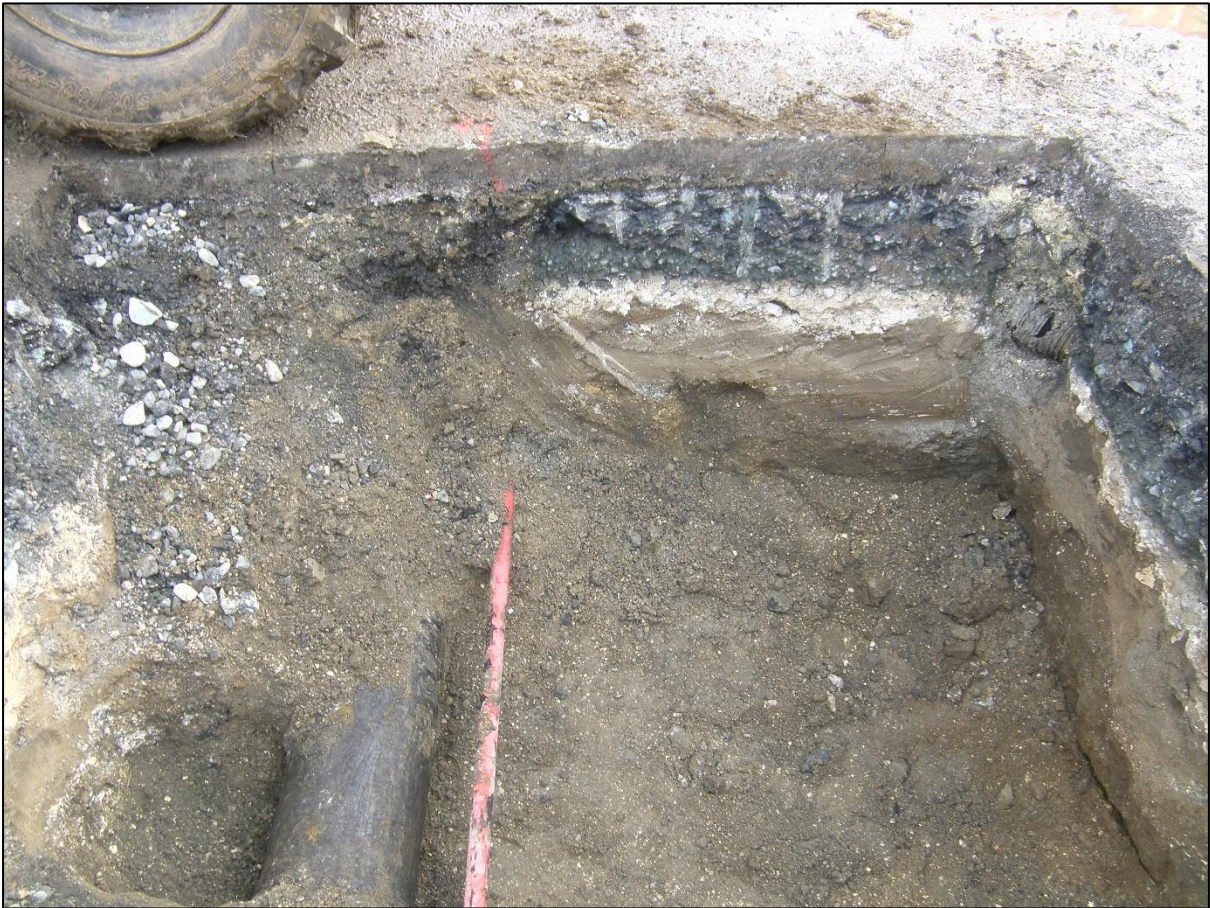
Plate 2: Trench 2, Pit 2 showing tarmac surface, existing water main and modern backfill.
