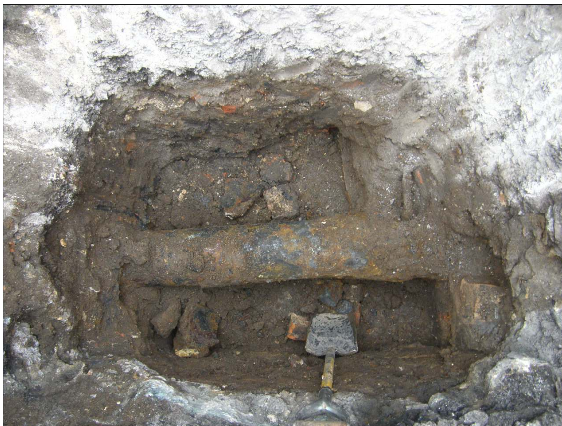
Gillygate, York: typical pit profile showing made ground and water main
