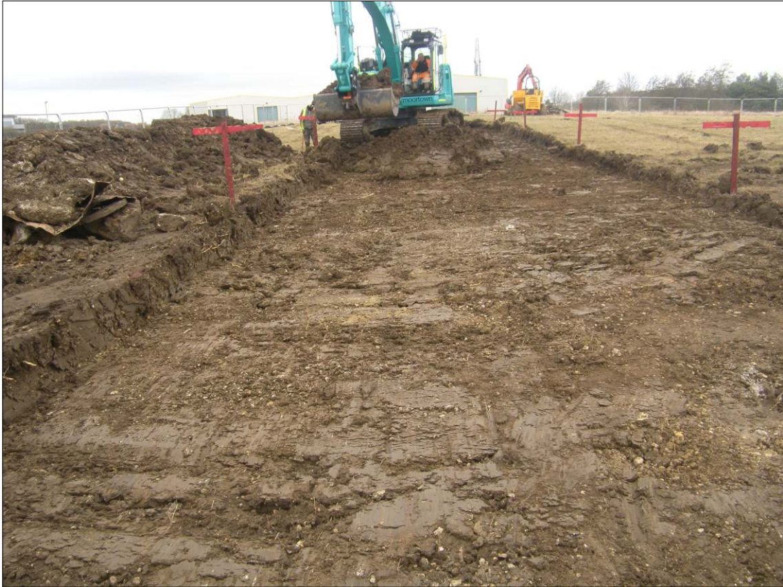
Goole Business and Innovation Centre: working shot during machine stripping
