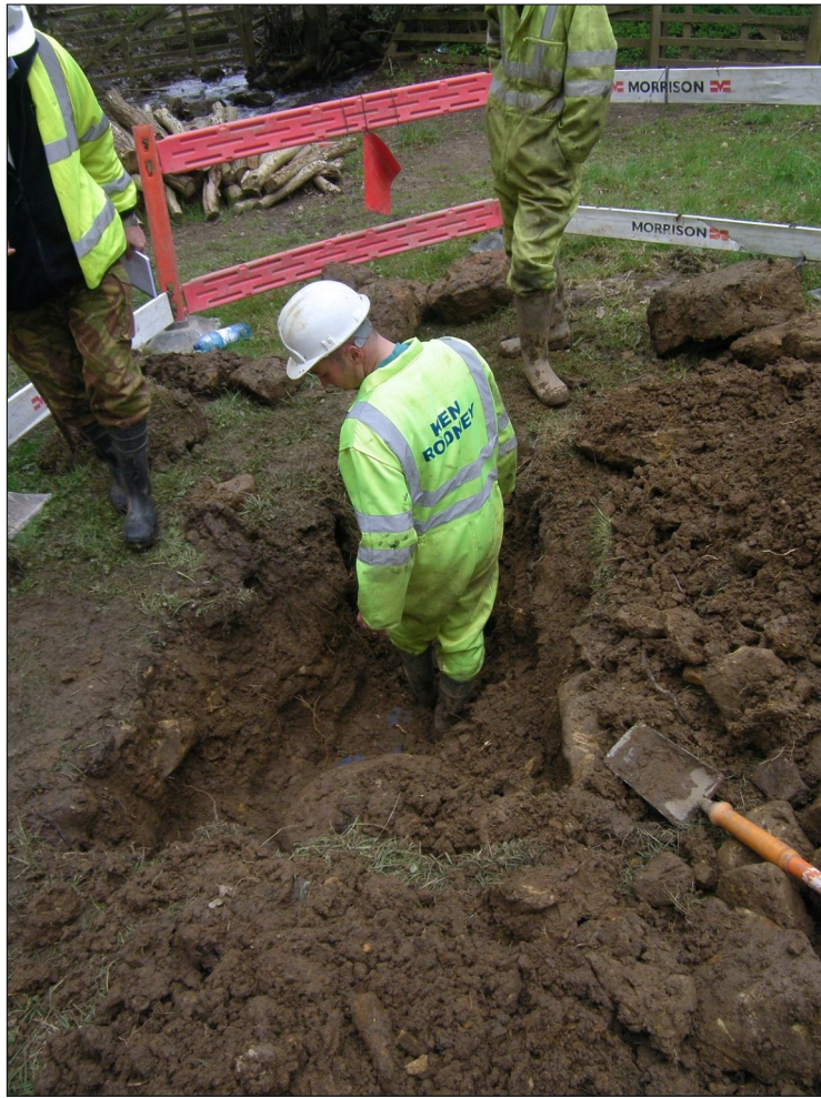
Randy Mere to Ruswarp Water Main: hand-excavation of inspection trench
