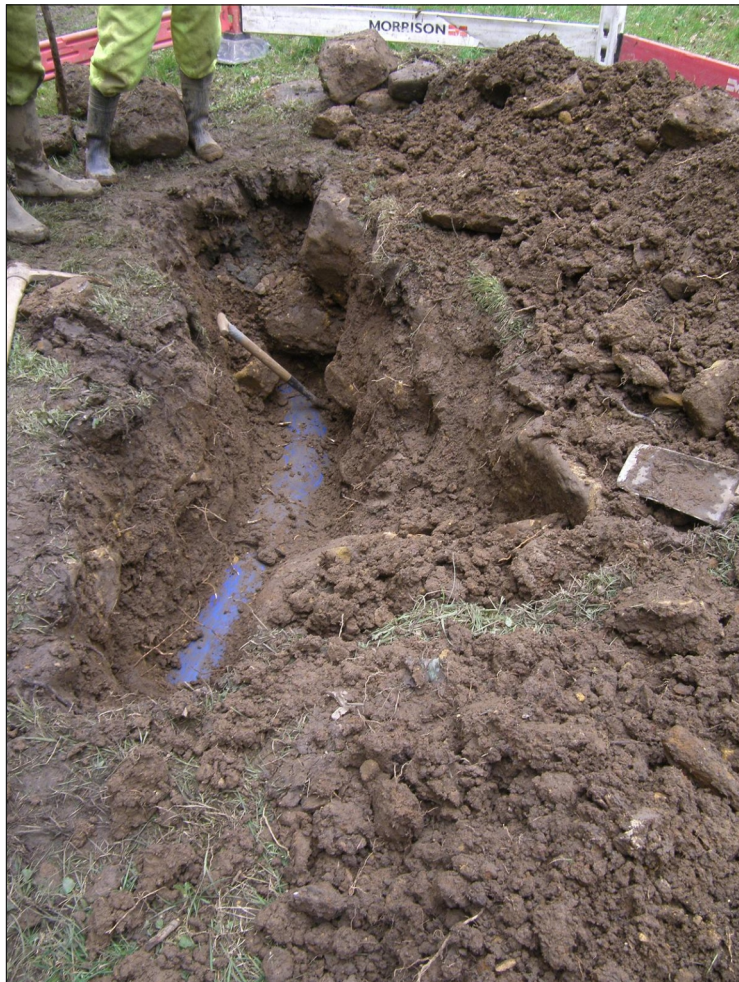
Randy Mere to Ruswarp Water Main: inspection trench
