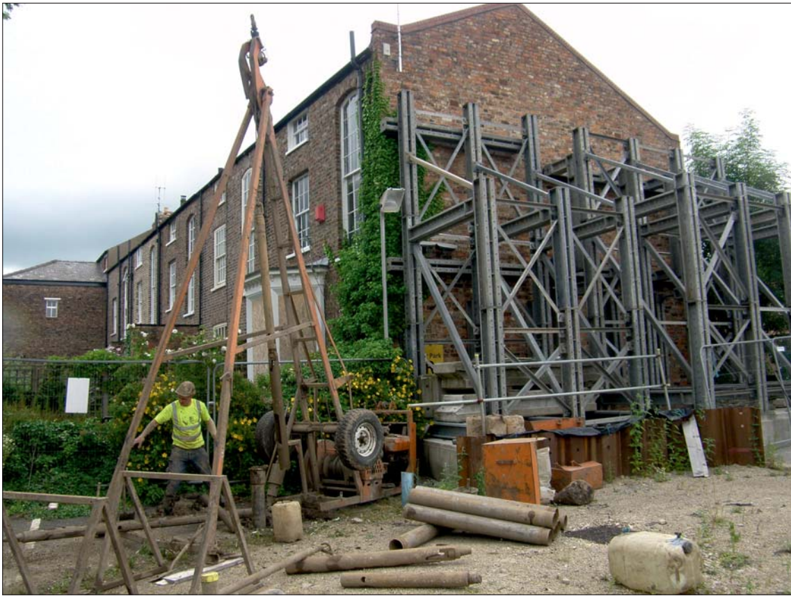
Union Terrace Geotechnical Investigation: location of starter pit for BH2
