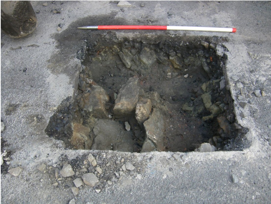
Plate 5. North Parade: pitched sandstone blocks used as road foundation
