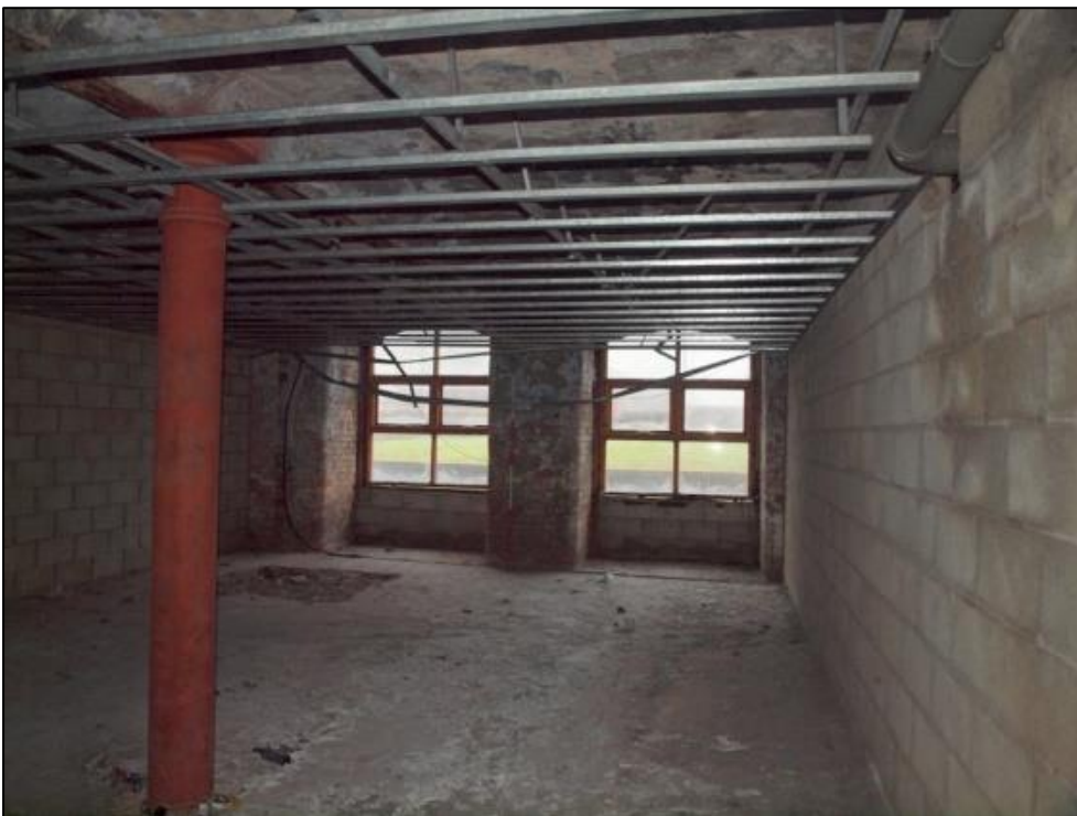
Plate 32: Northeast side of mill showing windows in north wall
