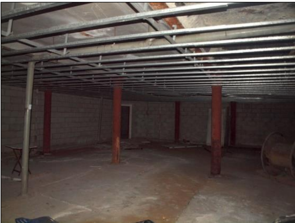
Plate 44: Southeast corner of mill looking northwest
