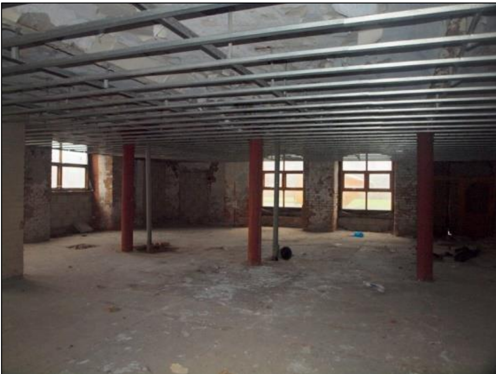
Plate 30: Northeast room of mill looking northwest
