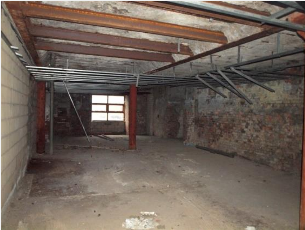
Plate 47: Northeast corner of Mill showing brick eastern wall
