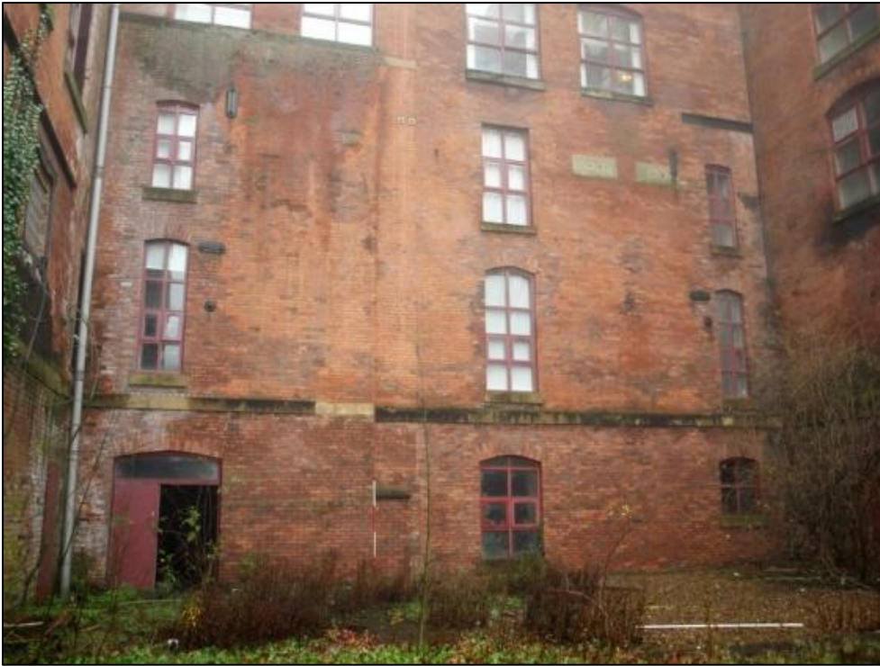
Plate 15: South facing courtyard wall
