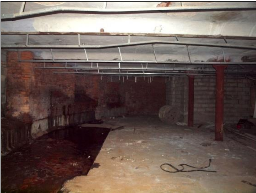
Plate 26: Southwest corner of mill showing angled wall with blocked windows
