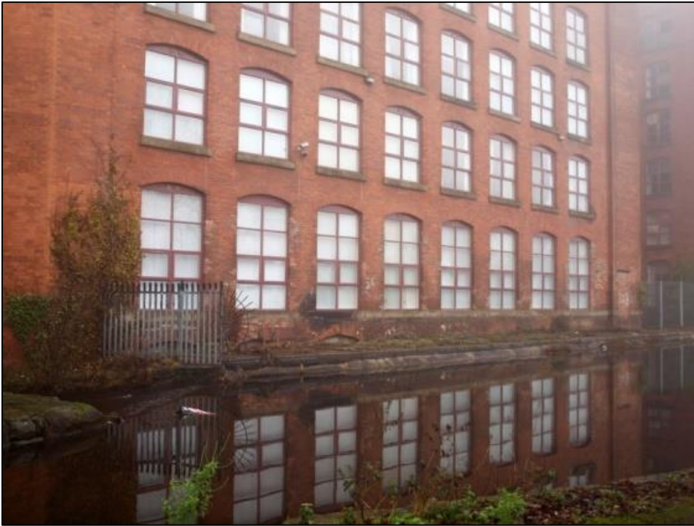
Plate 11: South elevation showing upper ground floor windows with arched lintels of lower ground floor blocked windows just visible
