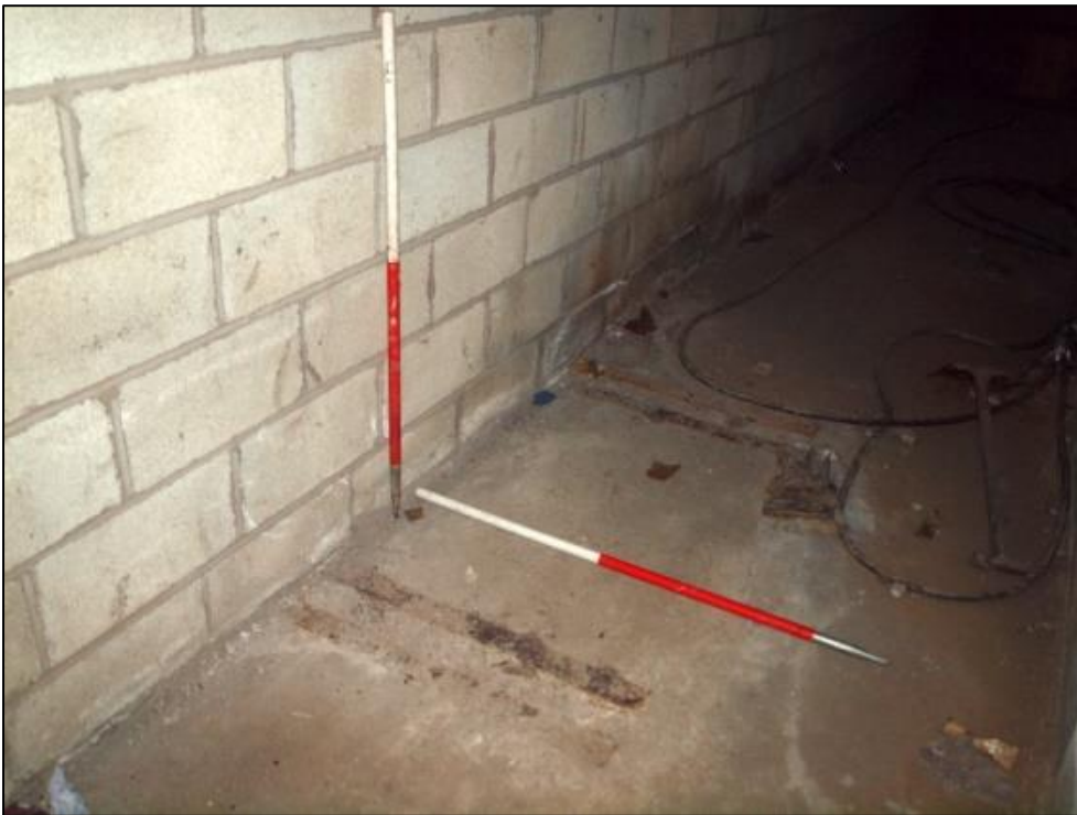
Plate 42: Rails as above as seen from other side of modern wall
