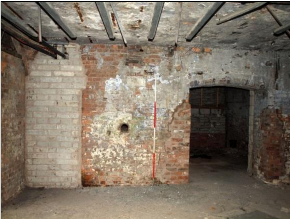
Plate 50: Northern end of east wall showing wide opening and blocked doorway to the north (left)
