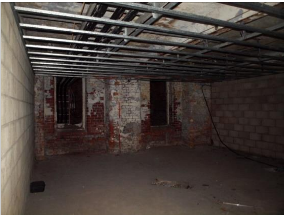
Plate 36: Northern wall of mill showing doorways leading through to small northern tower
