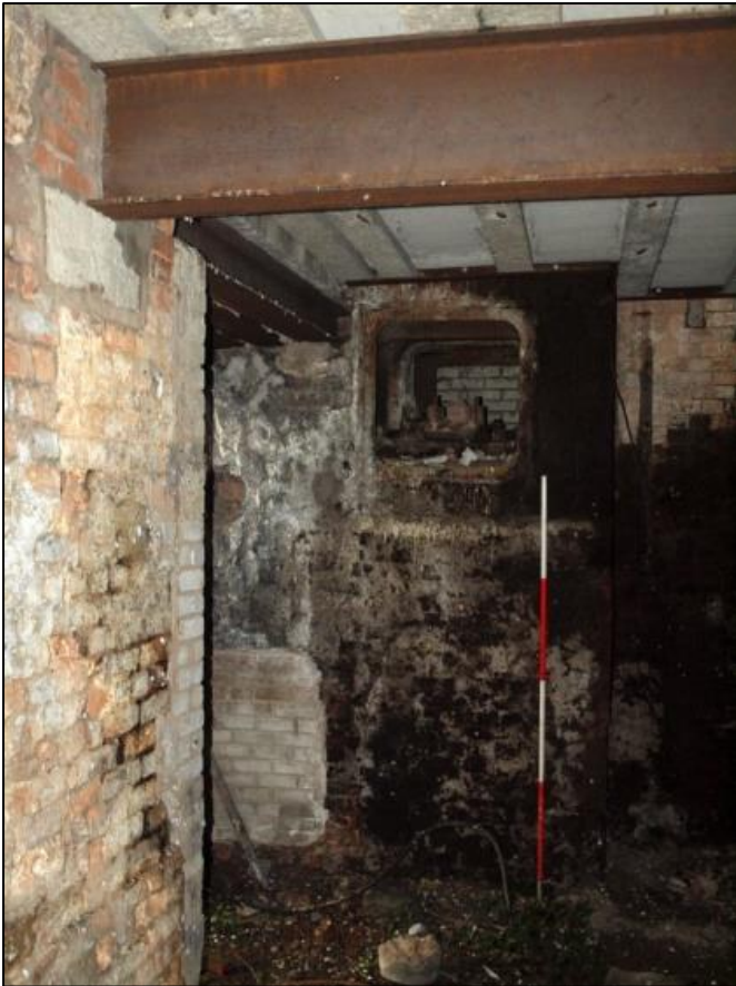
Plate 59: Detail of protruding transmission window
