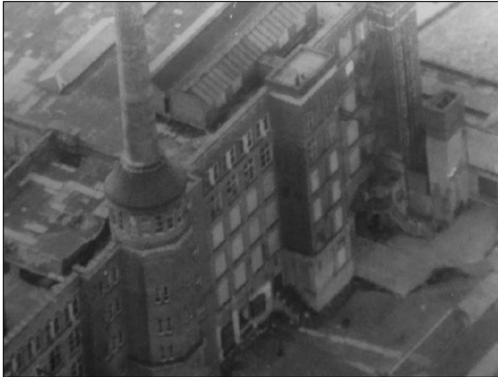
Figure 13: North elevation showing lower ground floor inserted windows, doorways and stair cases (Courtesy of GMAAS)
