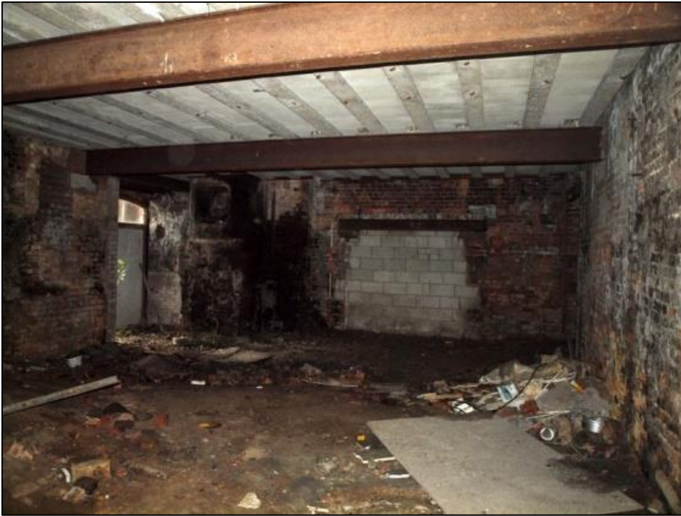
Plate 55: As above looking west
