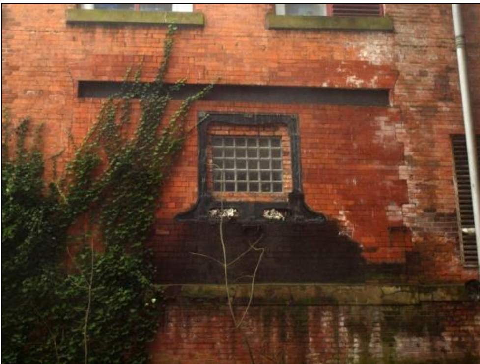
Plate 20: Detail of transmission window and surrounding rebuilding
