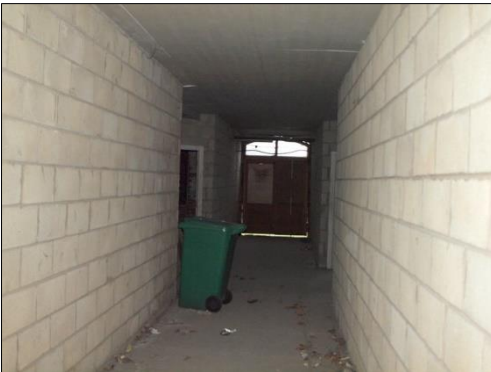
Plate 34: Corridor running to north end of mill
