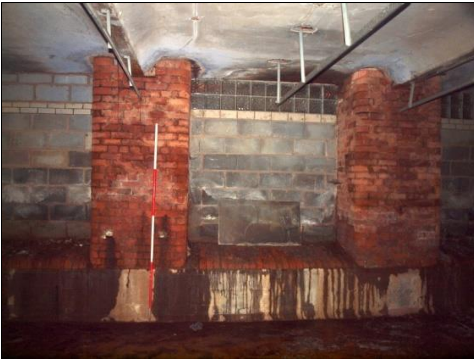
Plate 24: Southern wall of mill showing blocked windows
