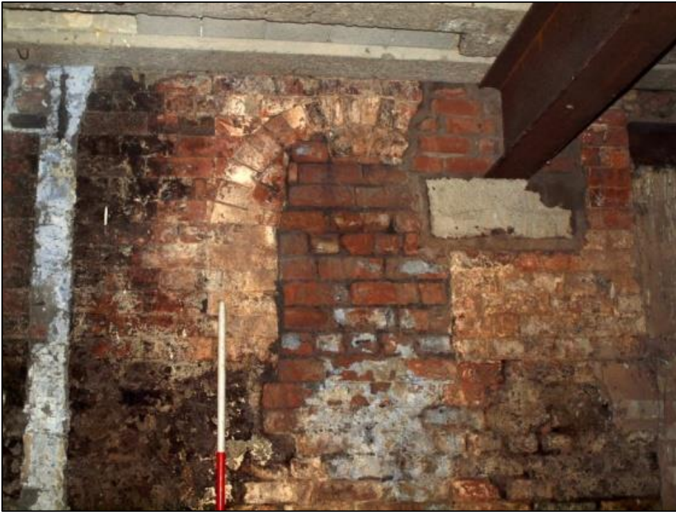
Plate 57: Blocked window with rounded arch high in southern wall
