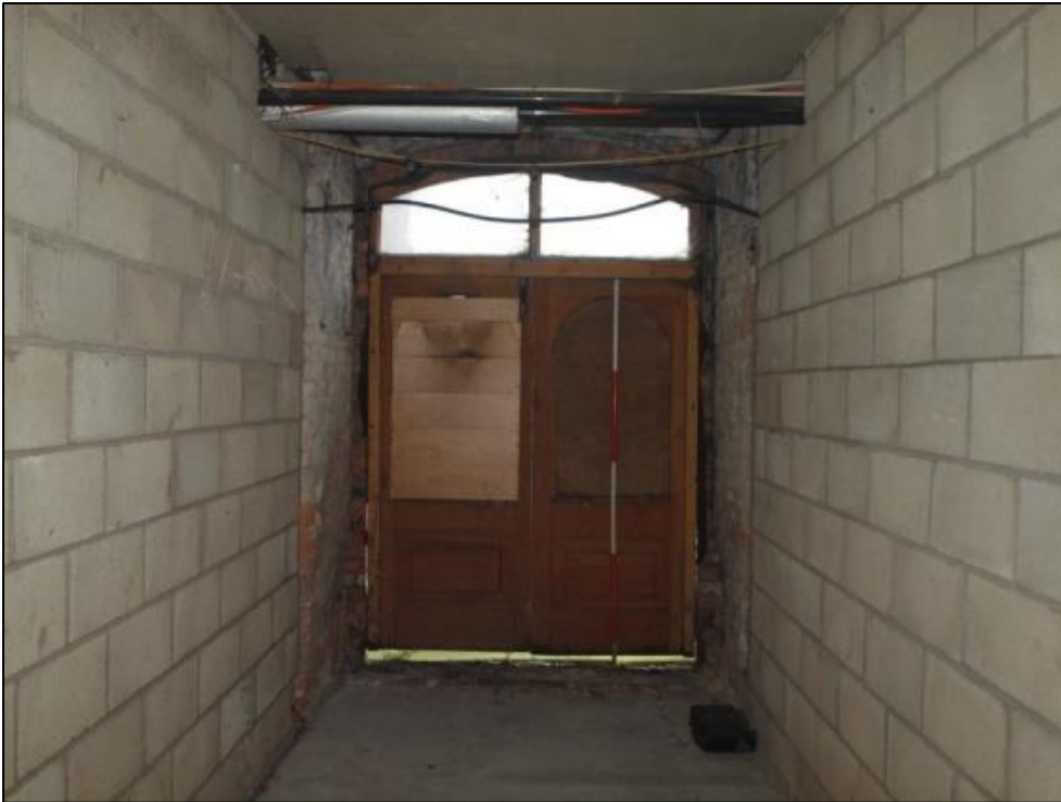
Plate 35: Detail of doorway in bay 5 of north wall
