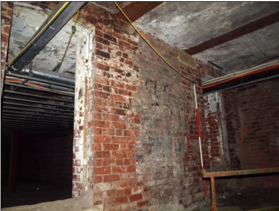
Plate 38: As above looking south, showing inserted doorways into blocked windows
