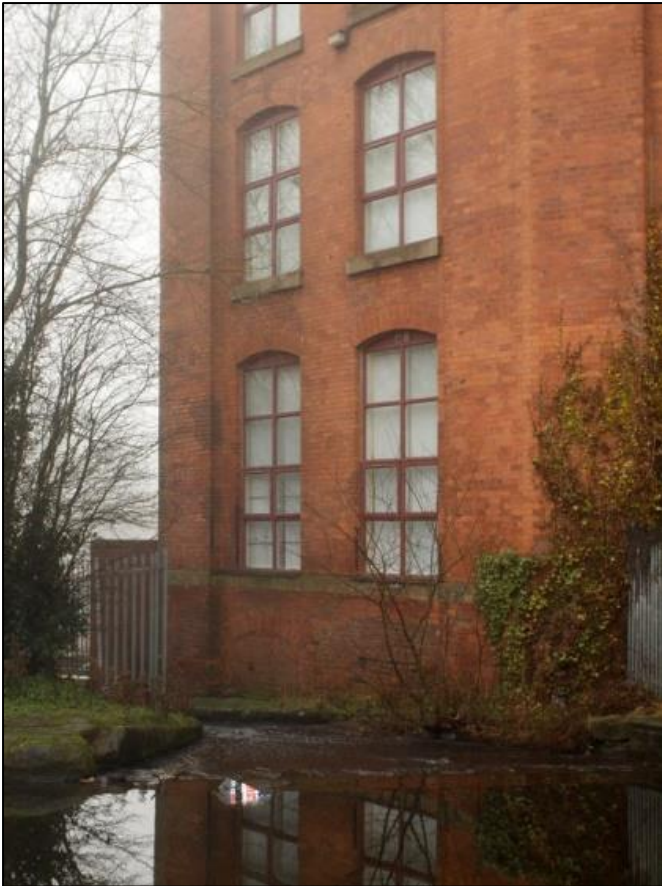
Plate 13: Angled southwest corner of mill
