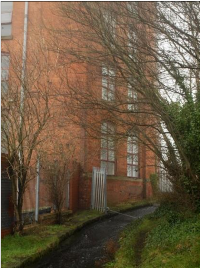
Plate 12: Angled southwest corner of mill
