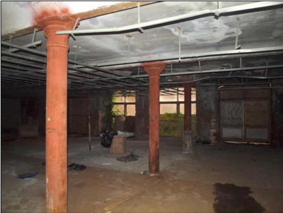
Plate 43: Southeast side of mill showing windows and doorways to courtyard
