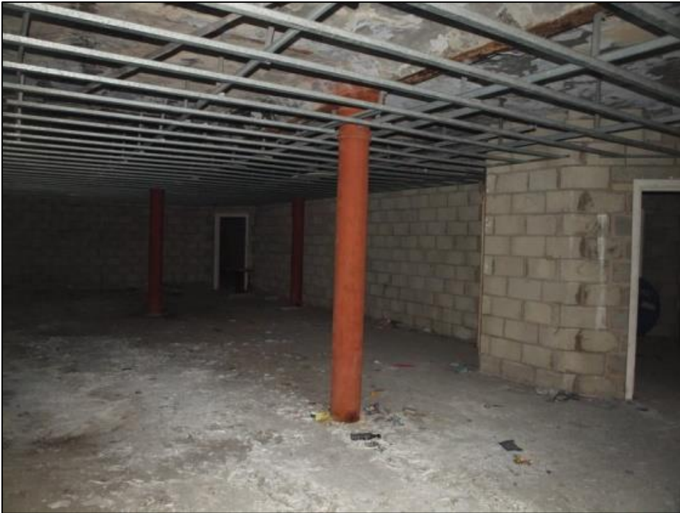
Plate 33: Northeast side of mill looking south
