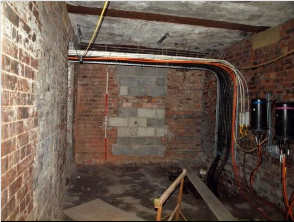
Plate 39: West wall of northern projection showing blocked doorway
