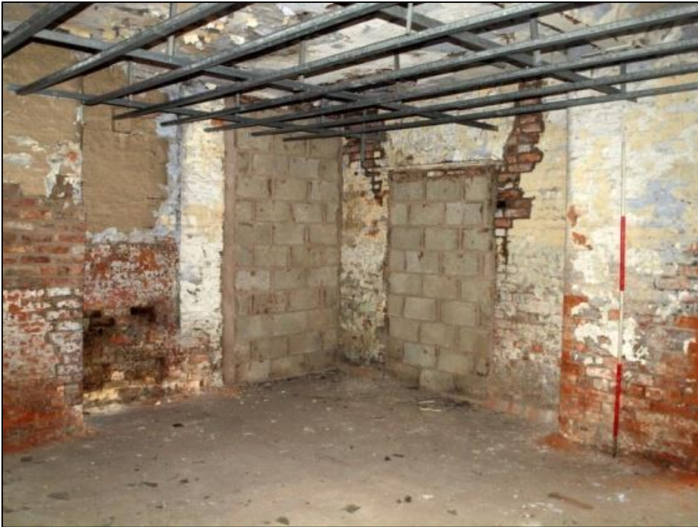
Plate 31: Northwest corner of mill showing blocked doorways
