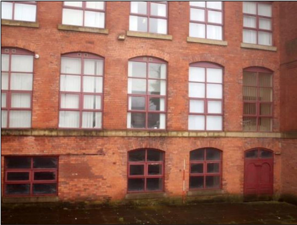
Plate 5: Eastern end of north elevation
