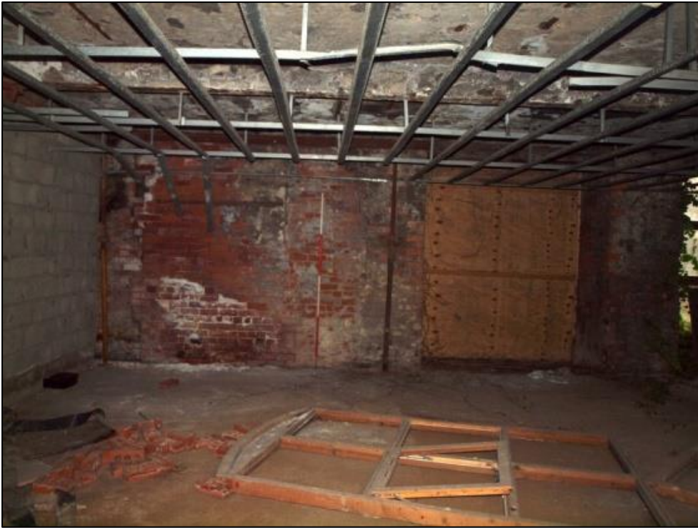
Plate 45: Blocked doorway in east wall
