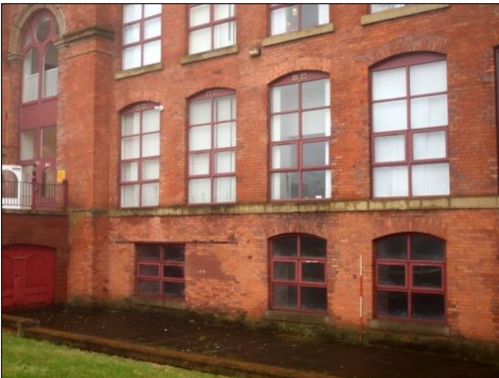
Plate 4: Eastern end of north elevation
