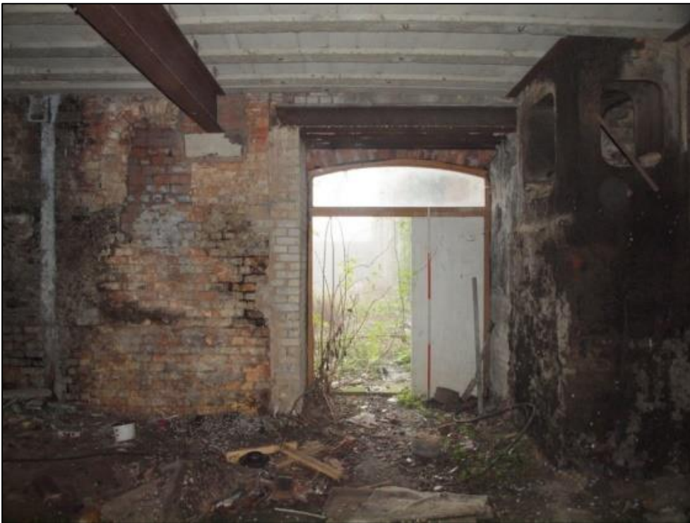
Plate 56: Inserted doorway at western end of southern wall and both windows of the protruding transmission window (right)
