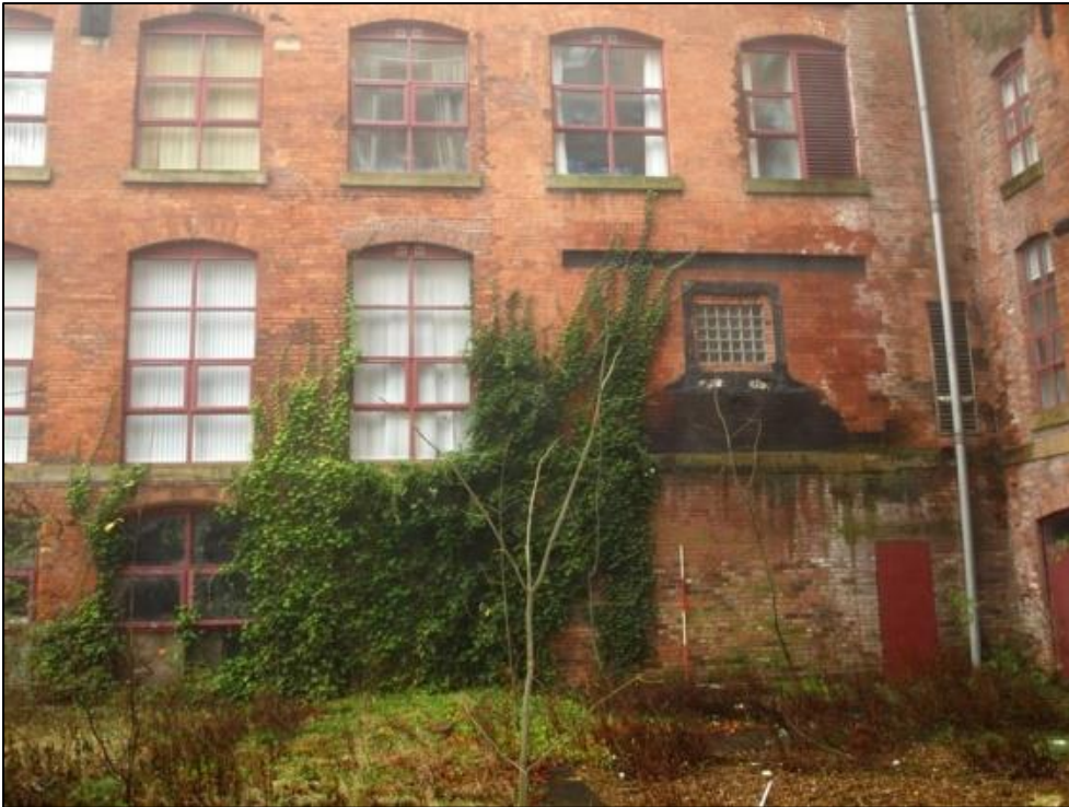
Plate 19: Northern end of east facing courtyard wall
