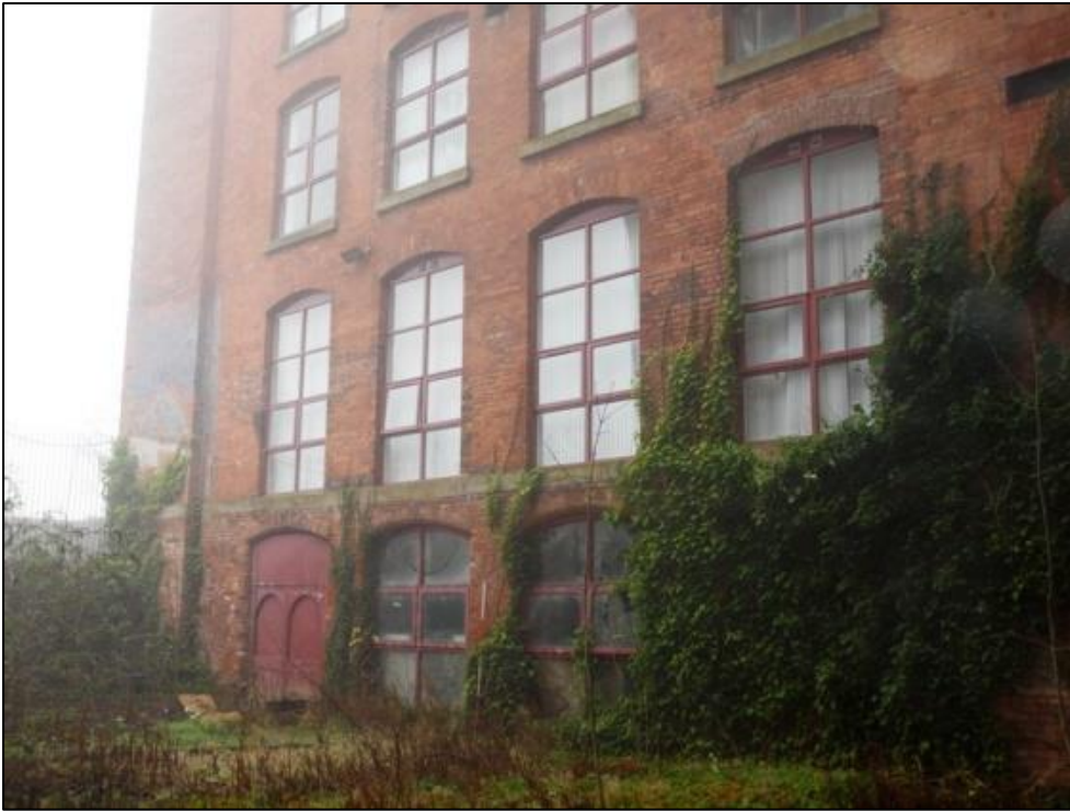
Plate 21: Southern end of east facing courtyard wall
