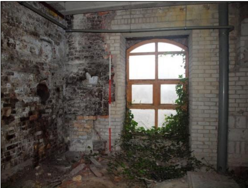
Plate 58: Detail of east end of south wall showing extensive rebuilding and sandstone block with fixing holes
