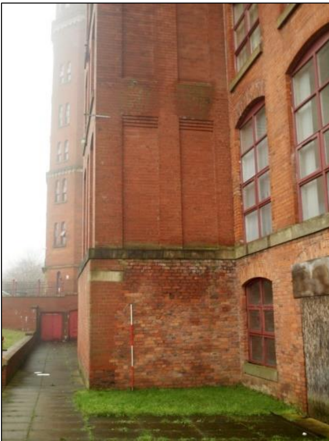
Plate 8: West elevation of shaft
