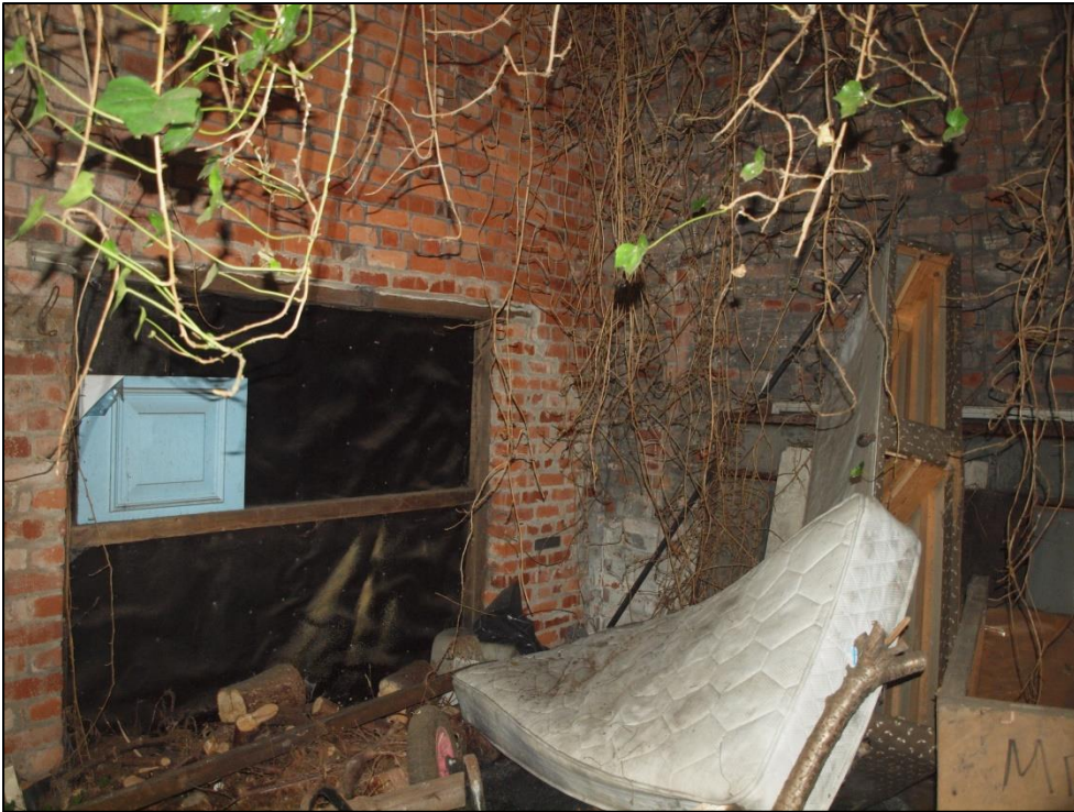
Plate 33: Inserted wall and opening in northern end of bay 3
