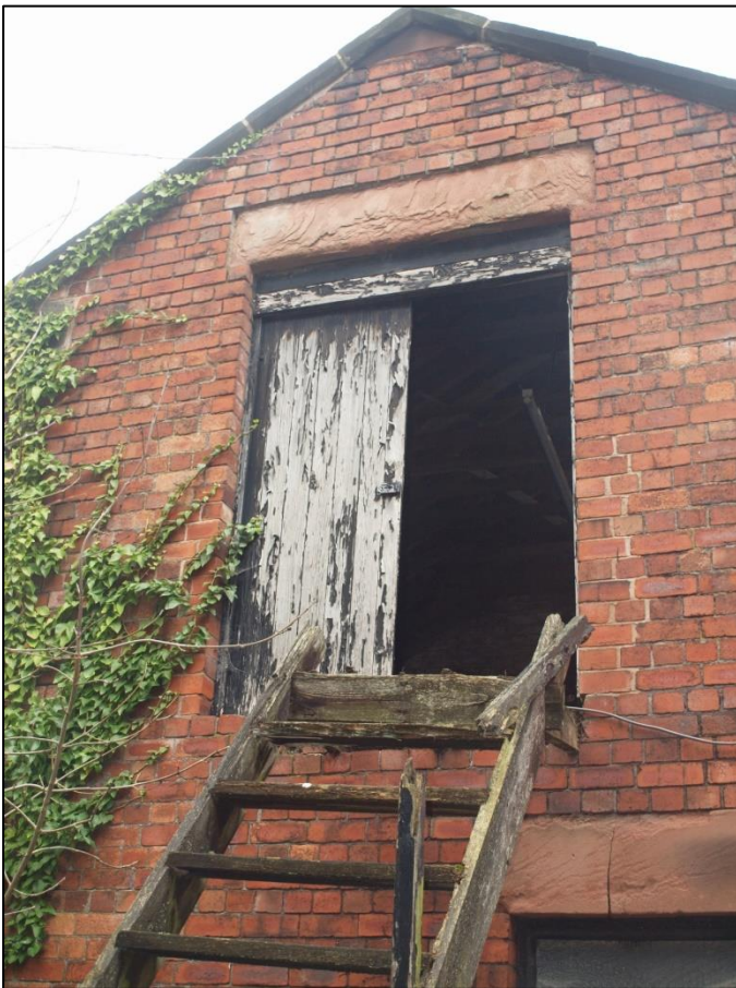
Plate 14: Detail of first floor doorway
