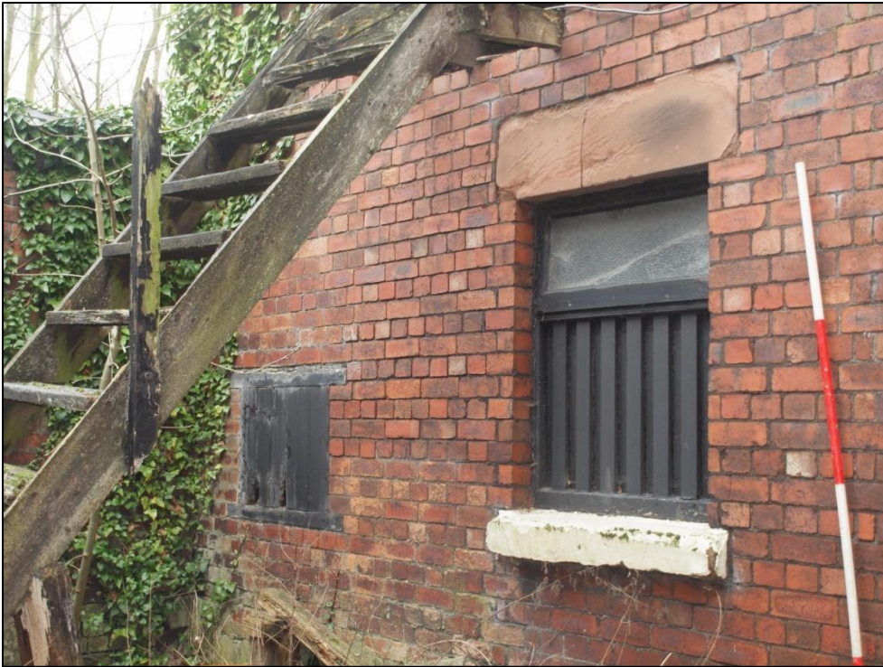
Plate 13: Detail of ground floor windows
