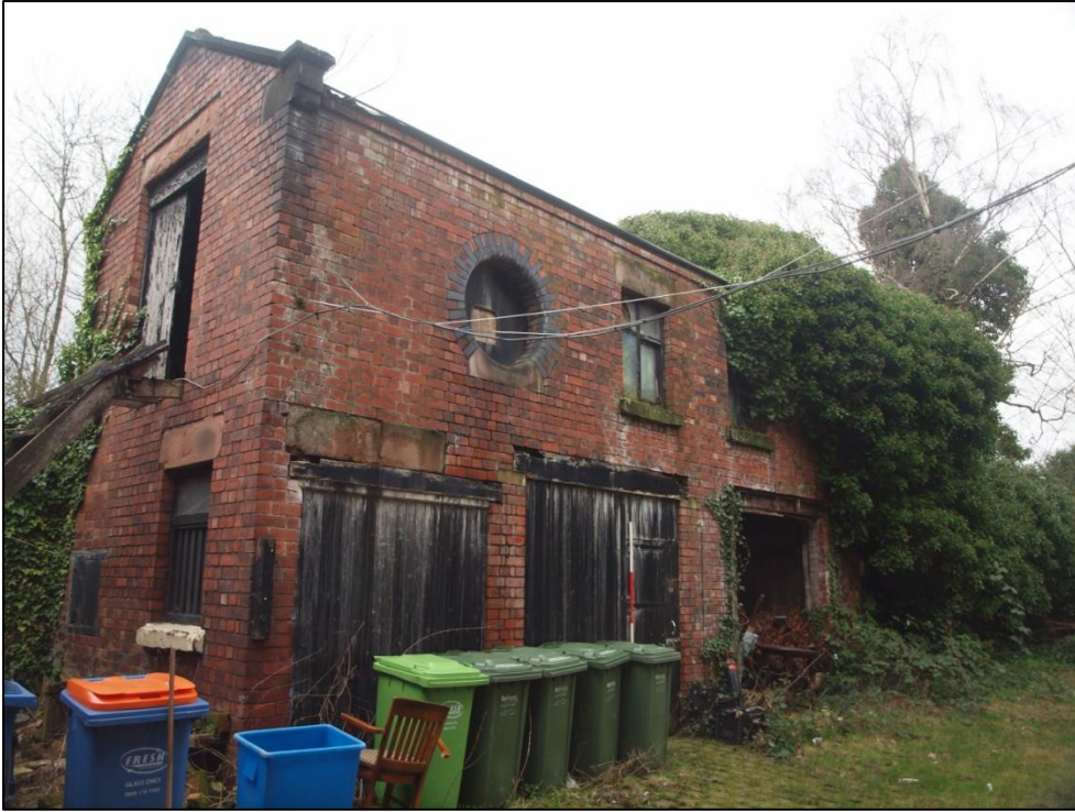
Plate 5: Bay 1 of east elevation
