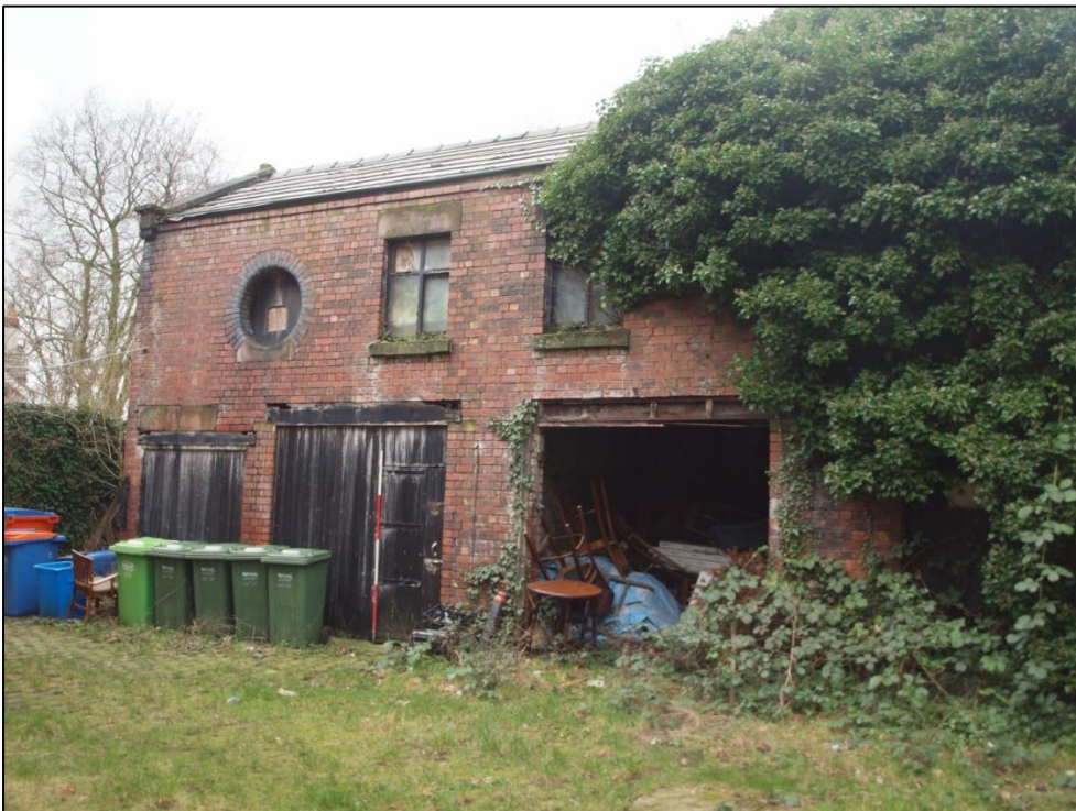
Plate 4: General shot of east elevation
