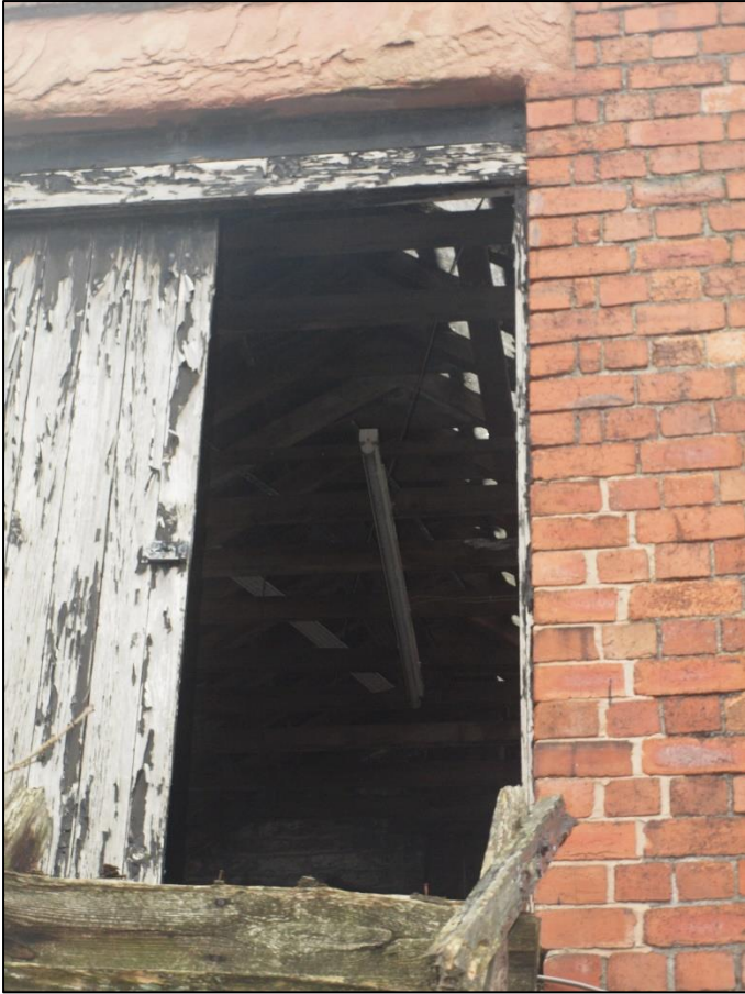
Plate 35: View into first floor showing roof trusses.
