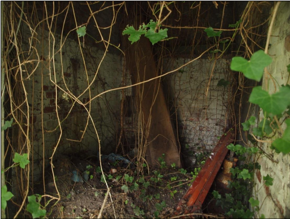
Plate 29: Southern end of bay 3
