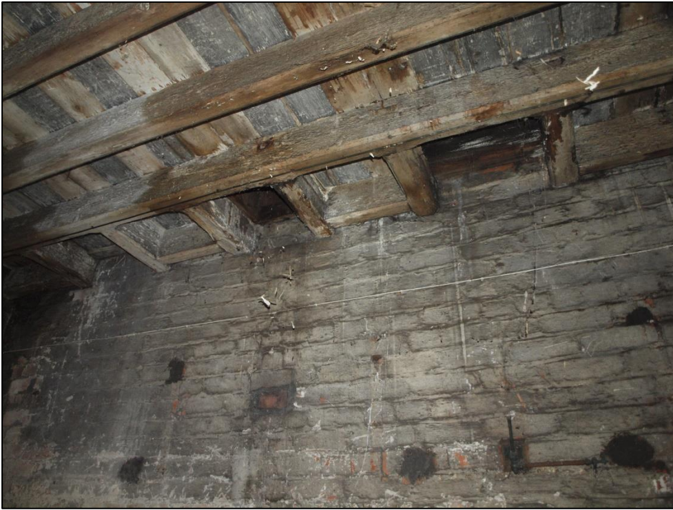
Plate 25: Detail of hatches in bay 1 ceiling
