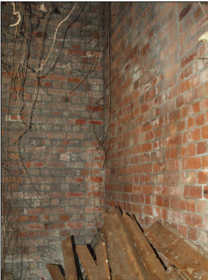
Plate 34: Different brick between west wall (left) and redder brick of north wall (right) in bay 3
