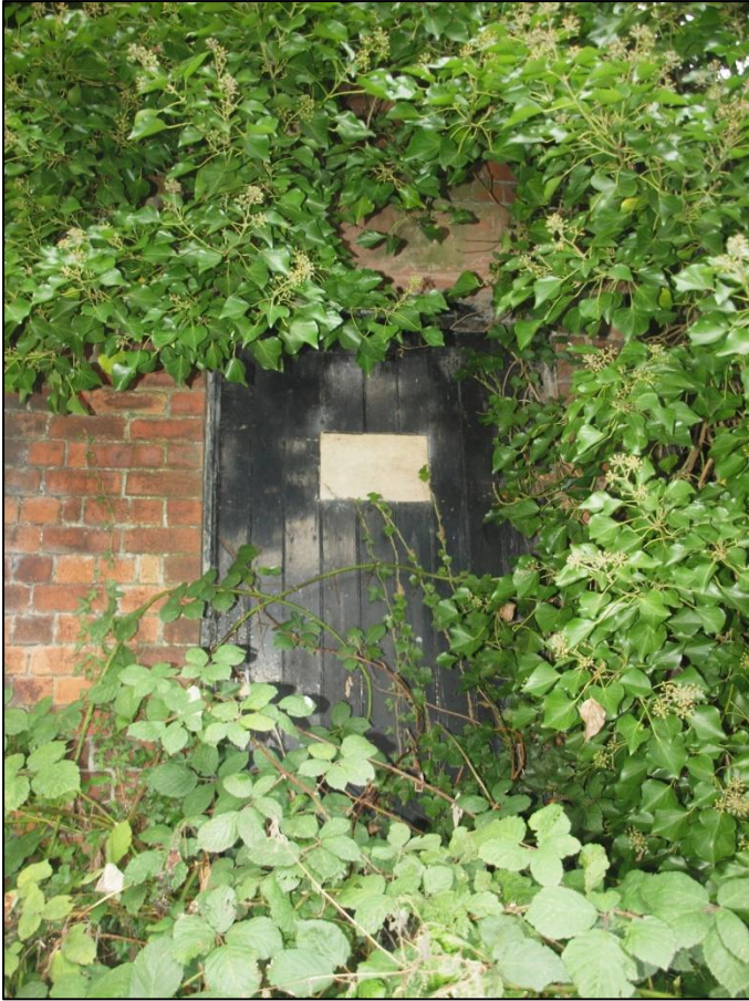
Plate 9: Personnel door to bay 2
