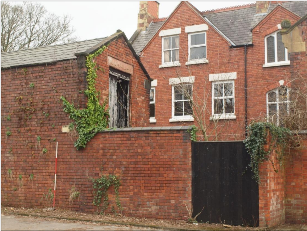
Plate 17: Wall of west elevation continues south with gate to yard
