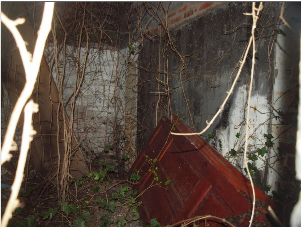
Plate 30: Southern end of bay 3
