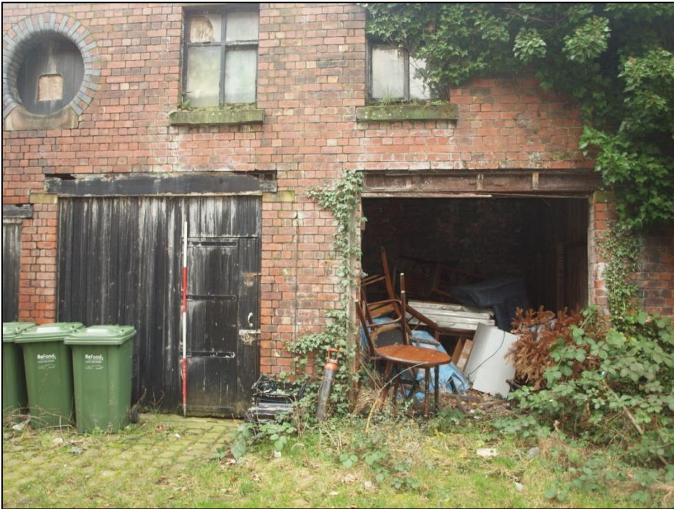
Plate 6: Detail of inserted loading doors at south end of east elevation
