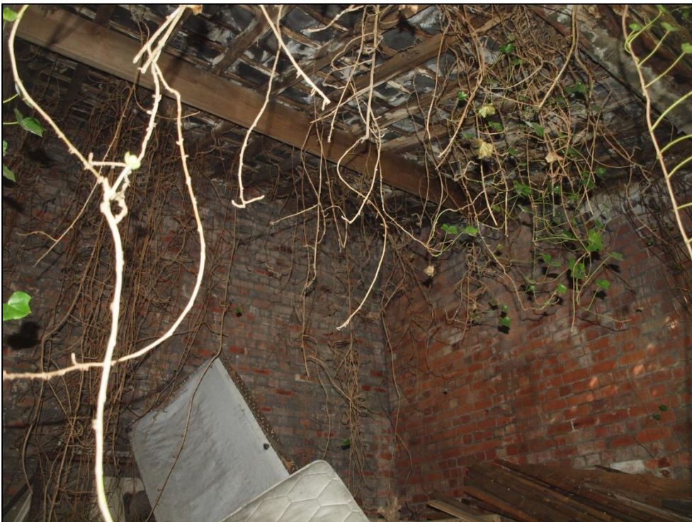
Plate 32: Detail of roof of northern end of bay 3
