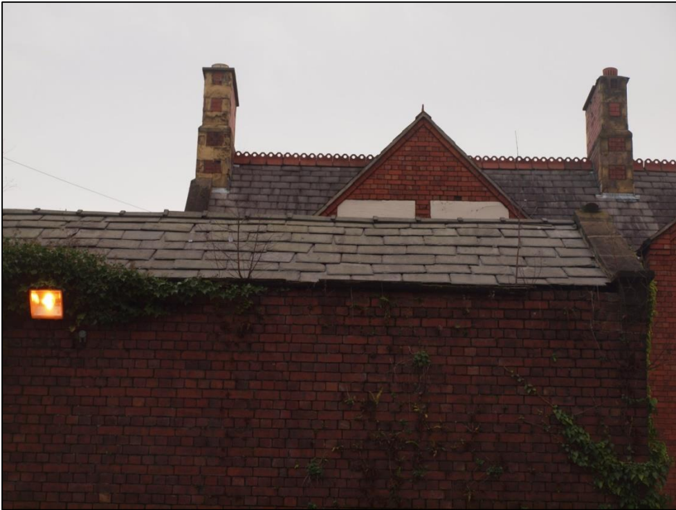
Plate 3: Detail of slate roof
