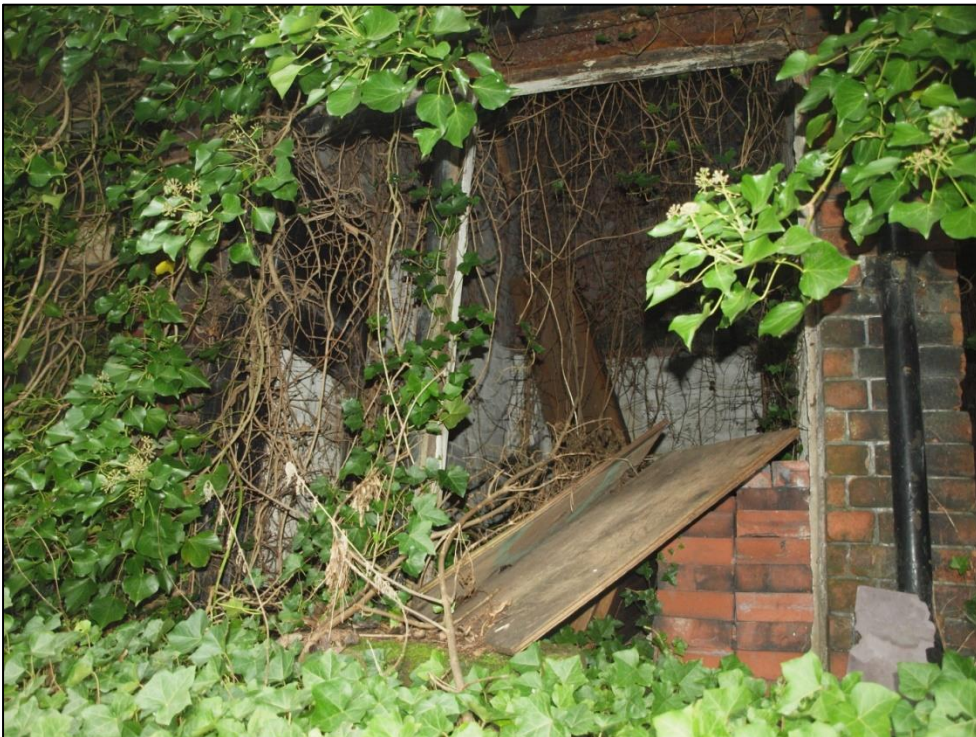
Plate 10: Southern loading door to bay 3
