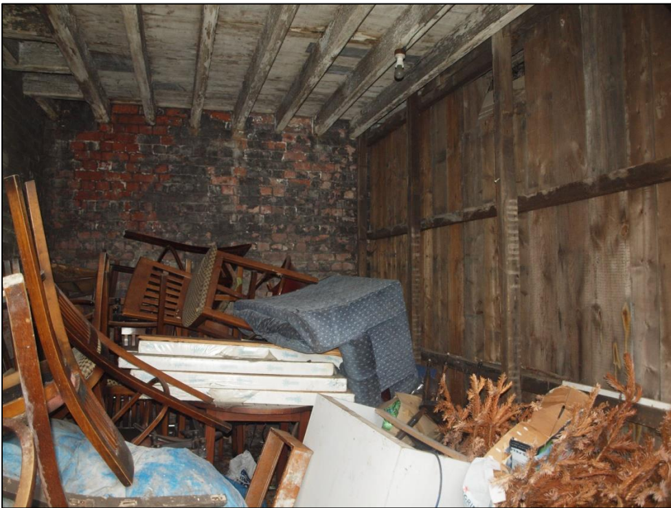
Plate 26: Bay 2, southern end showing inserted timber wall
