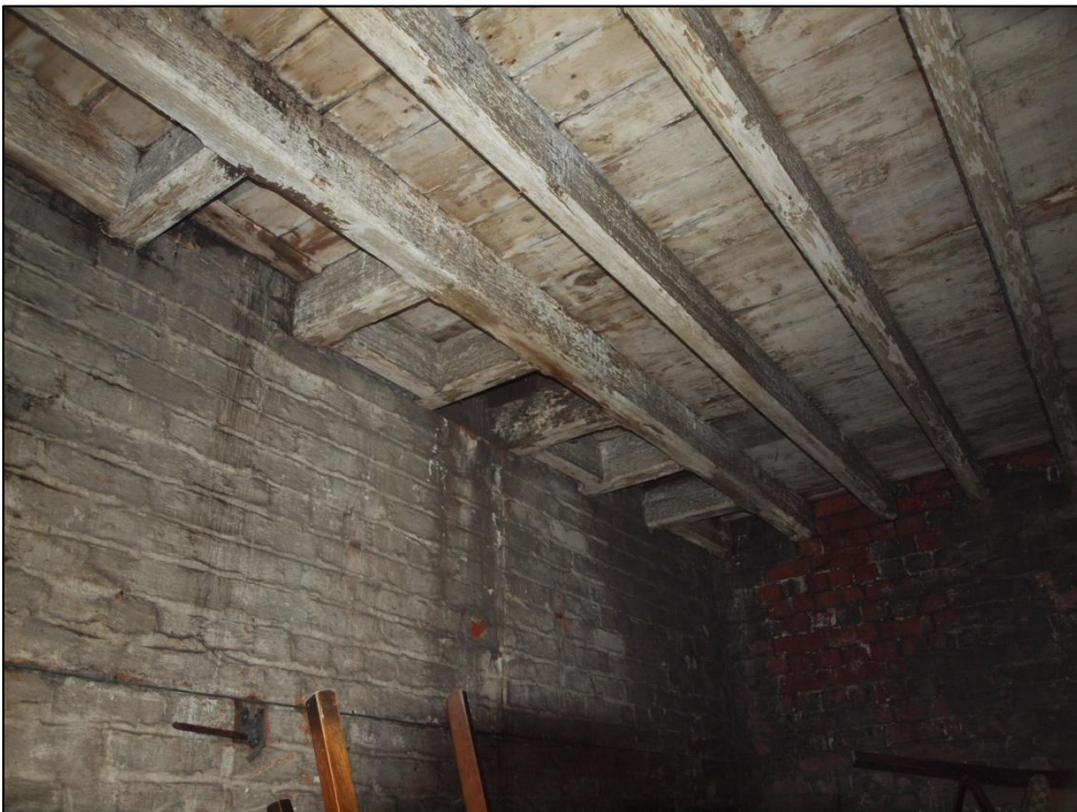
Plate 28: Detail of hatches in ceiling of bay 2
