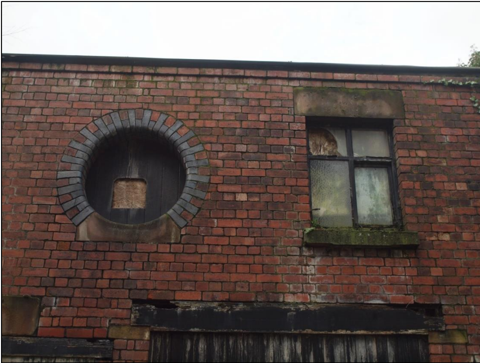
Plate 7: Detail of first floor windows
