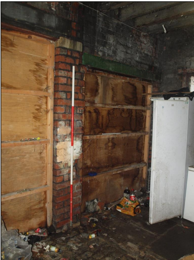
Plate 24: Detail of doorways
