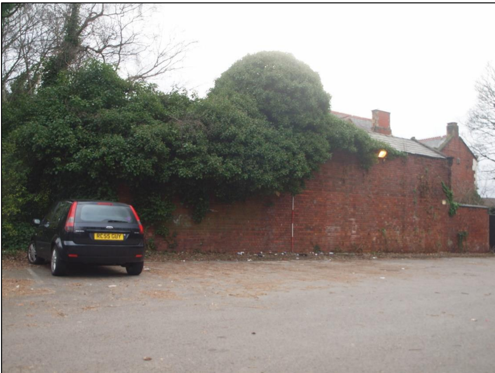
Plate 16: West elevation showing overgrown north end
