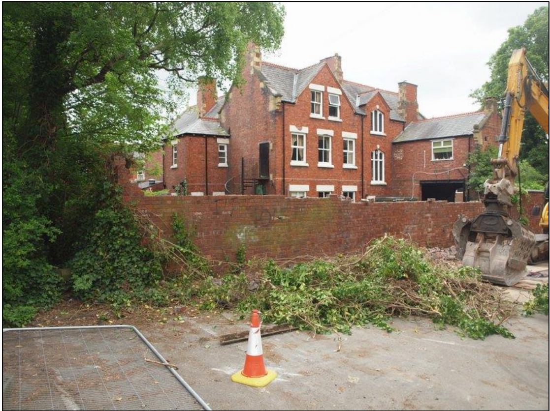
Plate 13: Building after partial demolition
