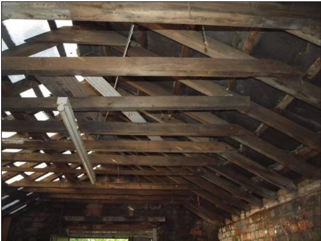
Plate 6: Detail of modern roof trusses
