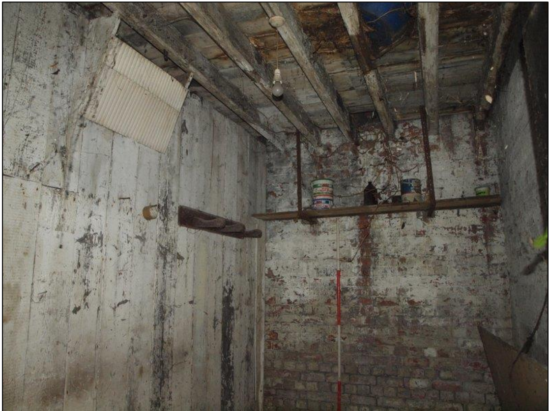
Plate 2: As above showing ceiling joists
