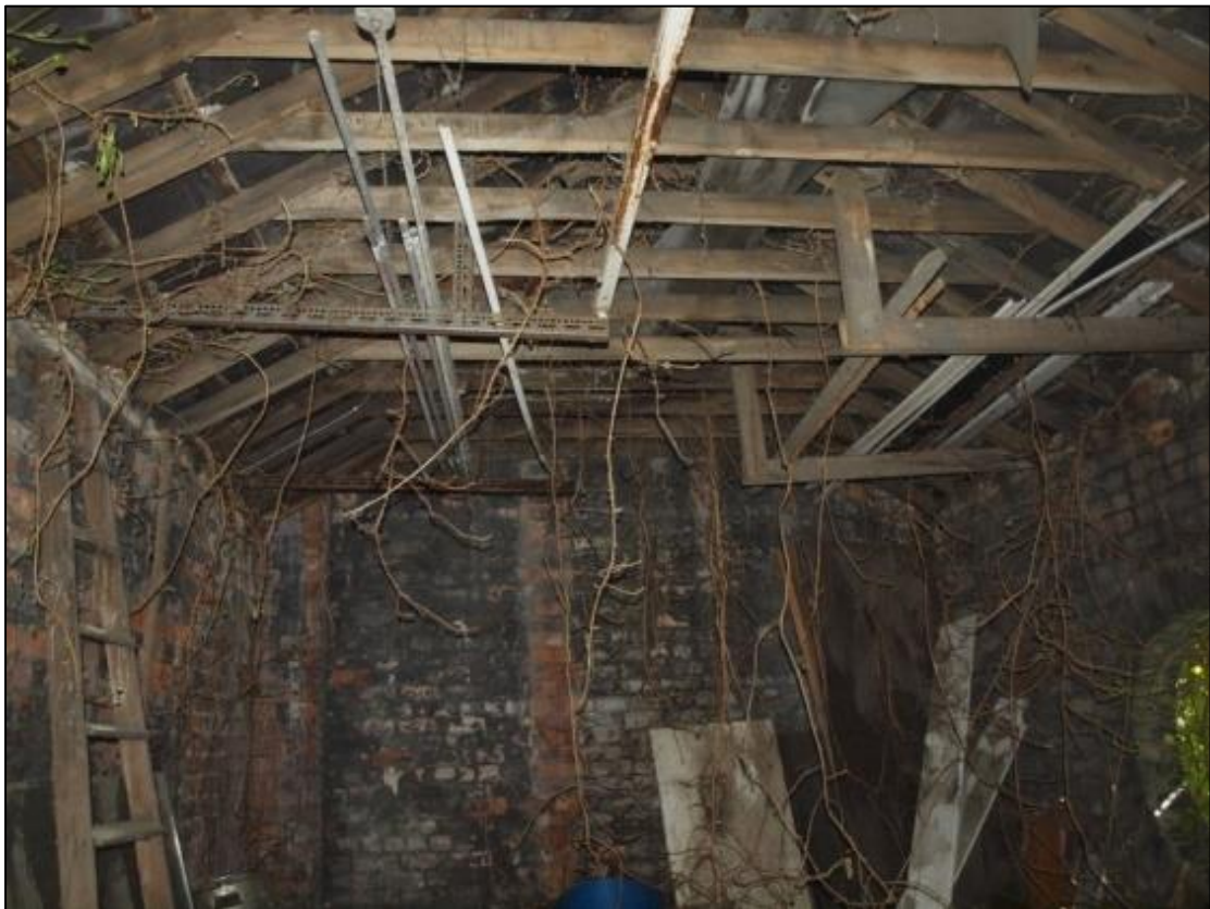
Plate 10: Roof trusses of north room
