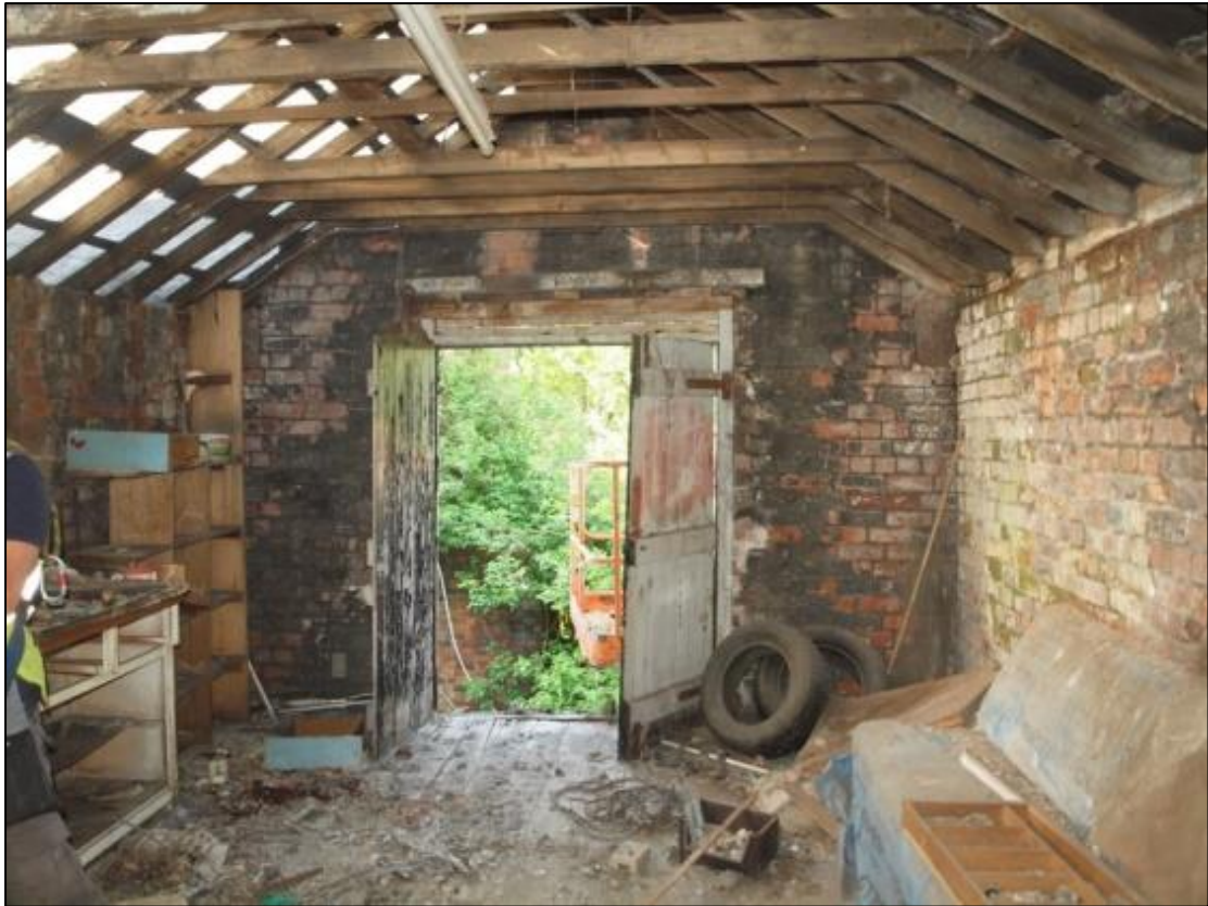
Plate 5: Southern room of first floor looking south
