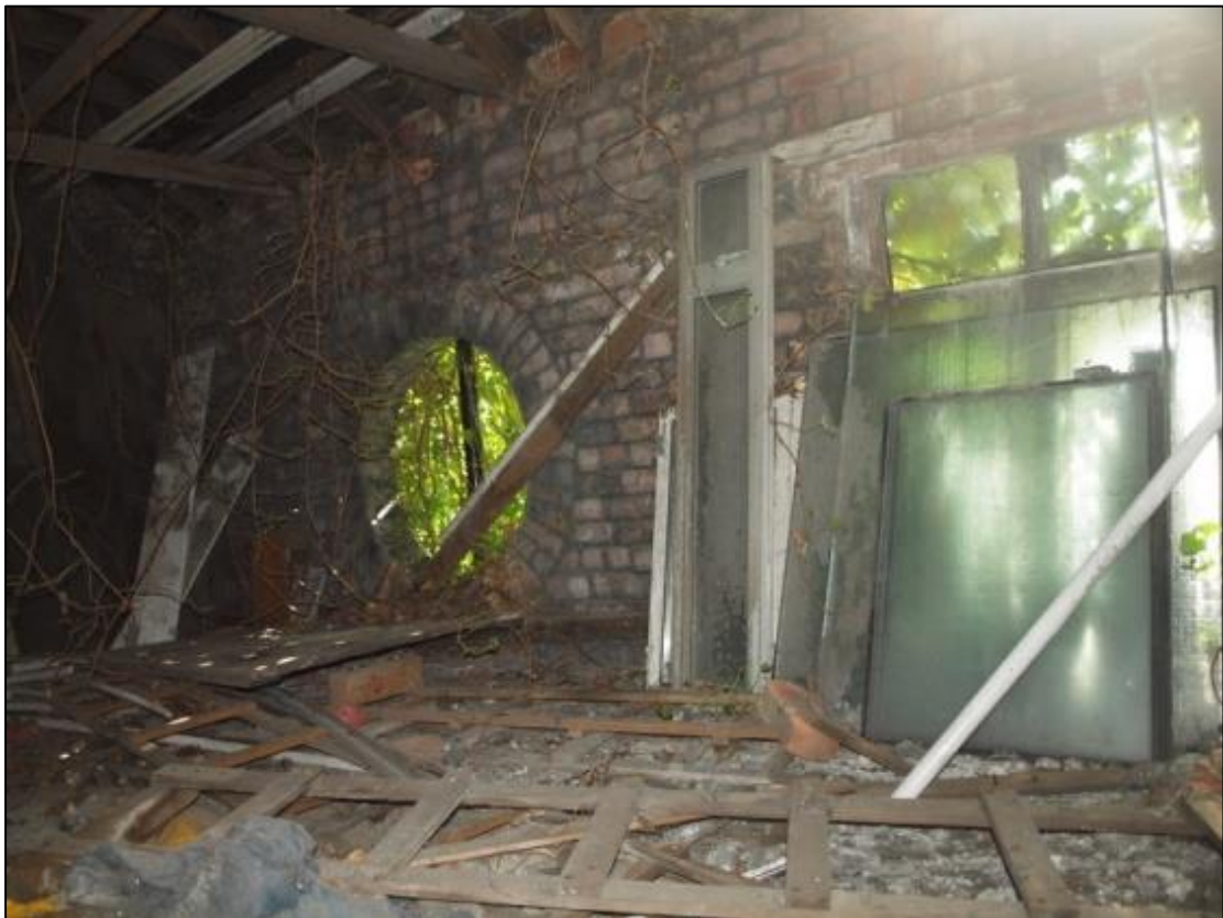
Plate 8: North room of first floor
