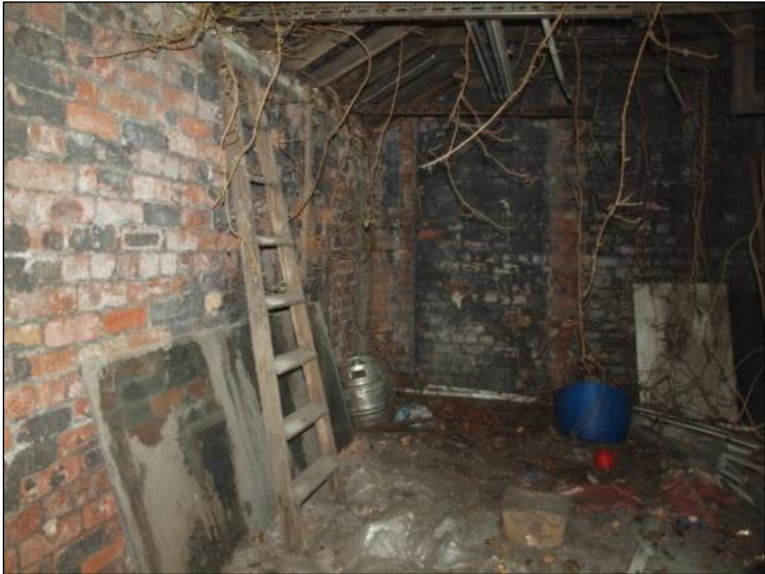
Plate 11: Blocked opening in north wall of north room
