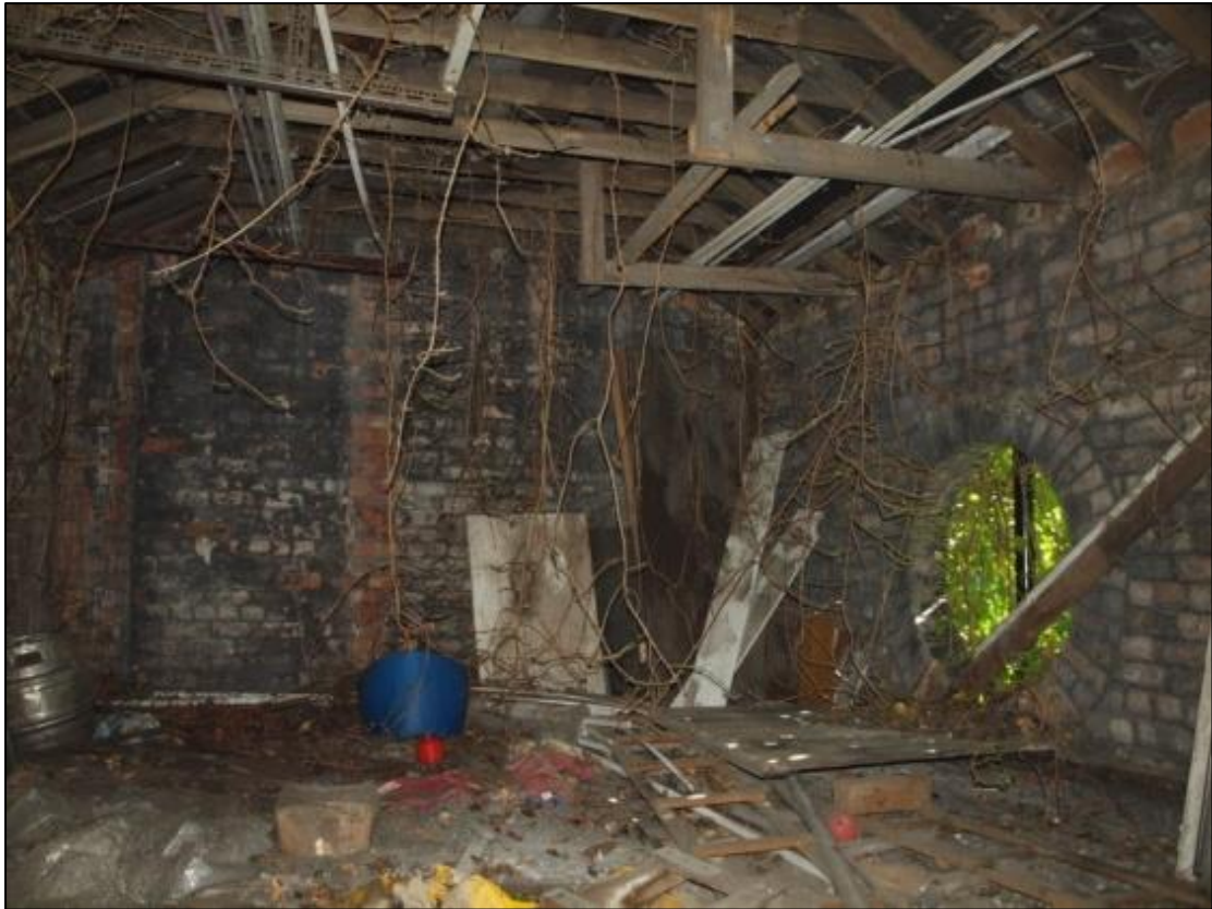
Plate 9: North room of first floor
