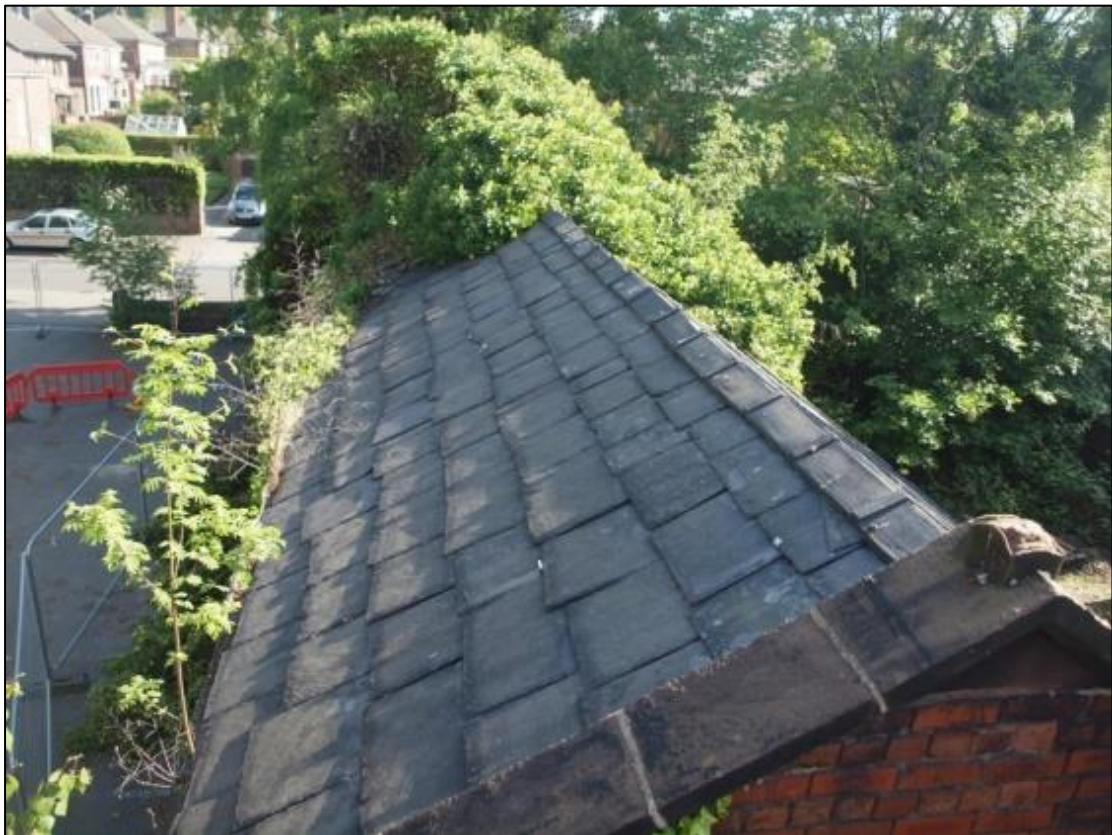
Plate 12: Detail of slate roof
