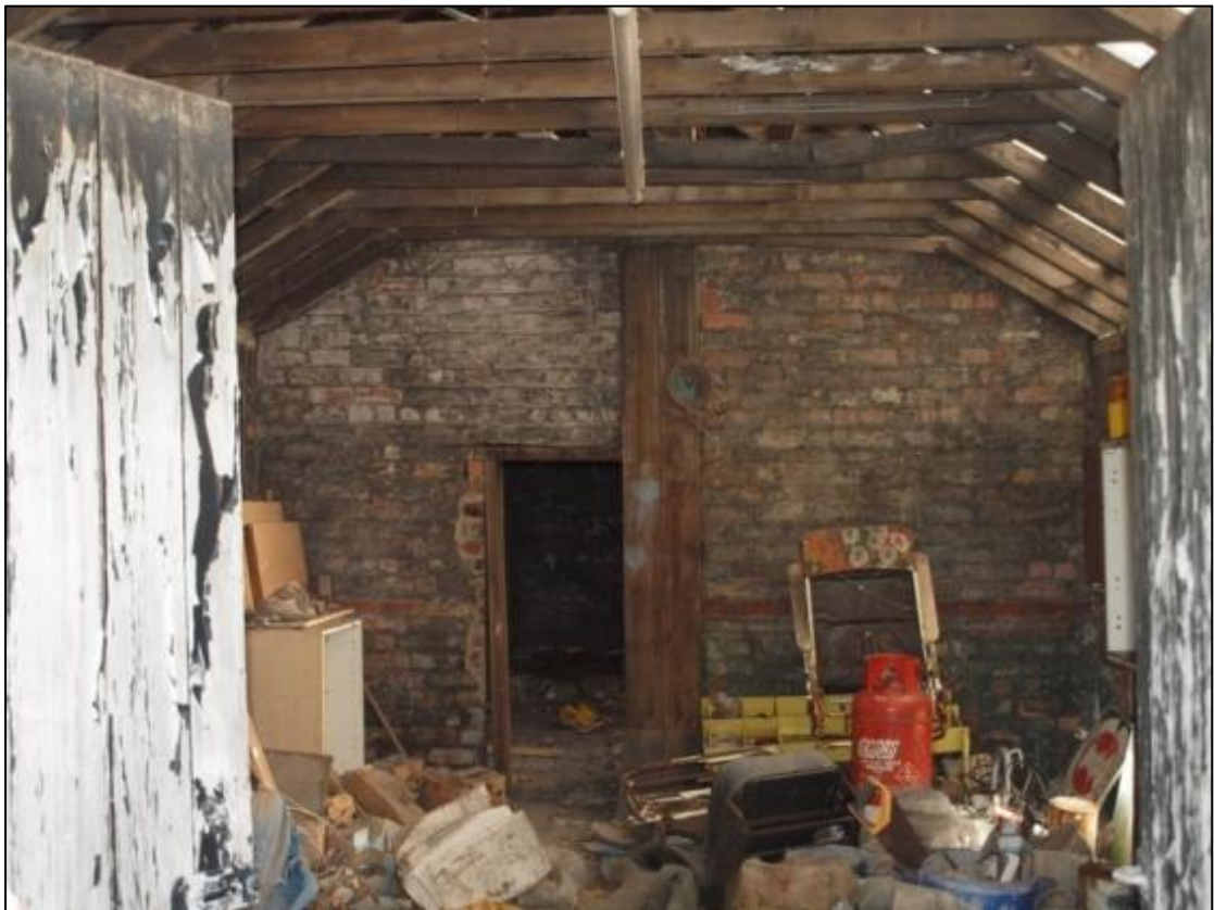
Plate 4: Southern room of first floor
