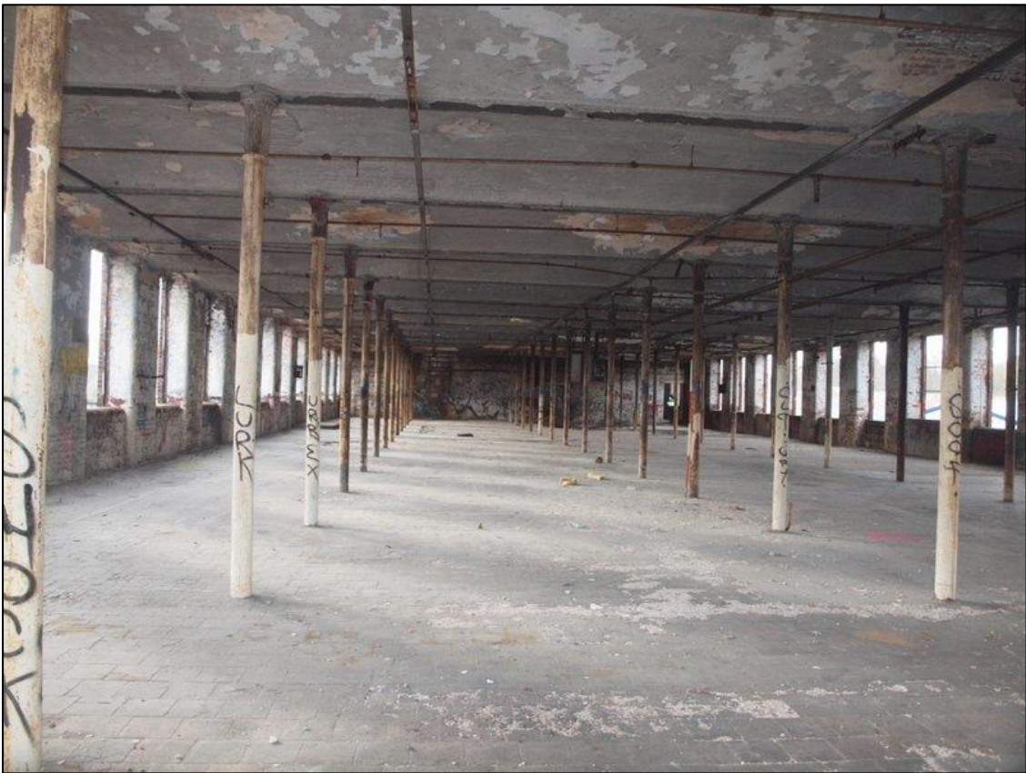
Plate 66: General shot of first floor of mill
