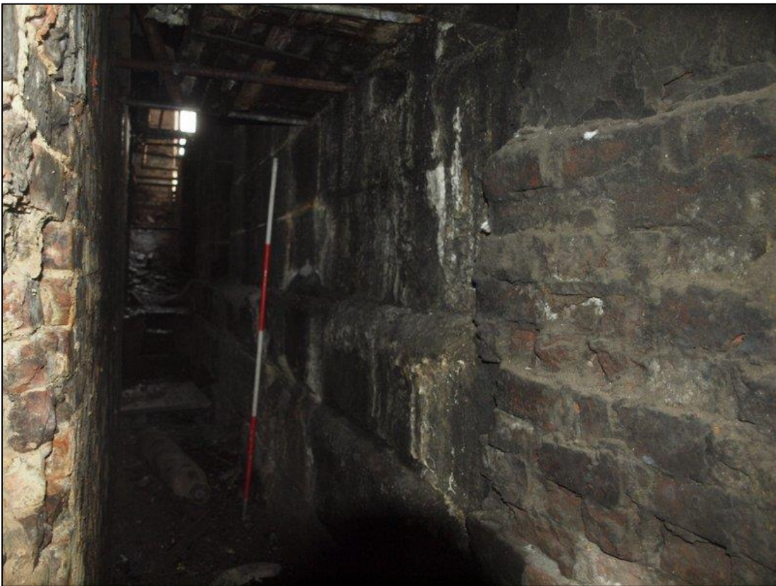
Plate 56: View down passageway between party wall (left) and stone engine base (right)
