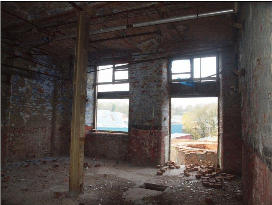
Plate 64: Inserted doorway to northwest elevation
