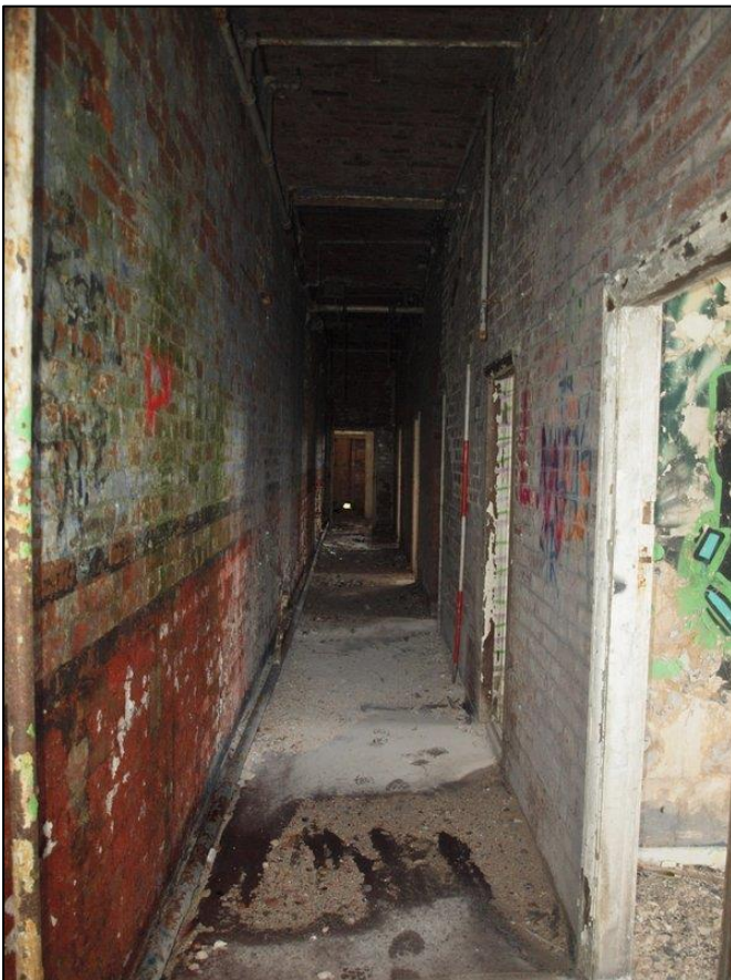
Plate 84: Inserted corridor along first floor of boiler house
