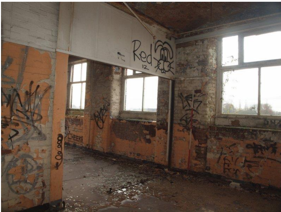
Plate 88: Inserted room in boiler house
