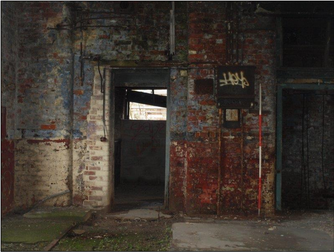
Plate 69: Detail of stair tower doorway
