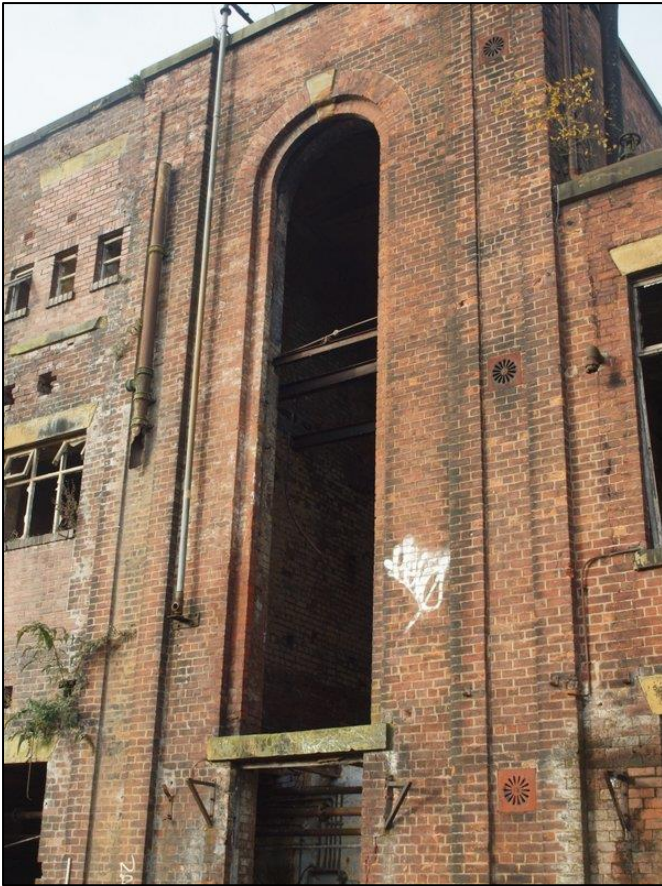
Plate 27: First floor of engine house showing two story window
