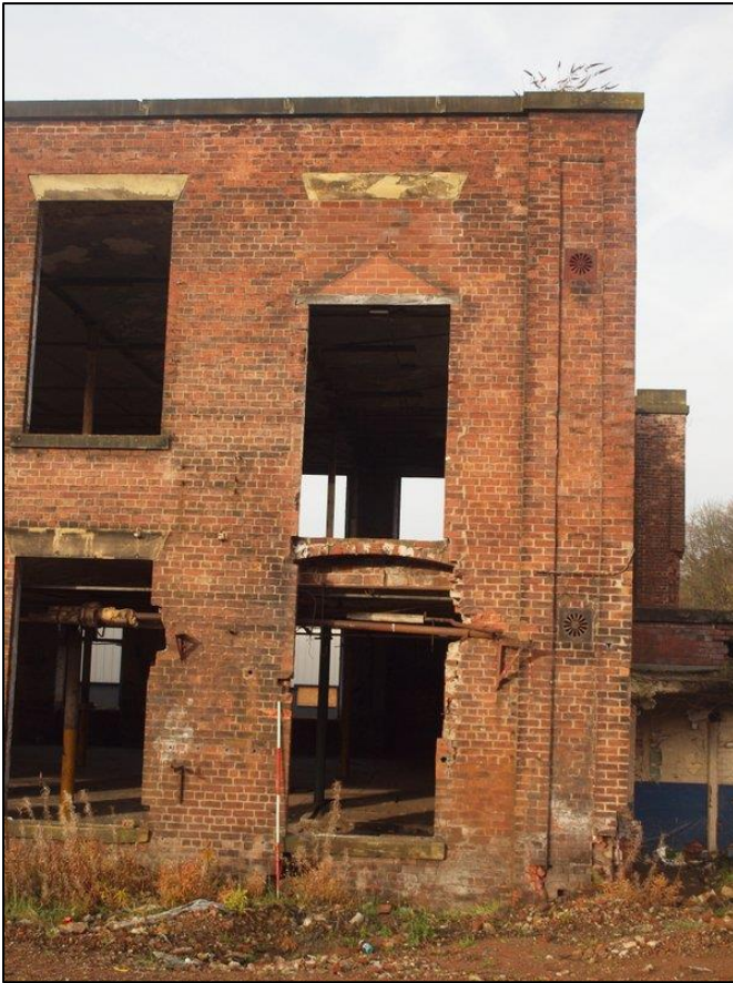
Plate 31: Southwest elevation bay 15 detail showing inserted first floor doorway Northeast elevation
