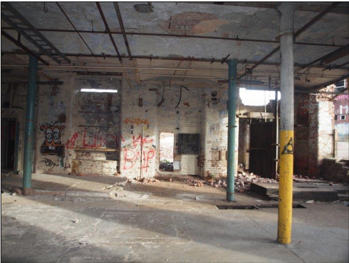
Plate 42: Eastern end of northeast wall showing inserted doorways
