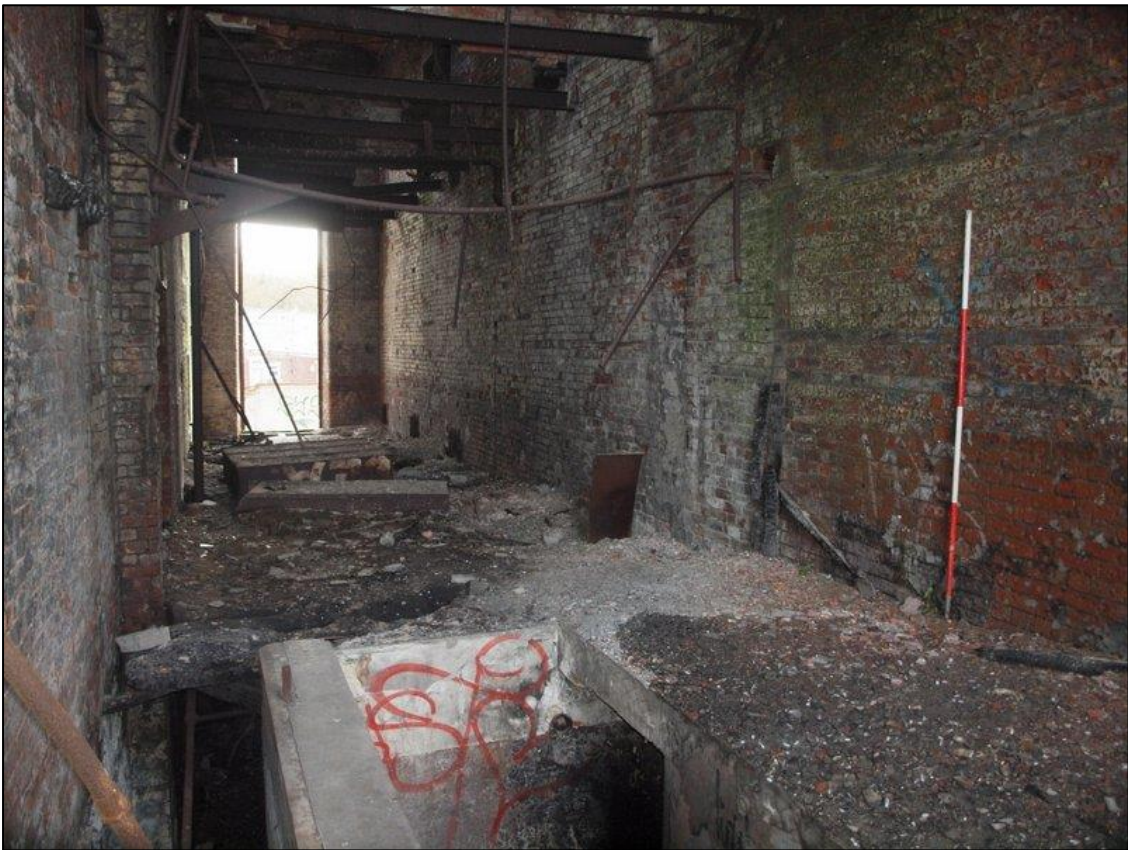
Plate 80: General shot of engine house
