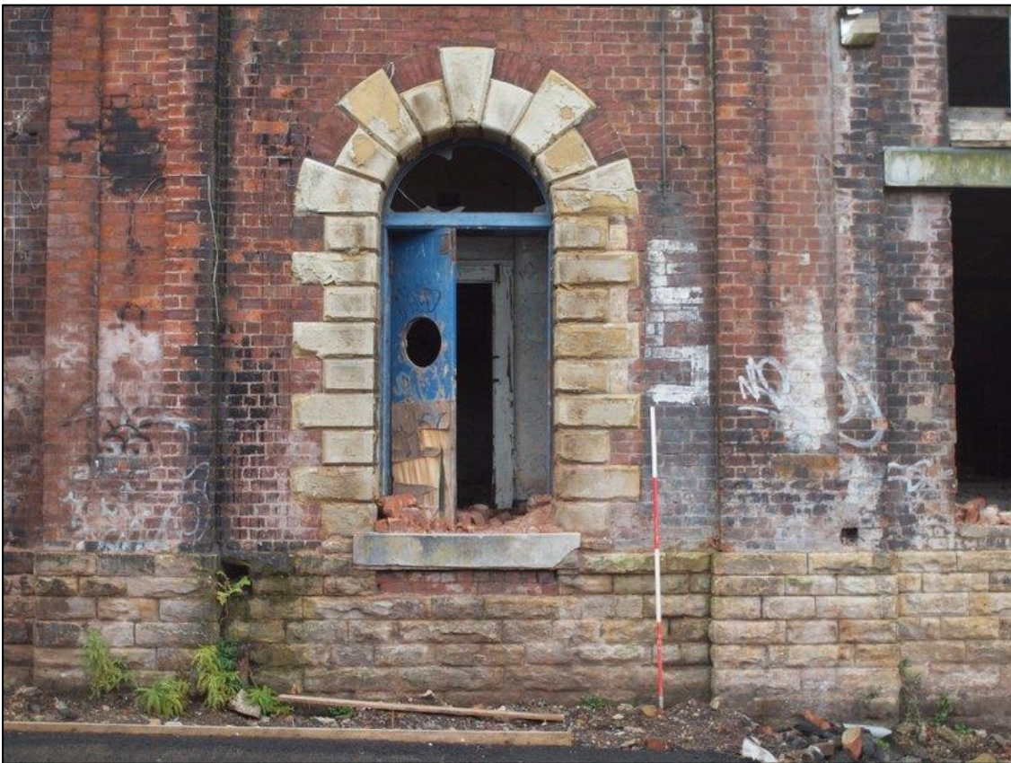
Plate 12: Detail of personnel door to engine house with steps removed
