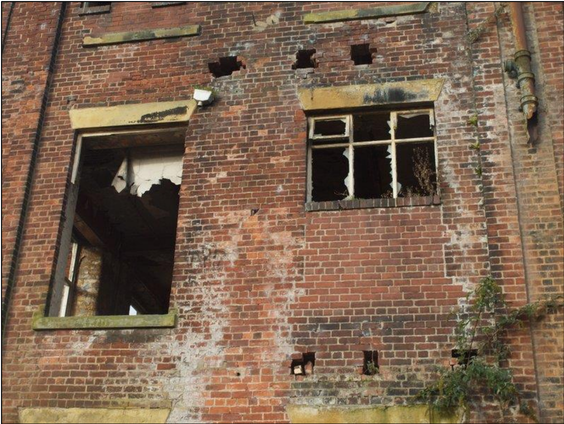
Plate 25: First floor windows of boiler house
