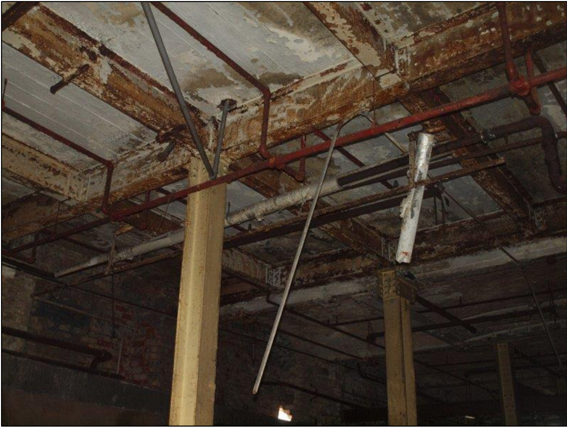
Plate 63: Detail of ceiling structure
