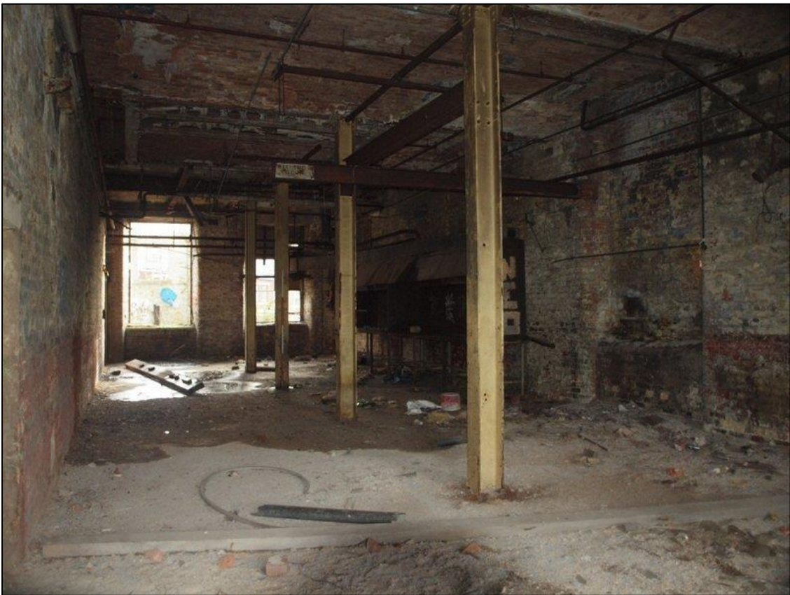
Plate 62: General shot of boiler house
