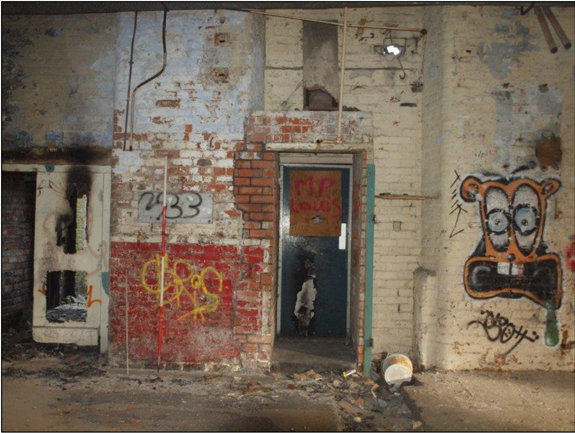
Plate 41: Detail of inserted doorway shown in plate 39
