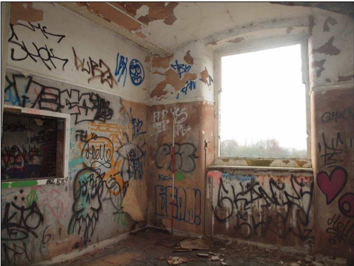
Plate 86: Inserted office in boiler house
