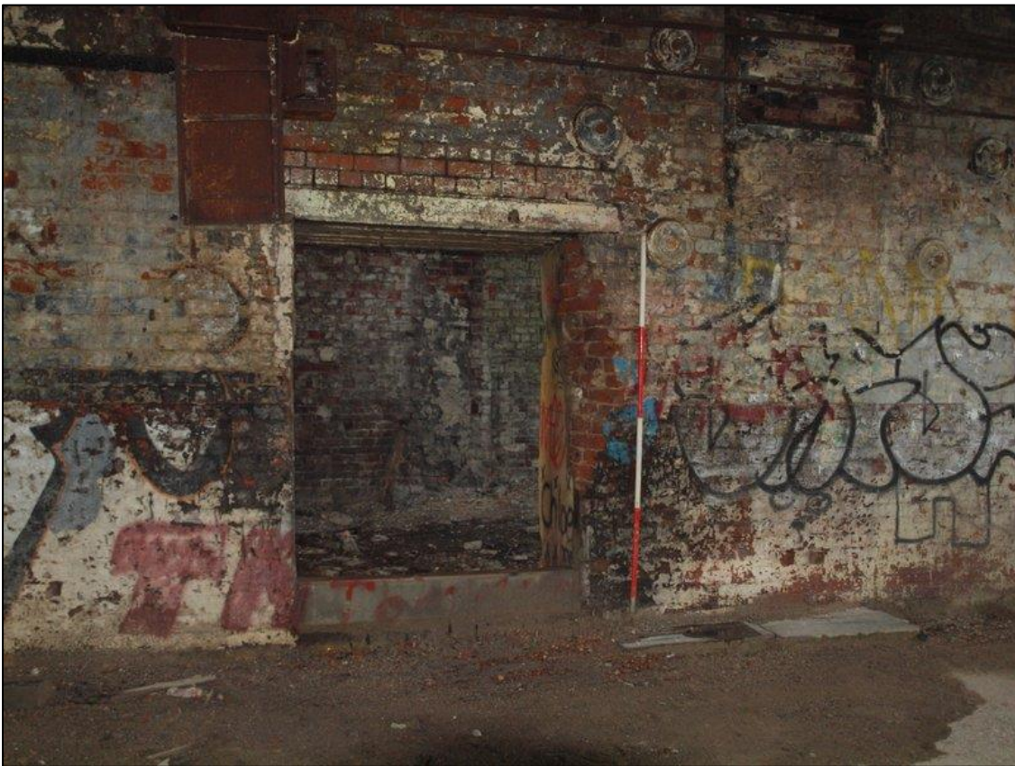
Plate 78: Central doorway to engine house
