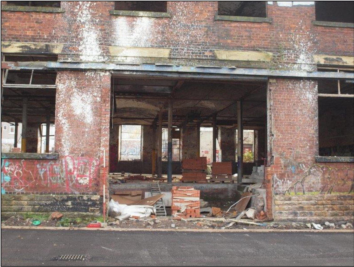
Plate 9: Detail of inserted doorway in bays 13 & 14
