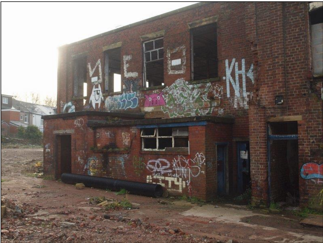
Plate 34: Single story extension on northeast elevation
