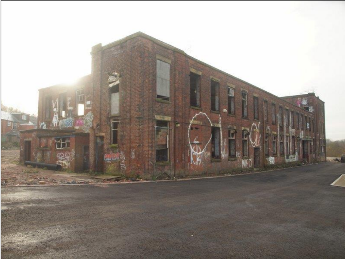
Plate 1: General shot of the mill
