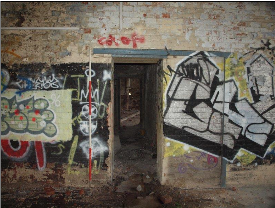
Plate 54: Detail of doorway into passage through engine room
