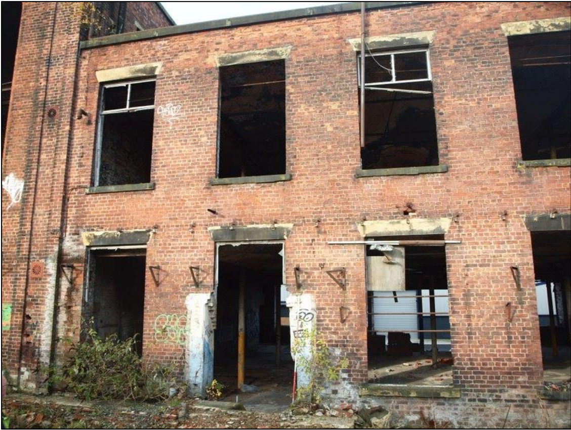
Plate 29: Southwest elevation bays 1 – 3, showing inserted doorway in bay 2
