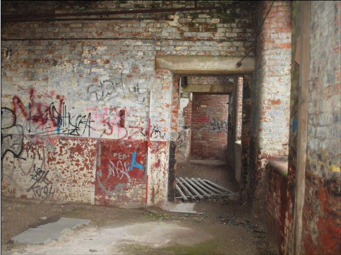
Plate 79: Western doorway to engine house
