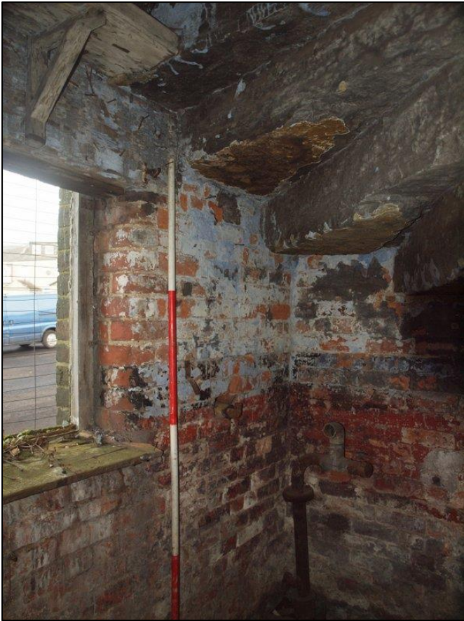
Plate 45: Room below staircase
