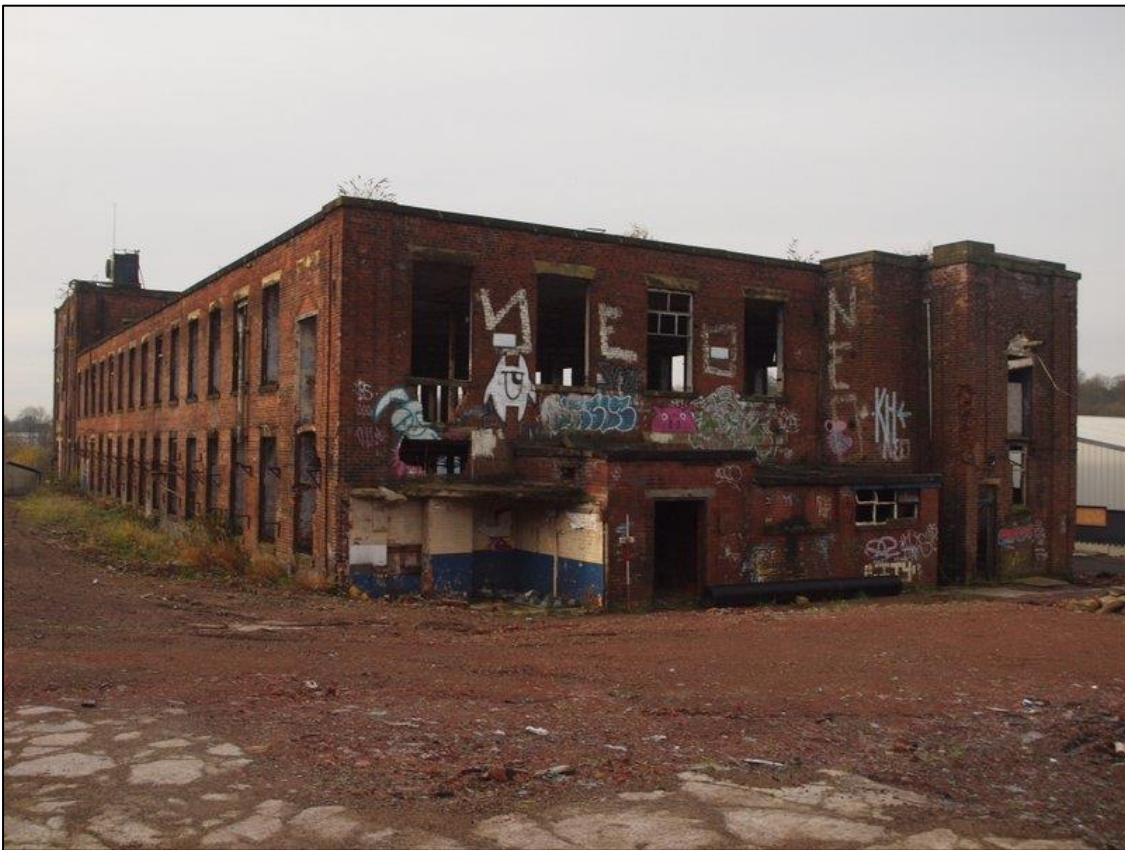
Plate 32: General shot of northeast elevation
