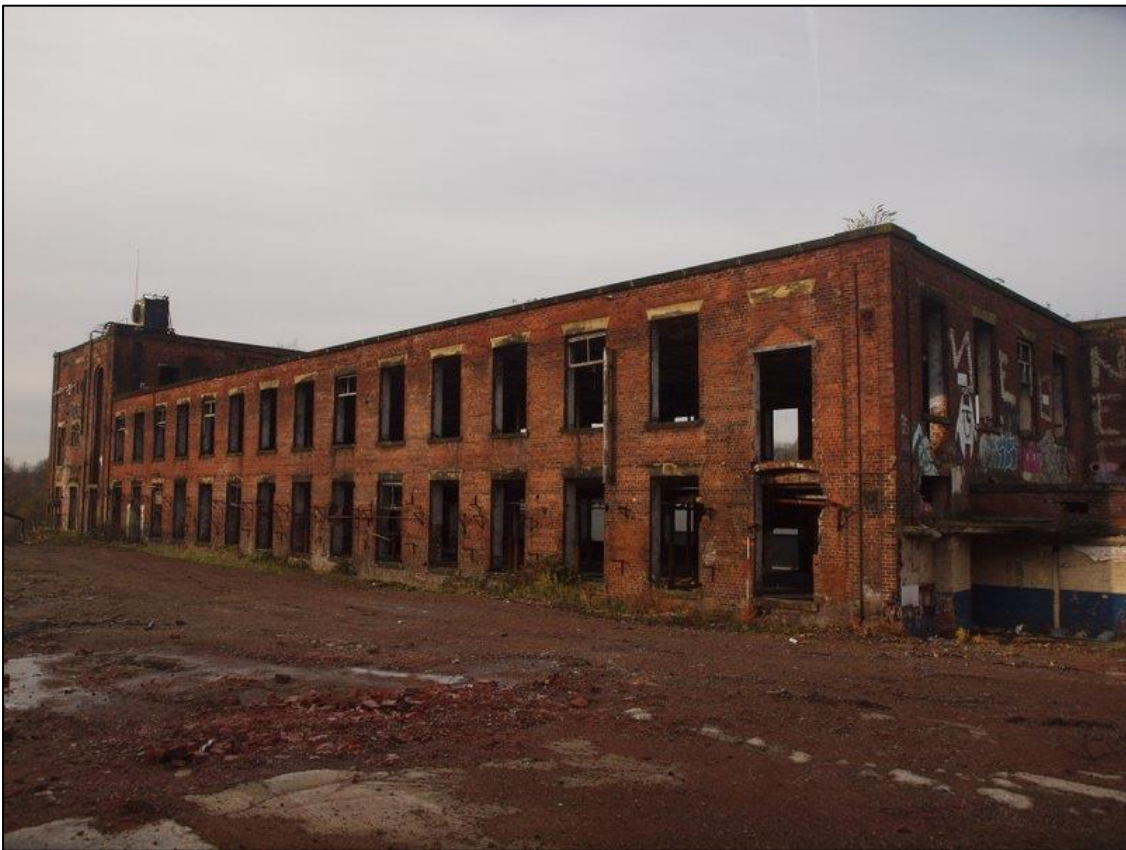
Plate 28: General shot of southwest elevation
