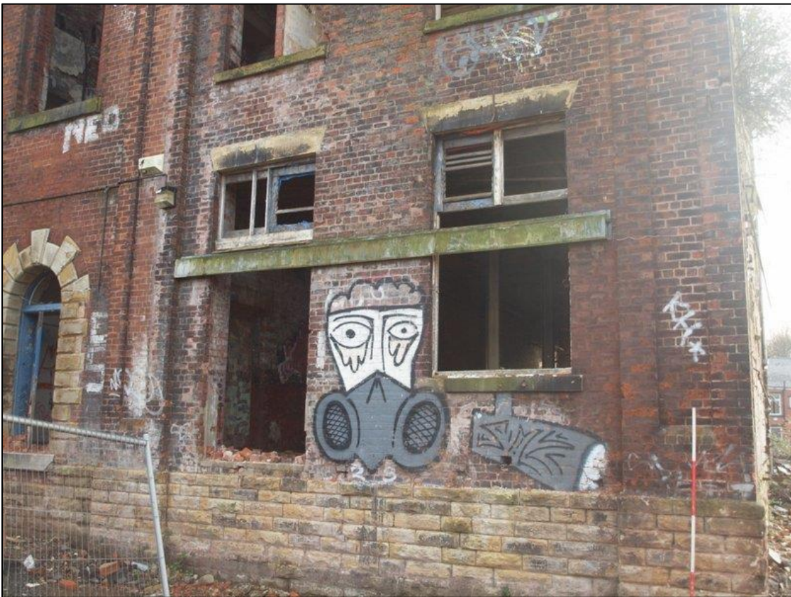
Plate 14: Detail of boiler house ground floor
