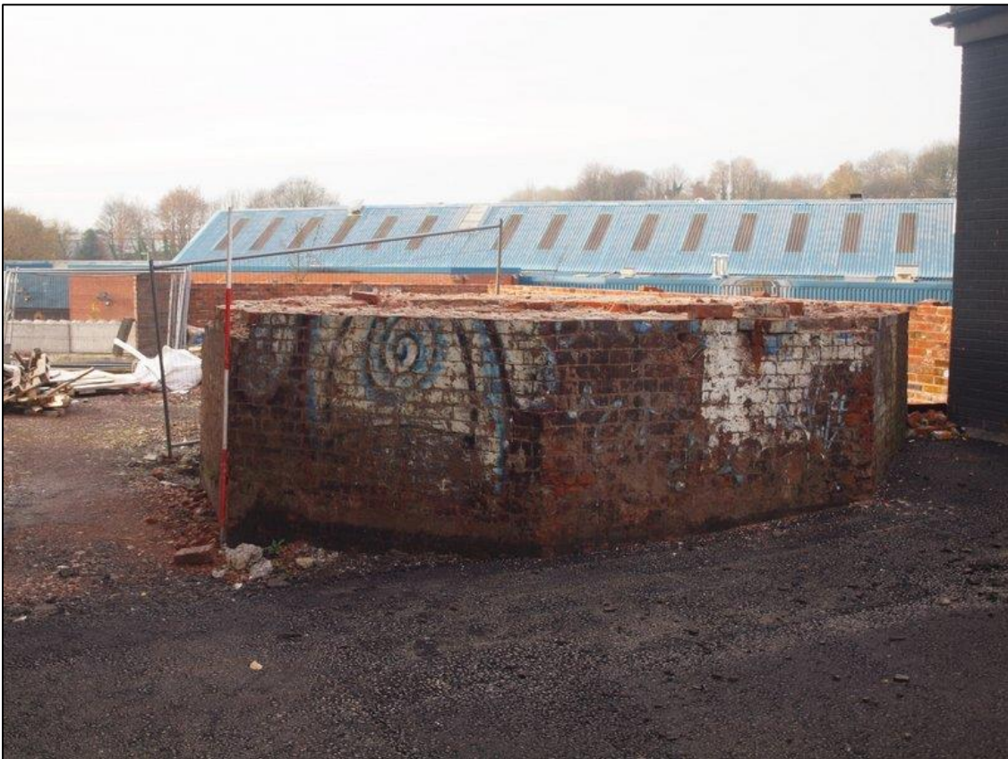
Plate 2: Octagonal chimney base
