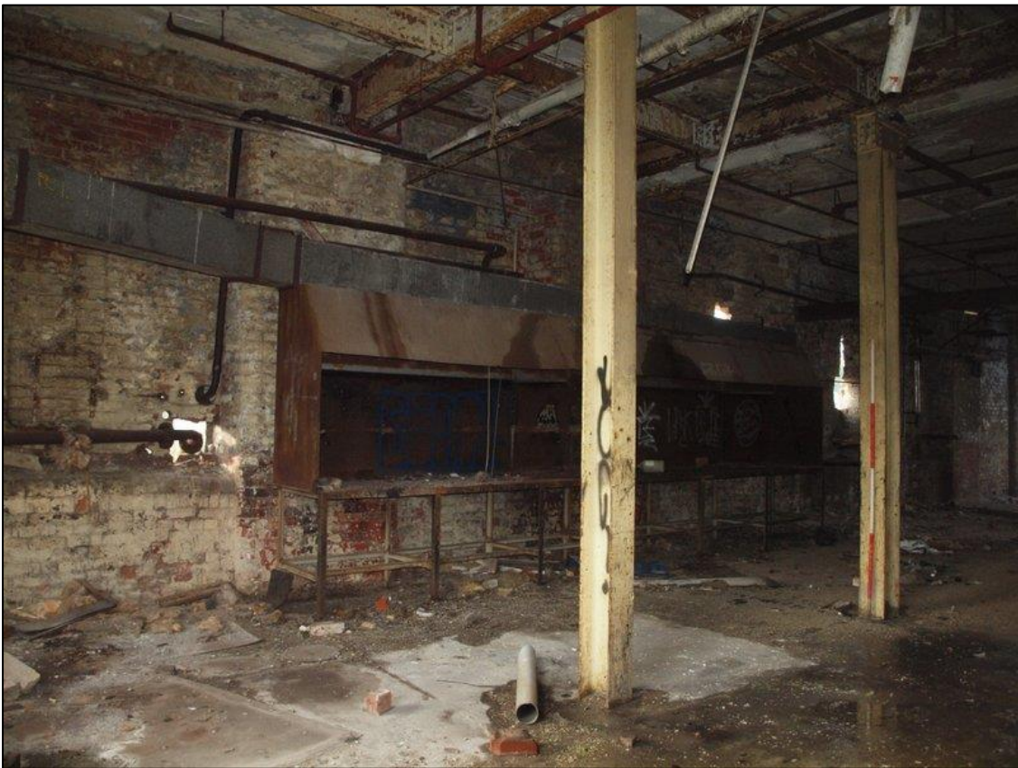
Plate 60: General shot of boiler house
