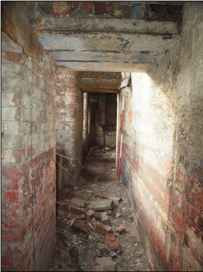
Plate 59: Passage at east end leading into boiler house
