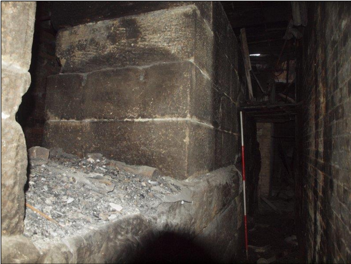
Plate 57: As above viewed from the other direction, showing inset for high pressure cylinder
