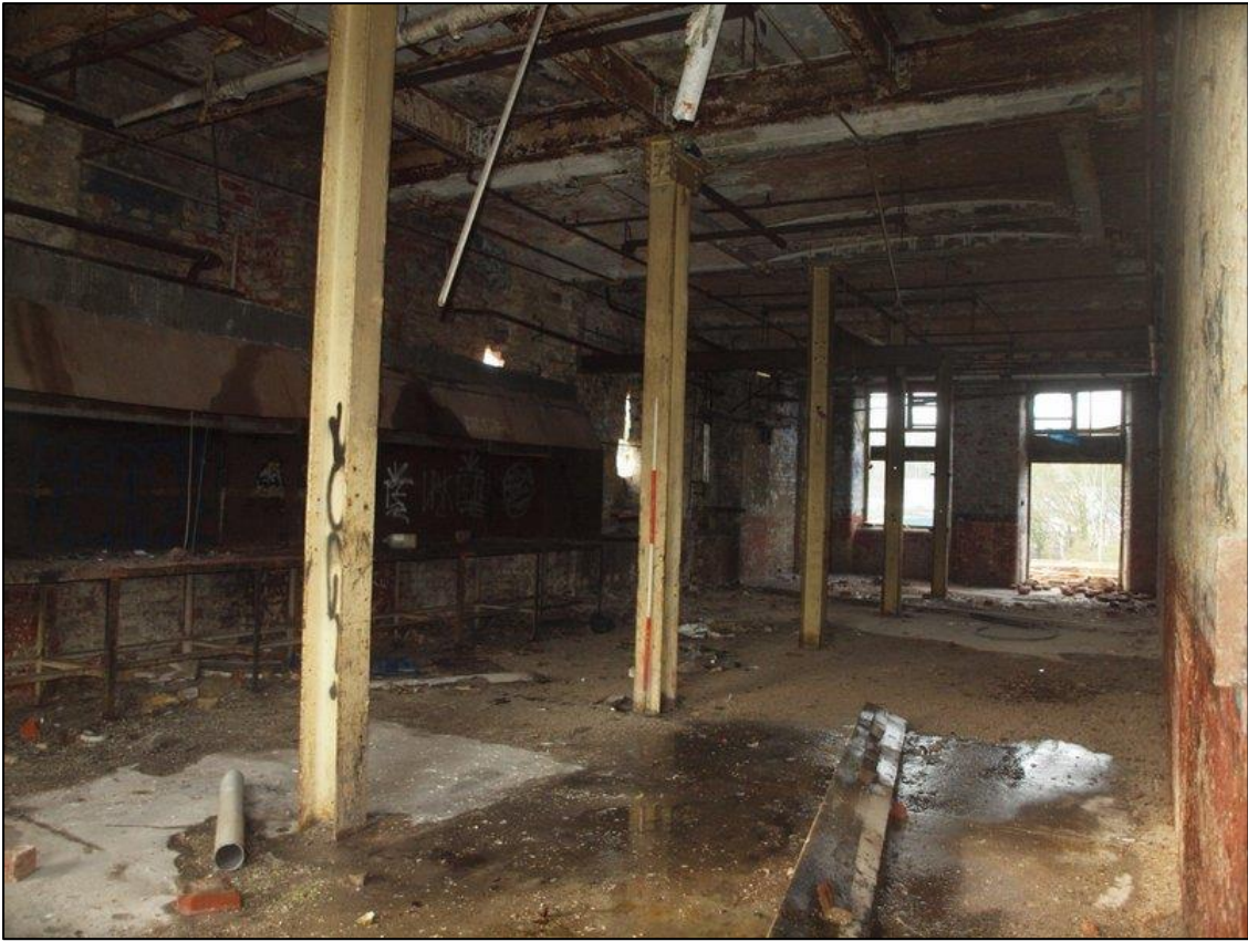
Plate 61: General shot of boiler house
