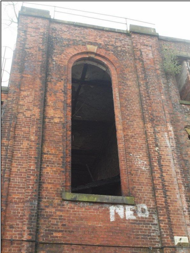
Plate13: Detail of first and second floor engine house window
