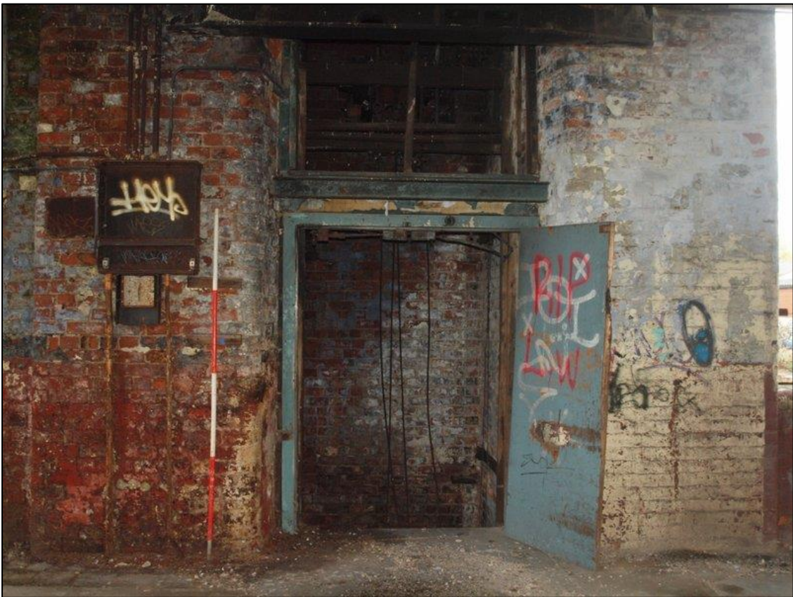
Plate 70: Detail of lift shaft doorway
