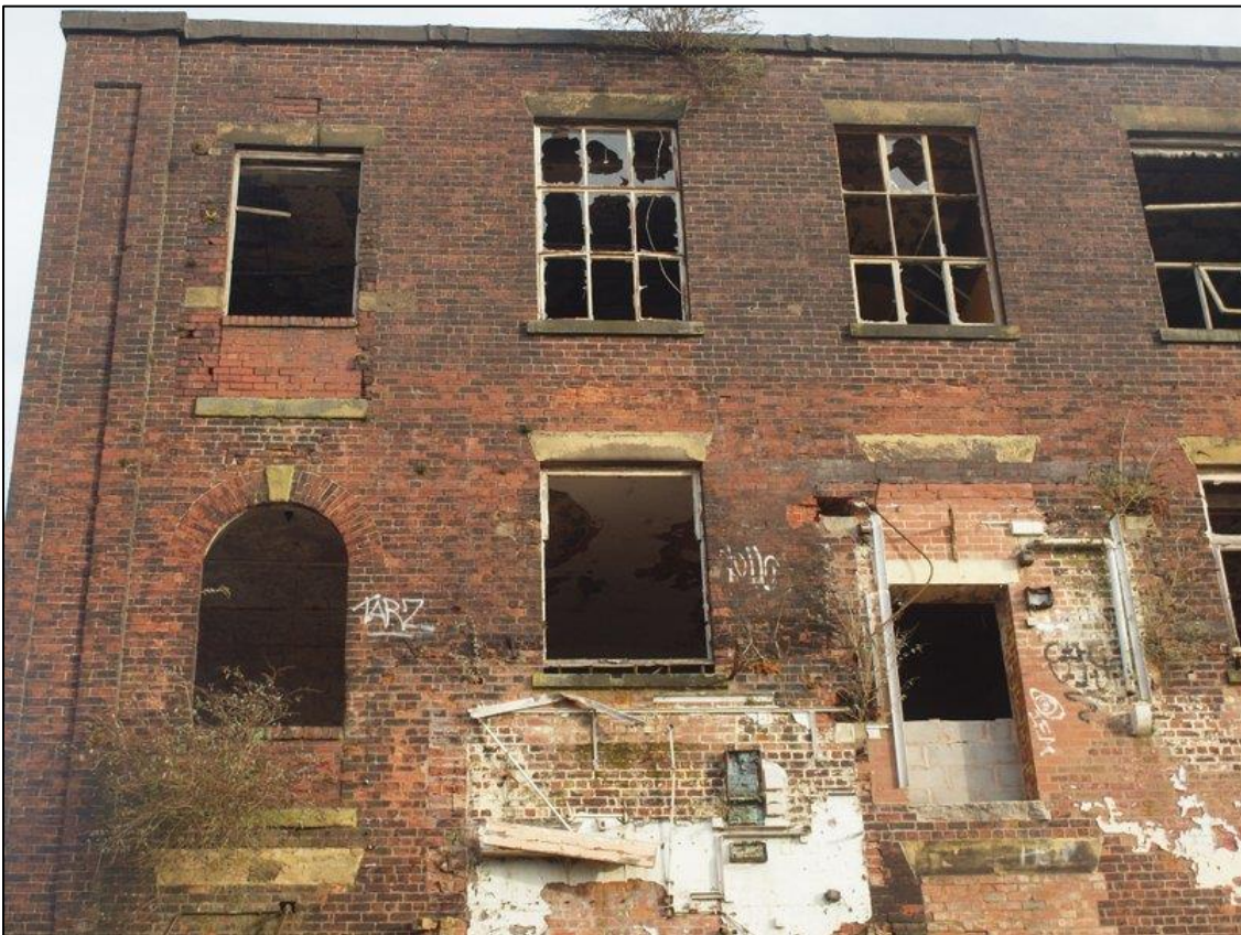
Plate 18: Southwest elevation bays 1 – 3 at first and second floor levels
