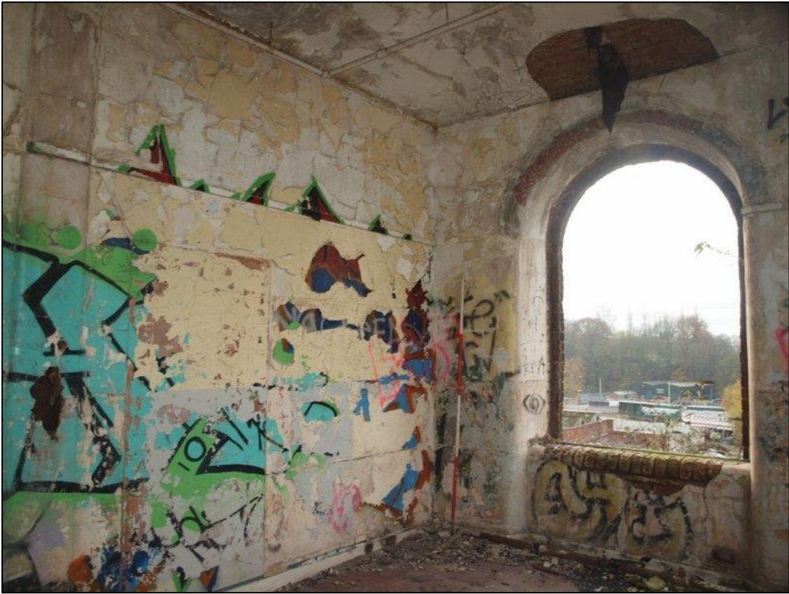
Plate 85: Inserted office in boiler house
