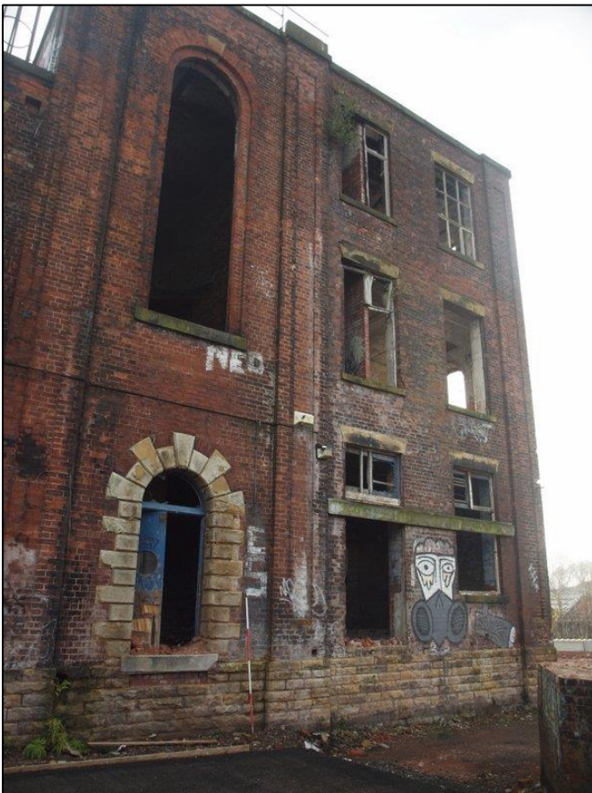
Plate 10: Engine house (left) and boiler house (right)
