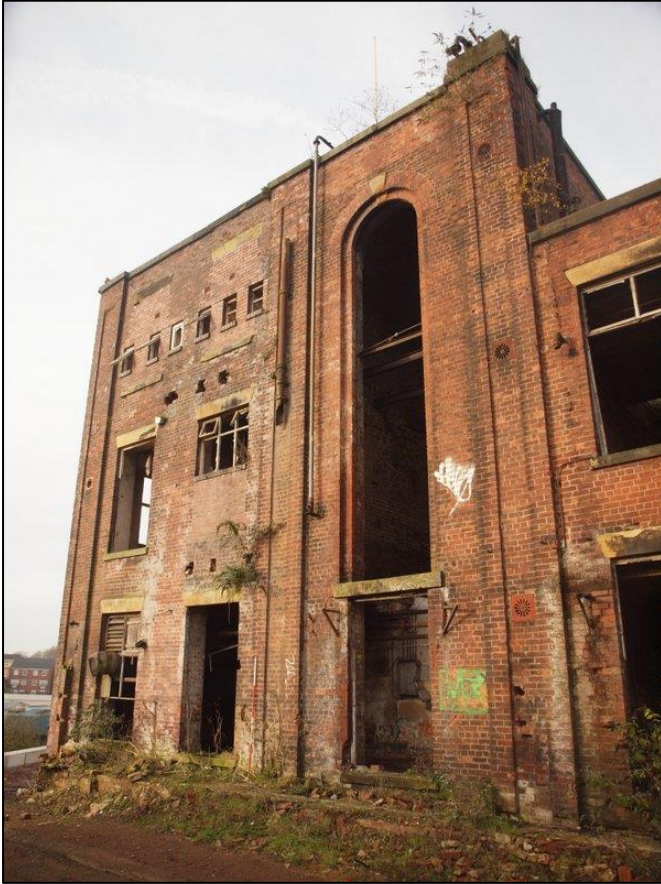
Plate 23: Southeast elevation showing boiler house (left) and engine house (right)
