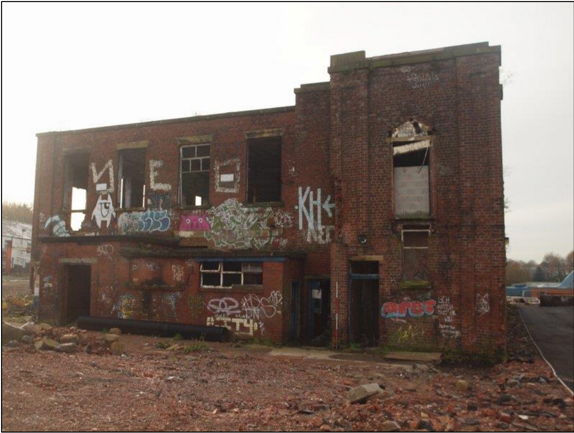
Plate 33: General shot of northeast elevation
