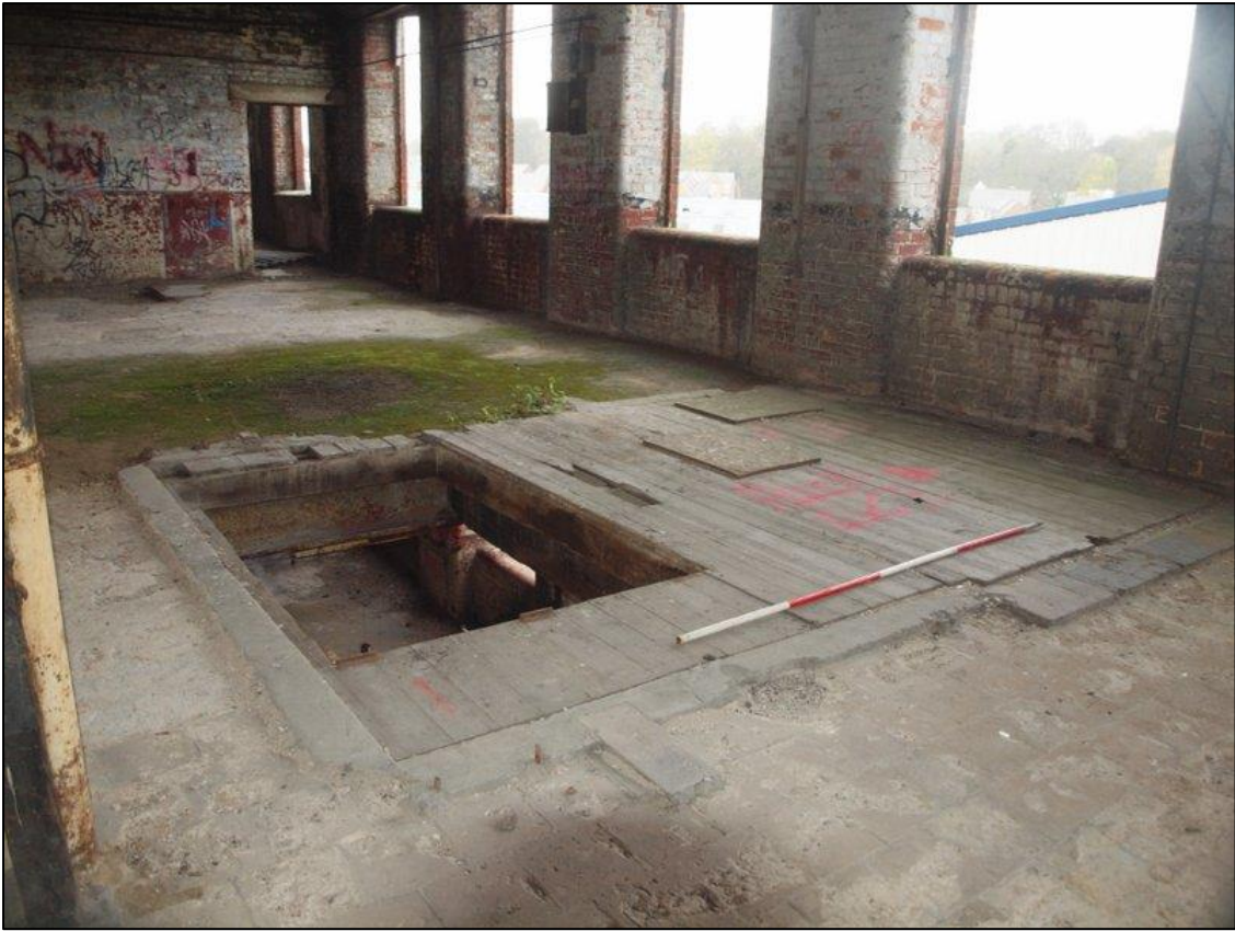
Plate 71: Detail of loading hatch in floor in bay 13
