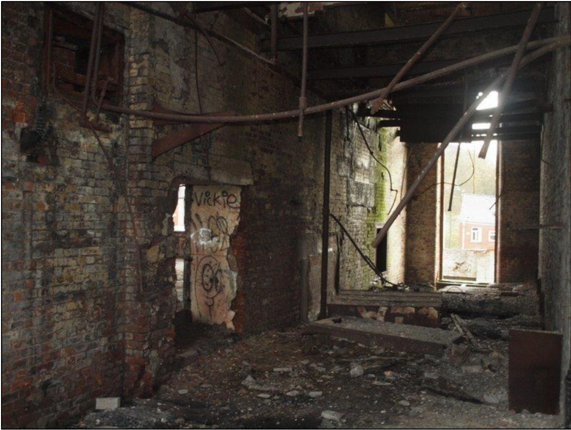
Plate 81: General shot of engine house
