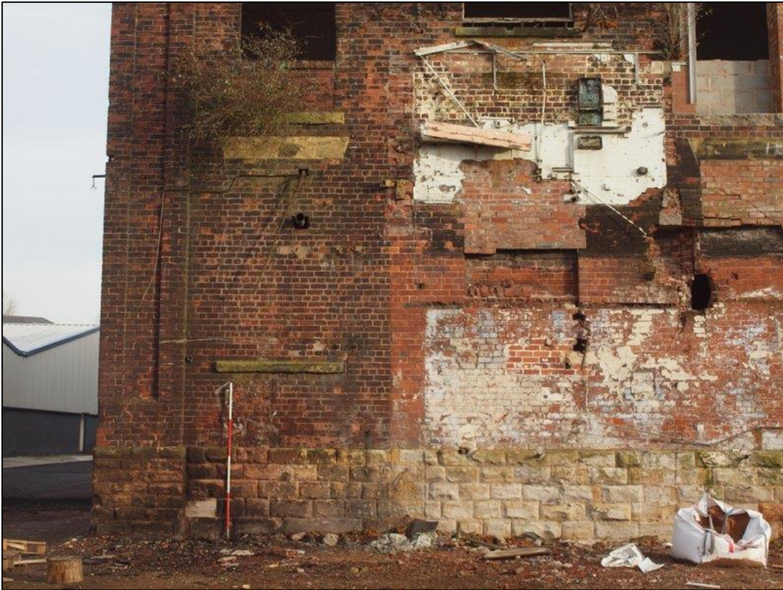
Plate 17: Blocked window in bay 1 at ground floor level
