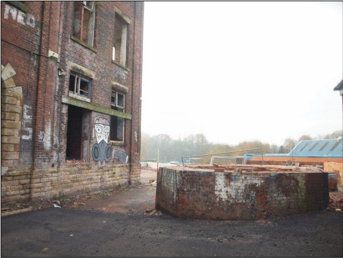
Plate 3: Chimney base in relation to the boiler house Northwest Elevation
