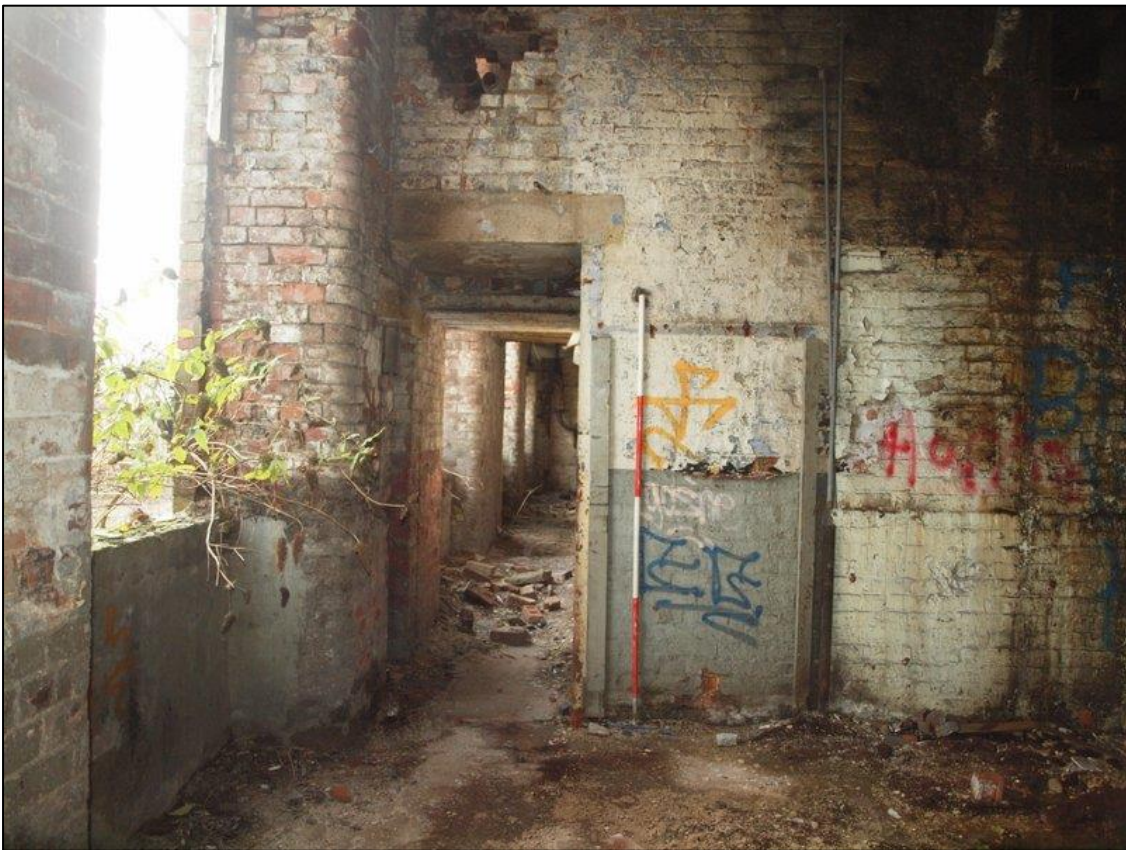
Plate 50: Doorway at eastern end leading directly to boiler house
