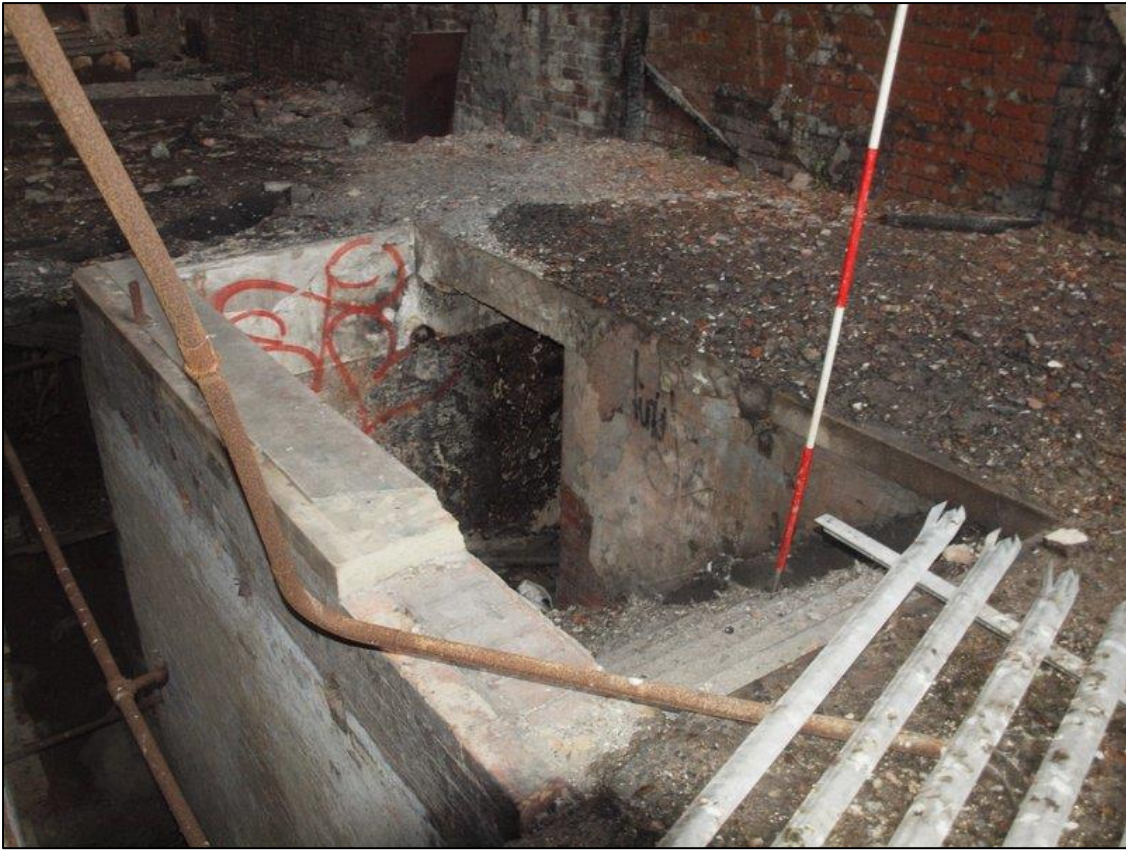
Plate 83: Concrete staircase to ground floor
