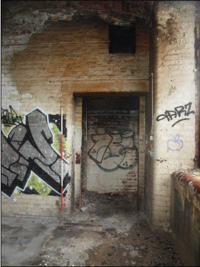
Plate 55: Detail of blocked doorway to boiler house
