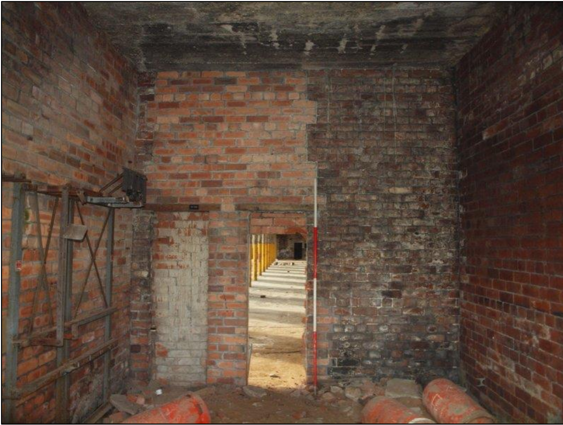
Plate 47: Storage room in extension showing inserted doorways and blocked window
