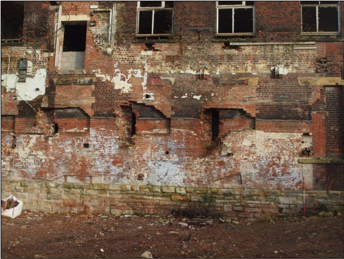
Plate 21: Southwest elevation showing ground floor bays 3 - 6
