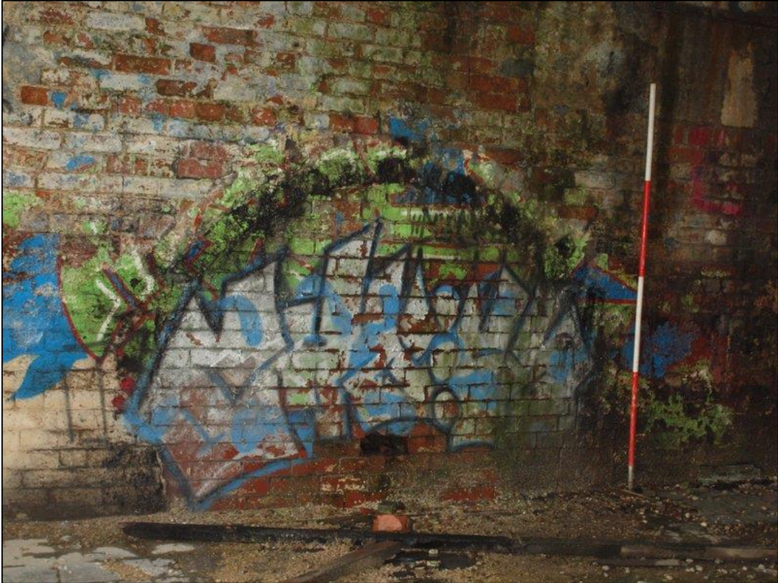
Plate 75: Arched brickwork in southwest wall
