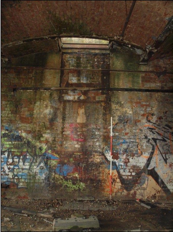
Plate 73: Detail of transmission window with hole in ceiling above
