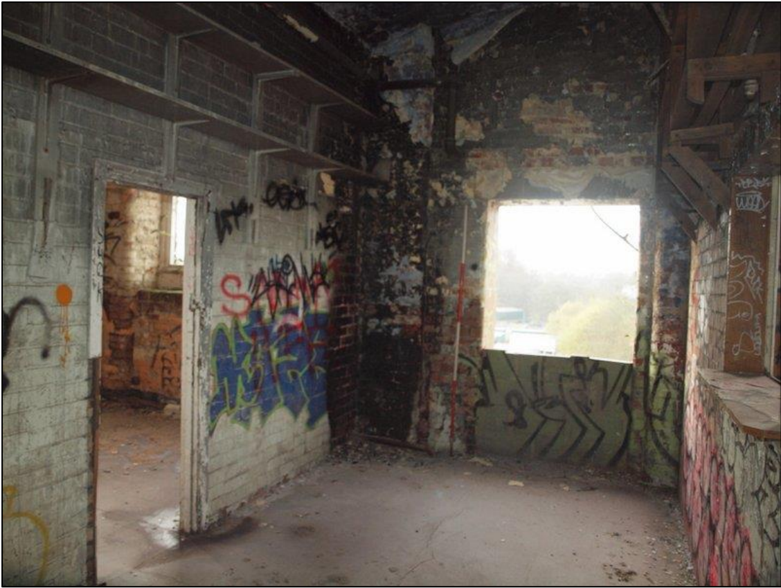
Plate 87: Inserted office in boiler house
