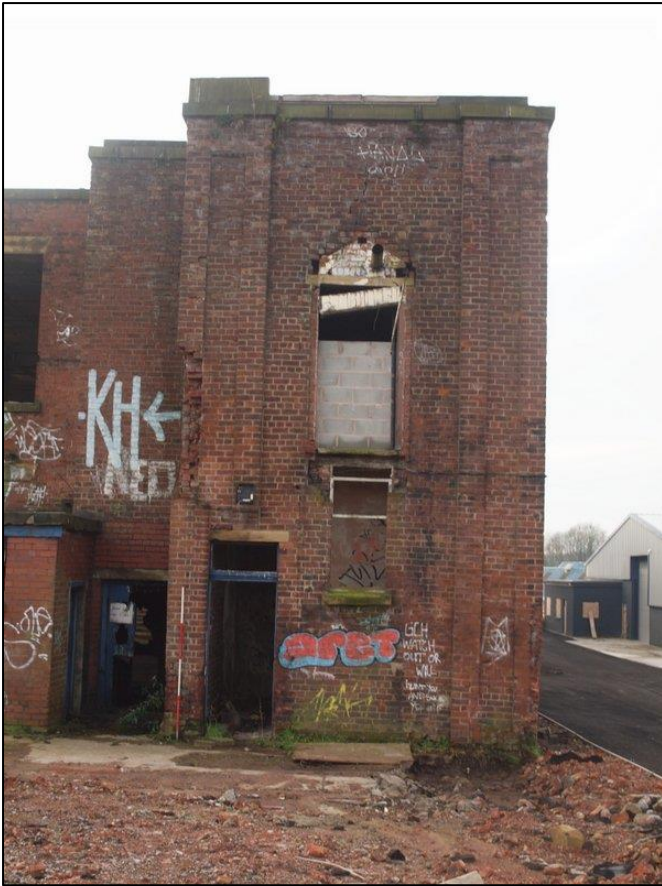
Plate 35: Detail of stair tower in bay 6 Interior – Ground floor
