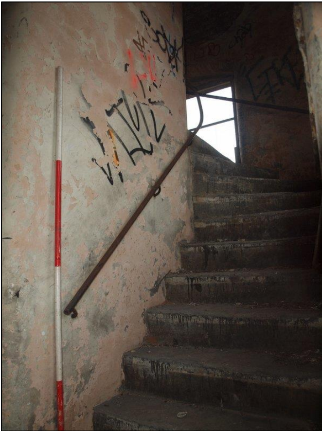
Plate 46: Detail of staircase
