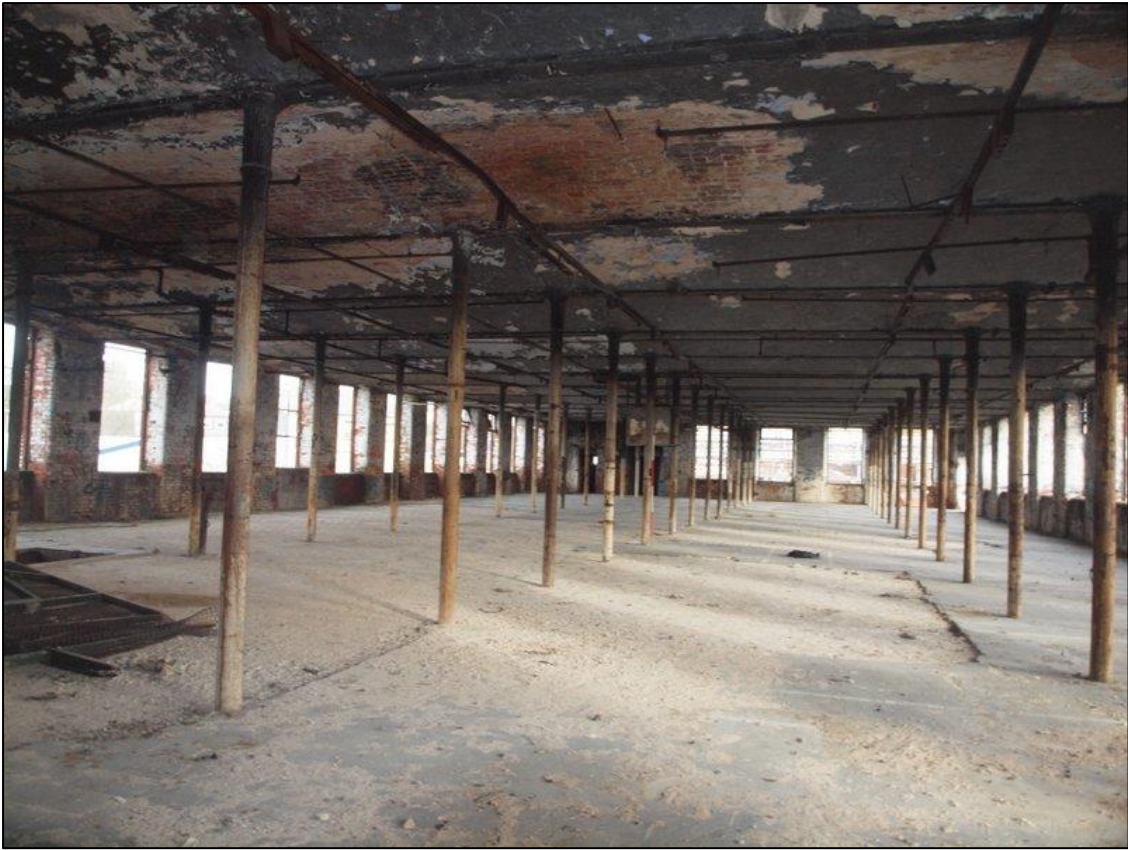
Plate 67: General shot of first floor of mill
