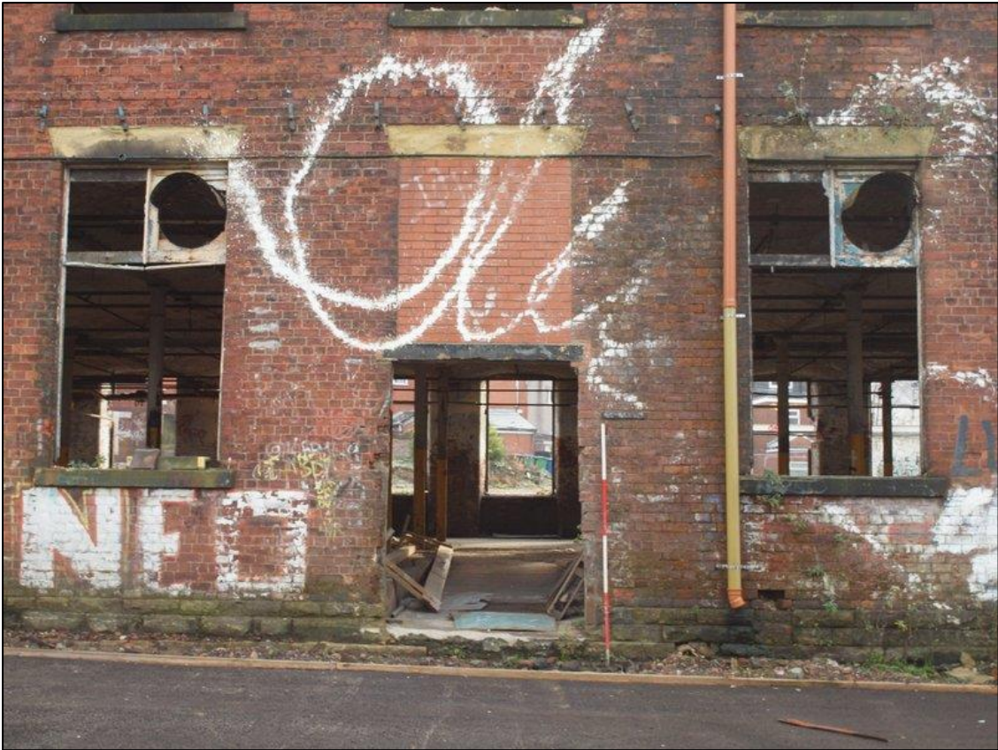
Plate 7: Detail of inserted doorway in bay 6
