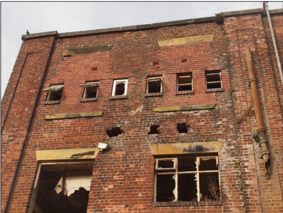
Plate 26: Second of boiler house showing blocked and inserted windows
