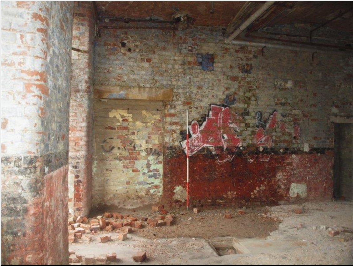
Plate 65: Blocked doorway to engine house
