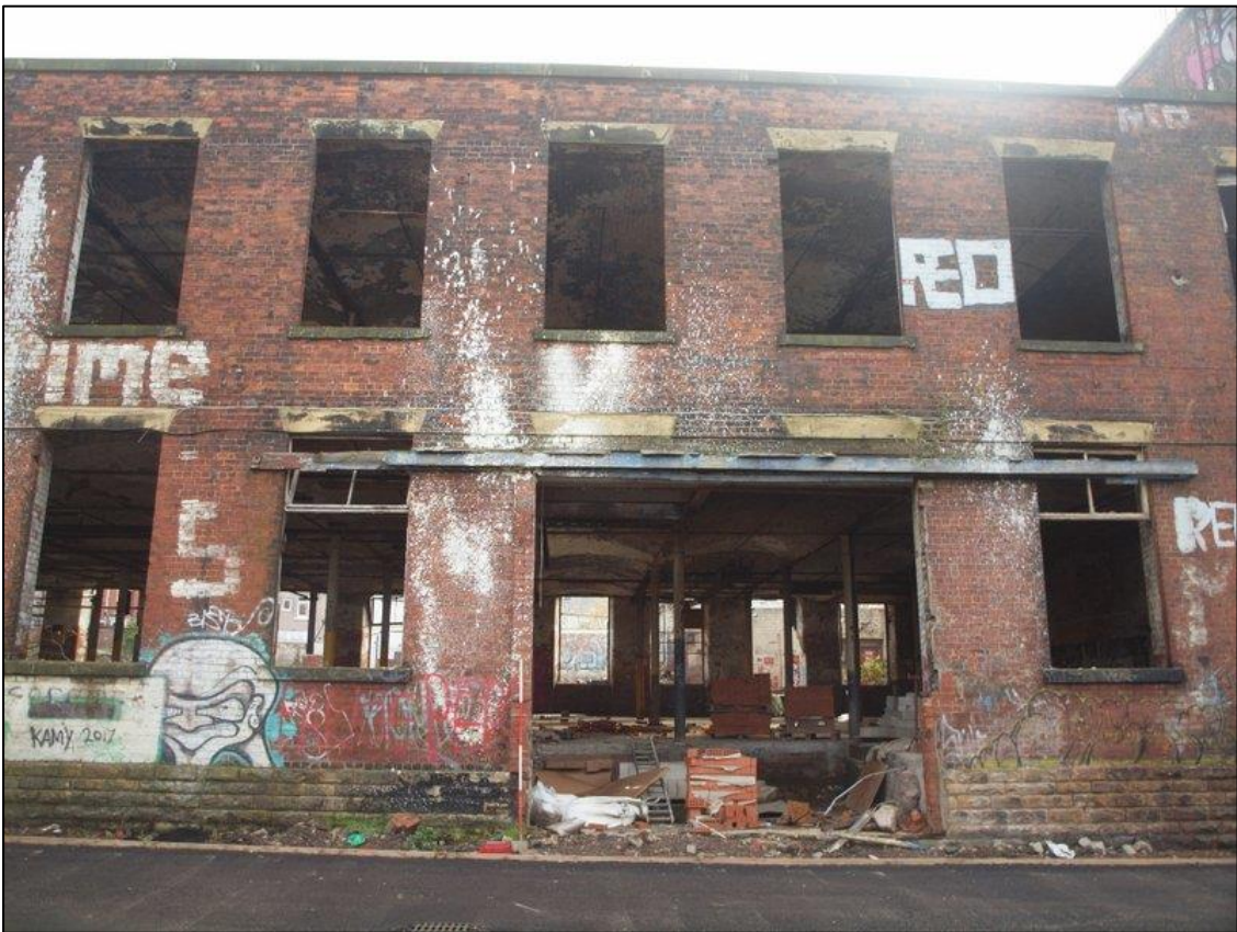
Plate 8: Northwest elevation bays 11 - 15
