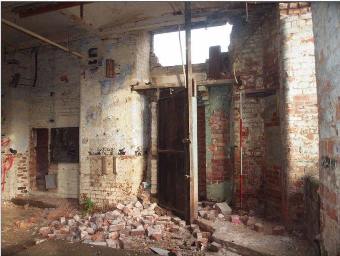
Plate 44: Detail of inserted doorway behind timber screen
