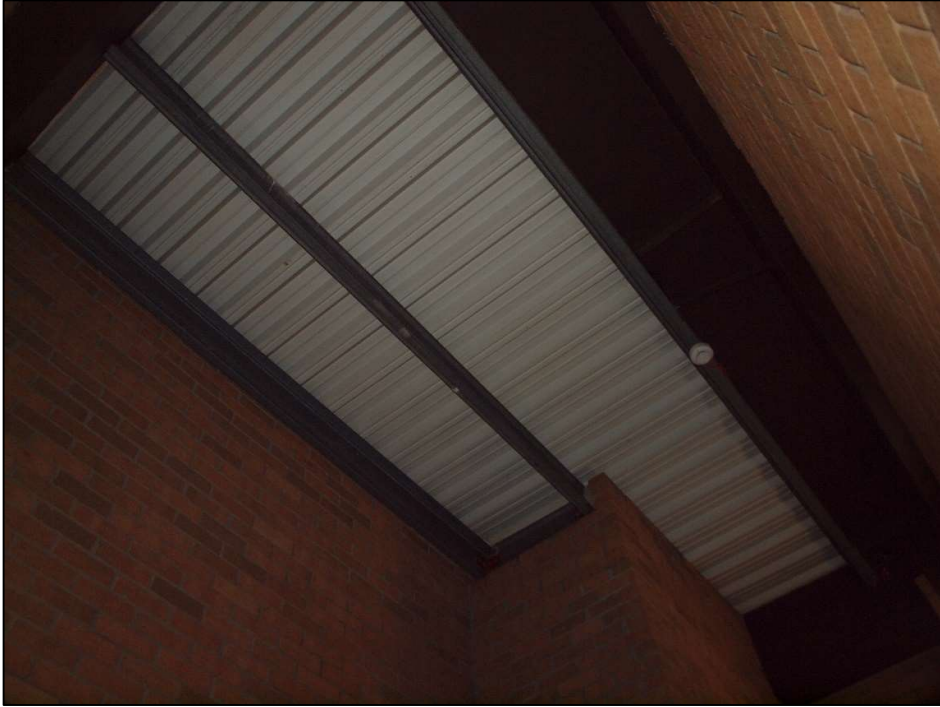
Plate 43: Detail of corrugated metal roof visible in staircase.
