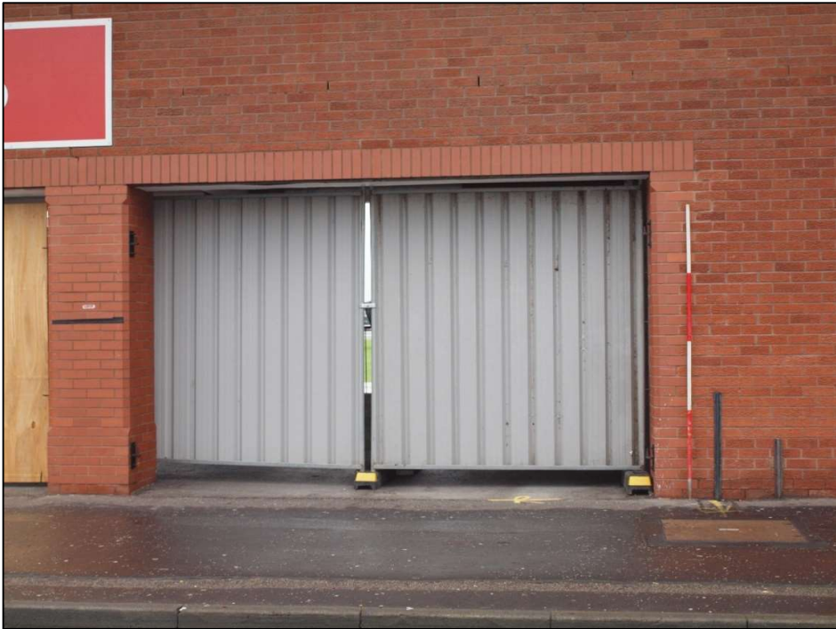
Plate 14: Detail of ground floor opening
