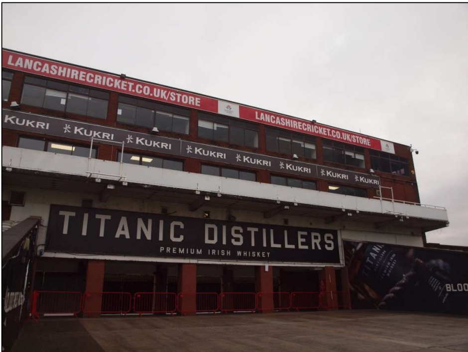
Plate 6: West elevation showing ground access
