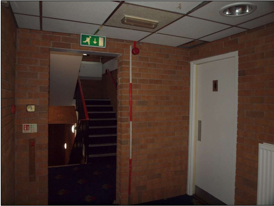
Plate 27: Southern end of corridor showing staircase and toilets
