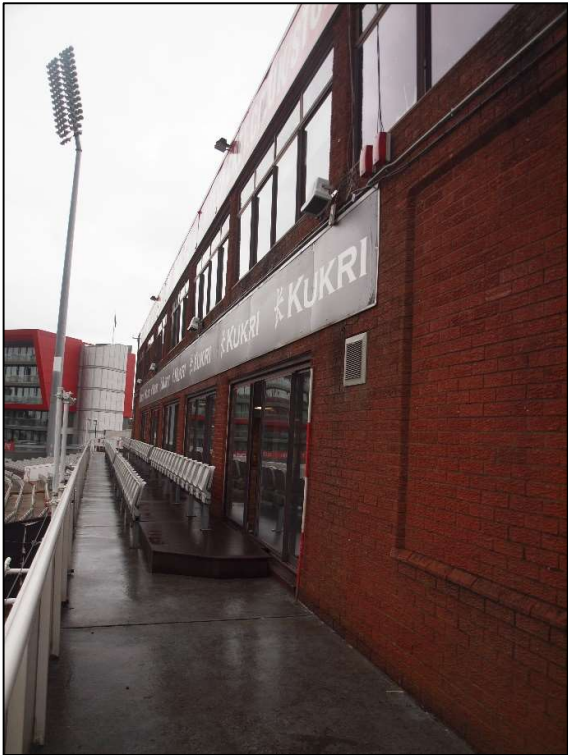
Plate 10: Detail of west elevation, second floor level to Red Rose Suite
