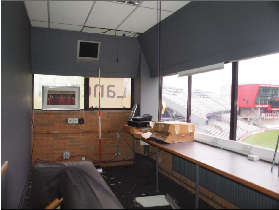
Plate 41: Room to southern end of press box
