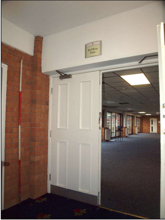
Plate 31: Second floor landing showing entrance to Red Rose Suite
