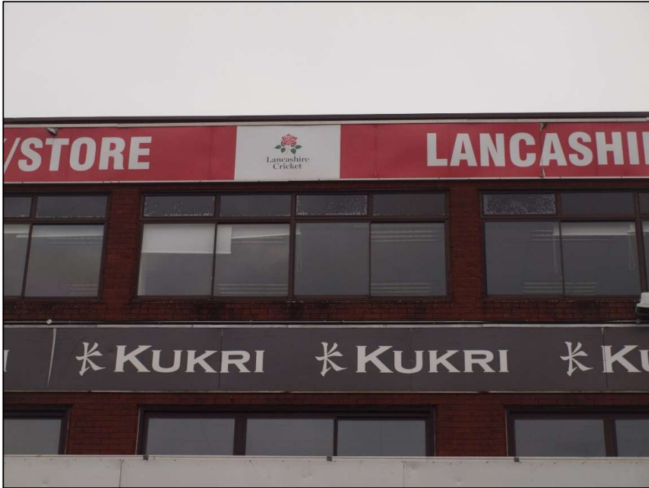
Plate 7: Detail of third floor windows to west elevation
