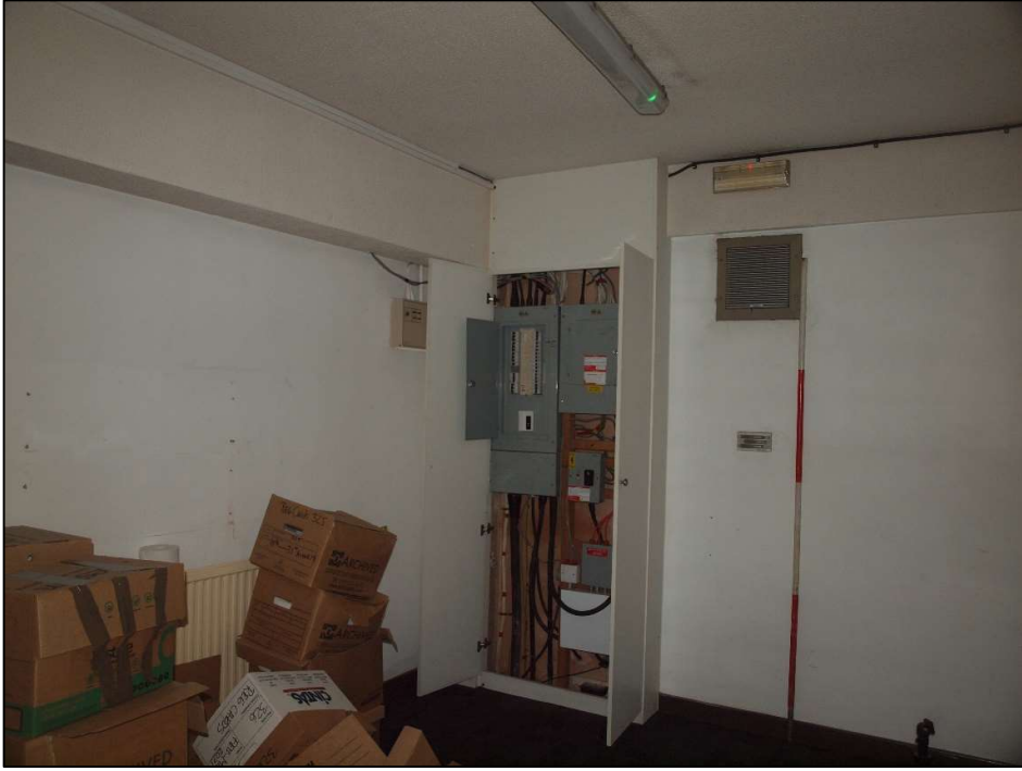
Plate 23: Storage room to south of kitchen
