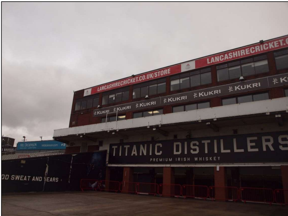
Plate 8: North end of west elevation
