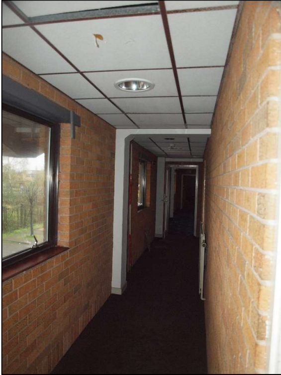
Plate 21: Corridor running south down east side of building
