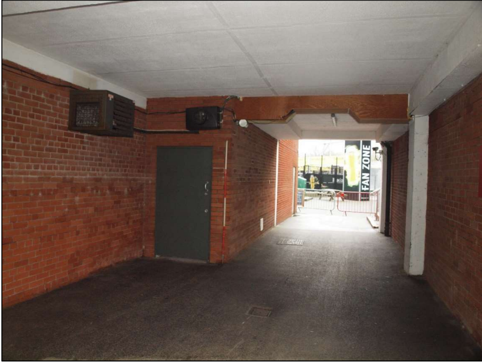
Plate 19: As above looking north
