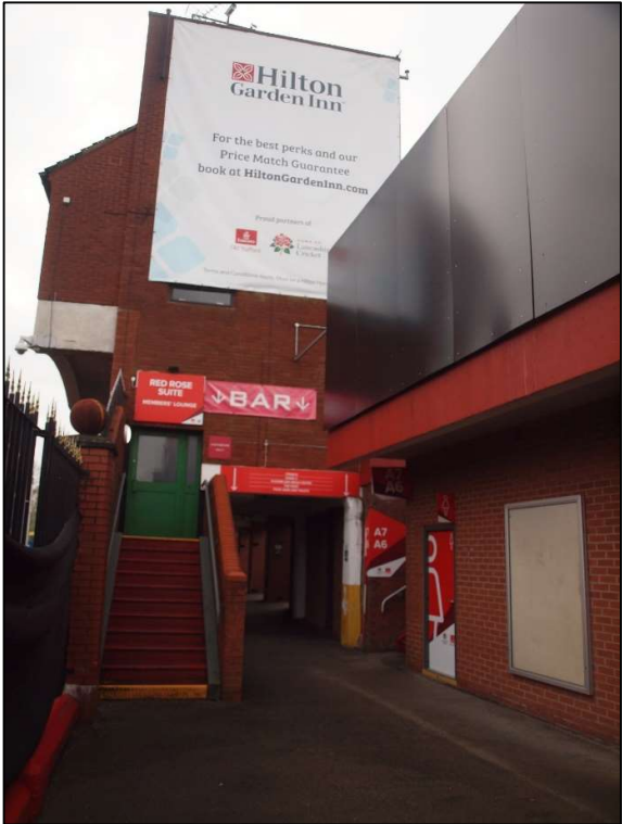
Plate 1: North elevation of building
