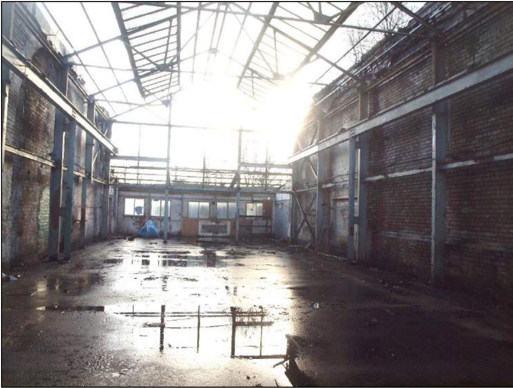
Plate 21: Interior of northern extension.
