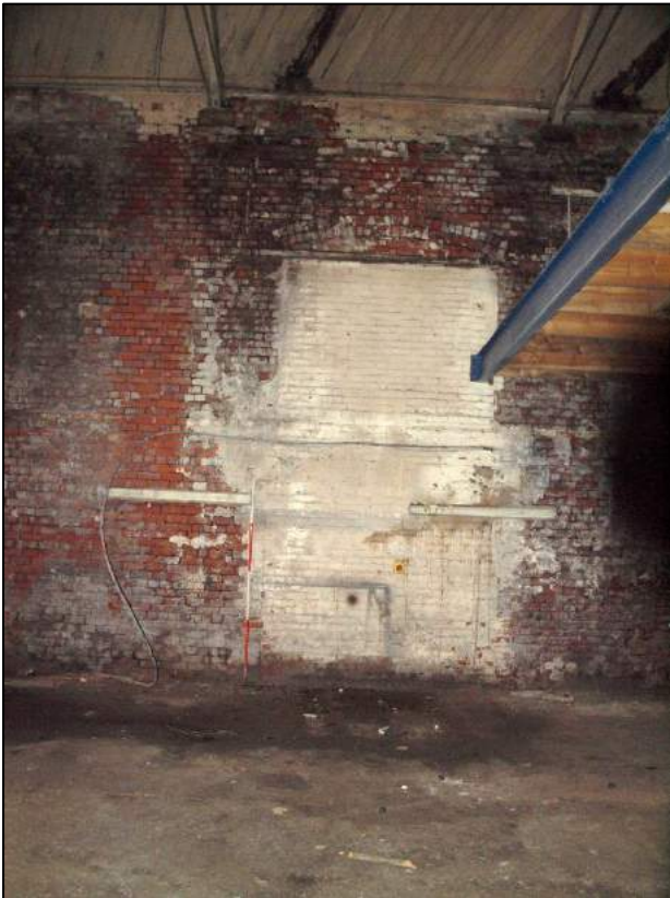
Plate 30: Window with inserted and blocked loading door at east end of north wall.
