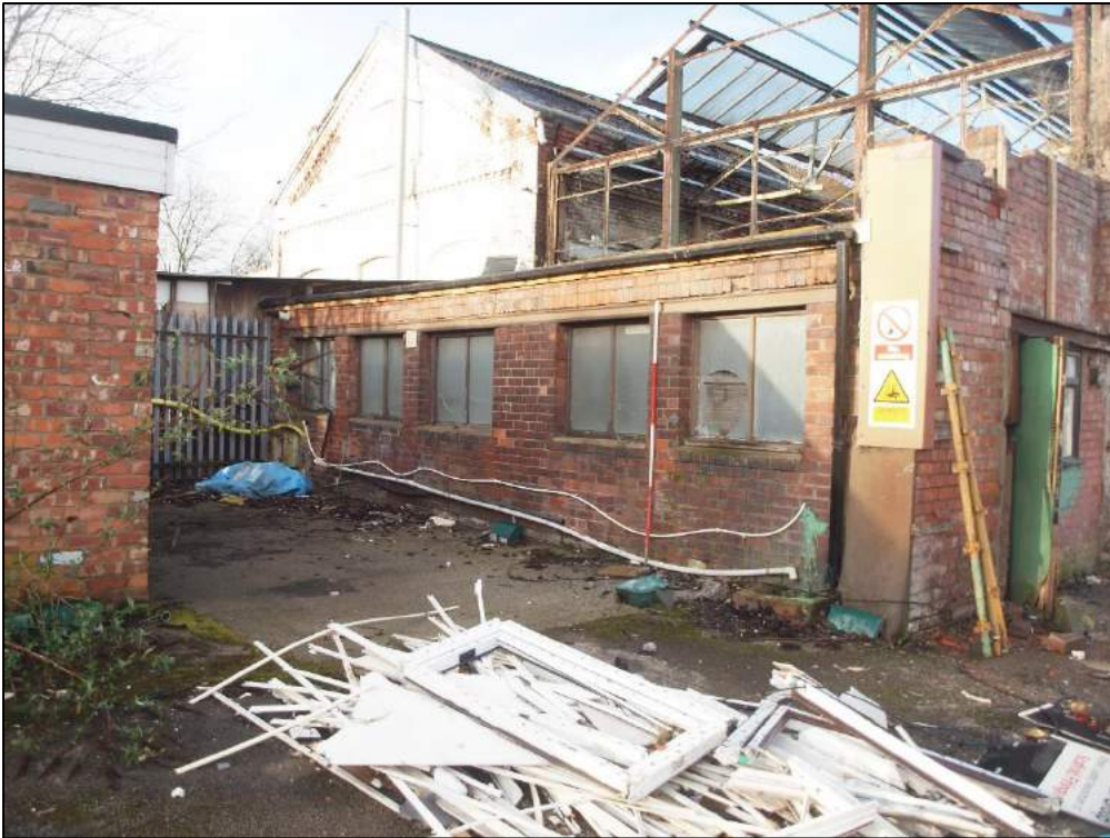
Plate 15: Northern end of east elevation.
