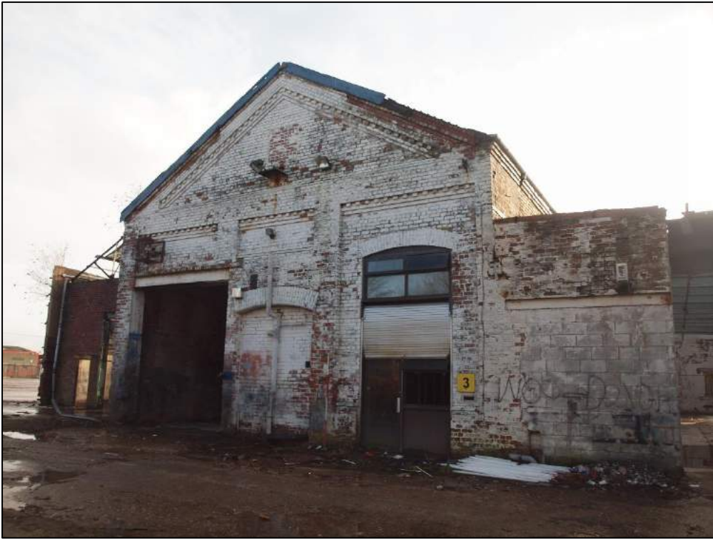
Plate 3: Western gable of central building.
