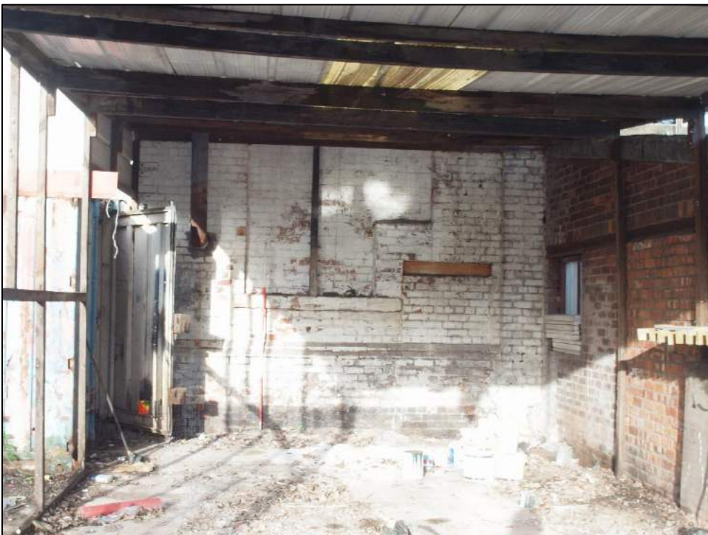
Plate 14: Detail of inserted and blocked personnel doorway in window.
