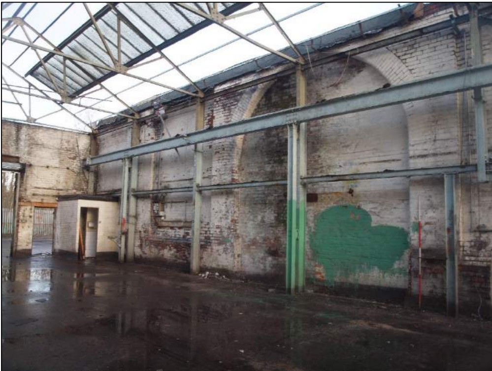
Plate 24: North wall (former external wall of factory) showing arched opening.
