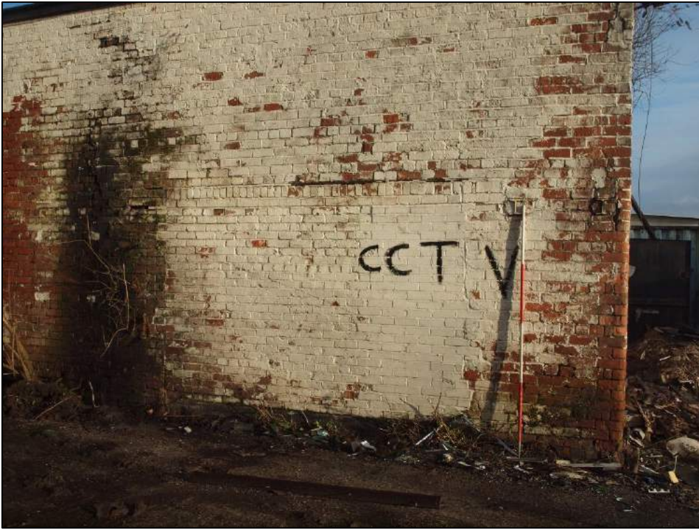
Plate 11: Blocked loading door at east end.
