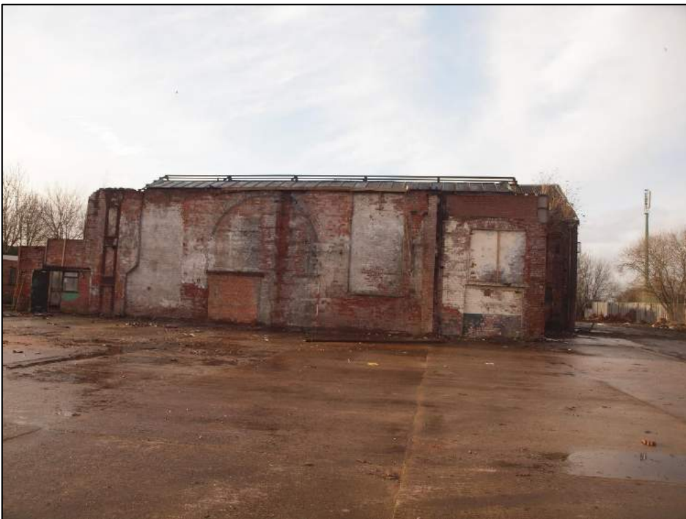
Plate 16: North elevation (former internal elevation of factory).
