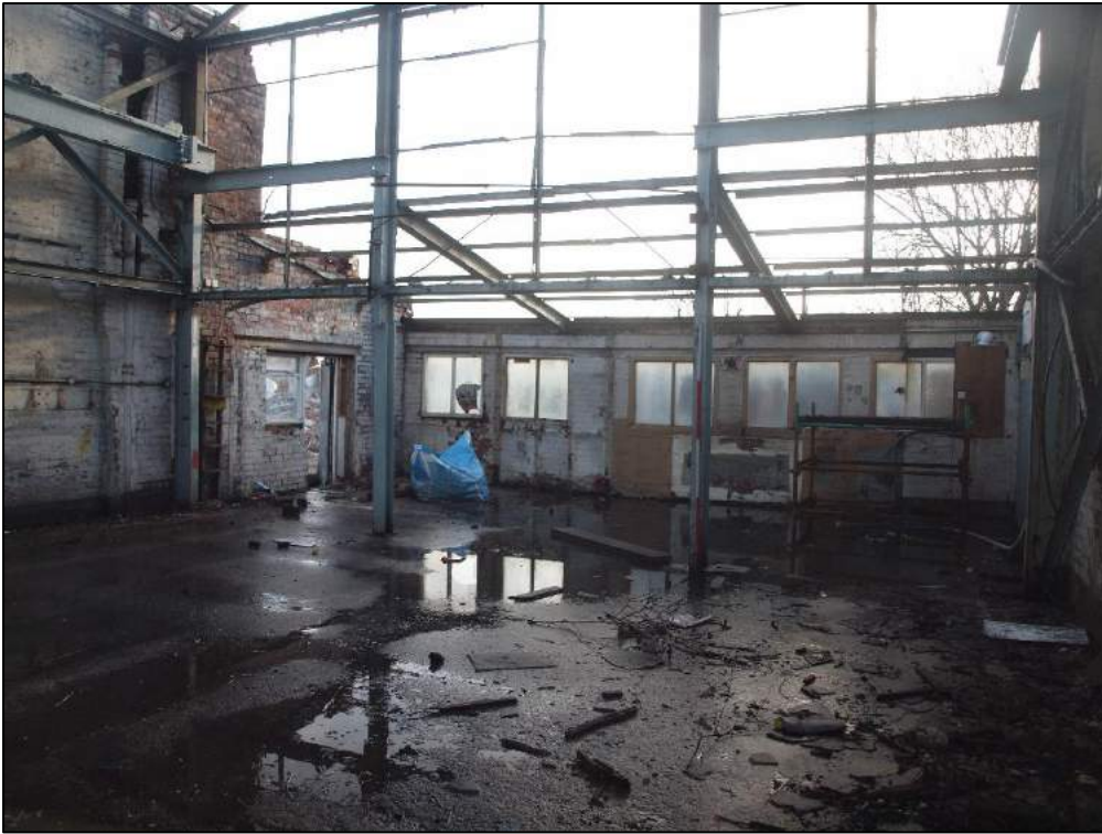
Plate 23: Single story extension to the east.
