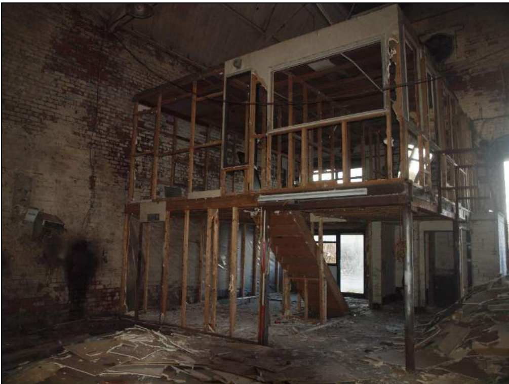
Plate 34: Detail of inserted stud walling.
