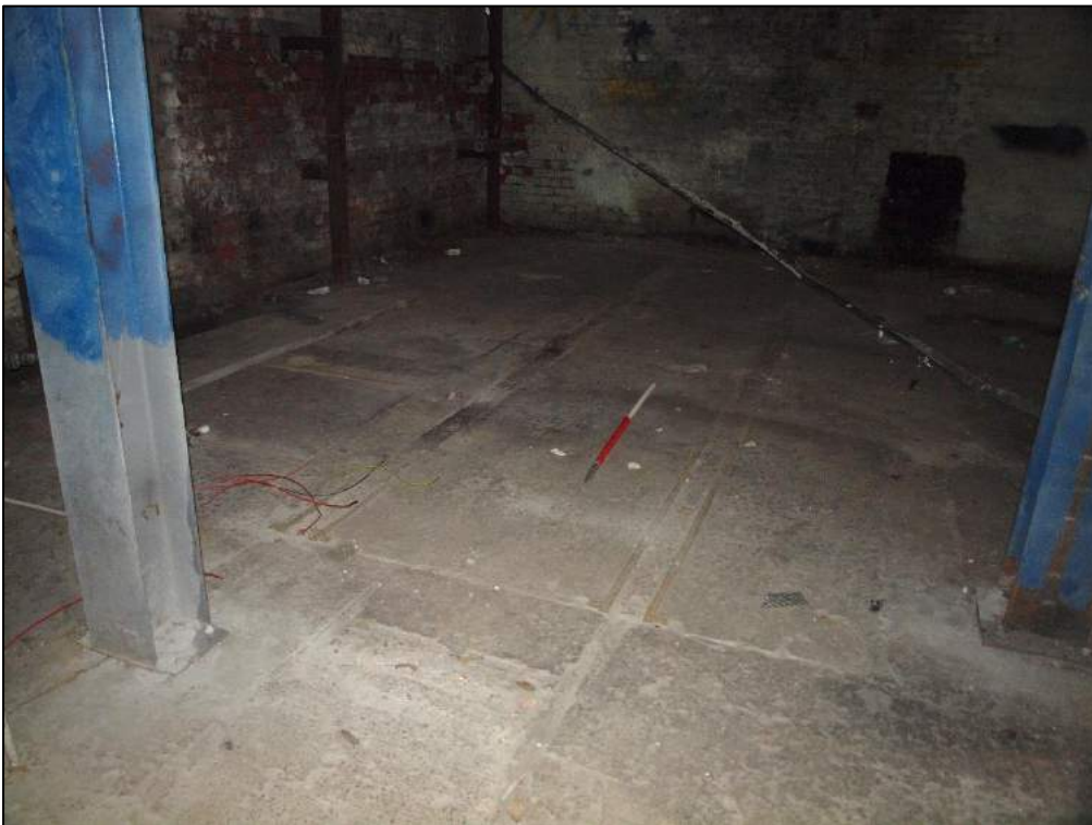
Plate 36: Detail of metal runners found within concrete at east end.
