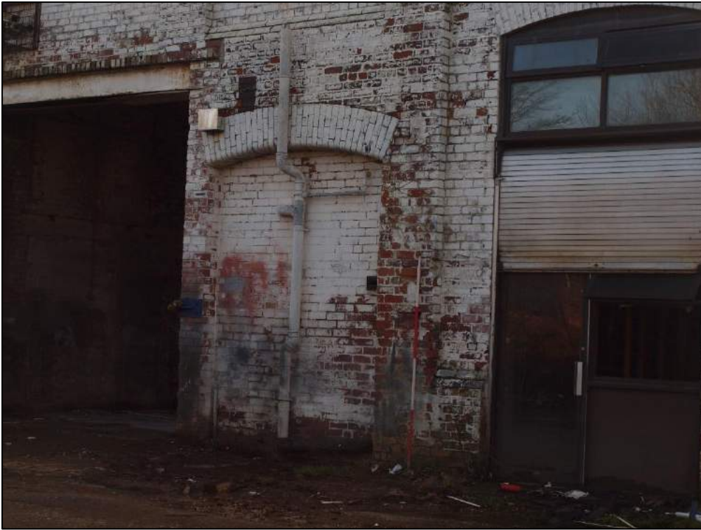
Plate 5: Detail of central blocked doorway.
