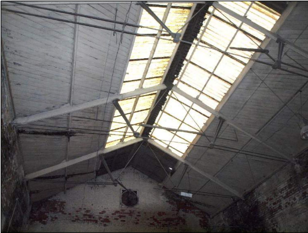
Plate 35: Detail of roof structure.
