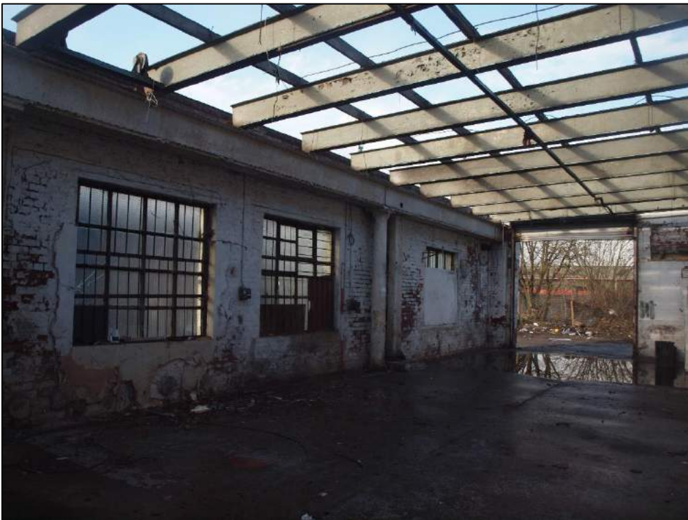
Plate 42: Southern wall showing roof structure.
