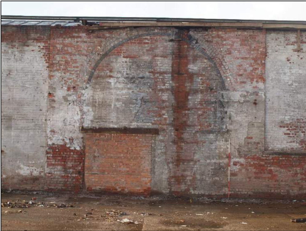
Plate 17: Arched opening with inserted and blocked loading doorway.
