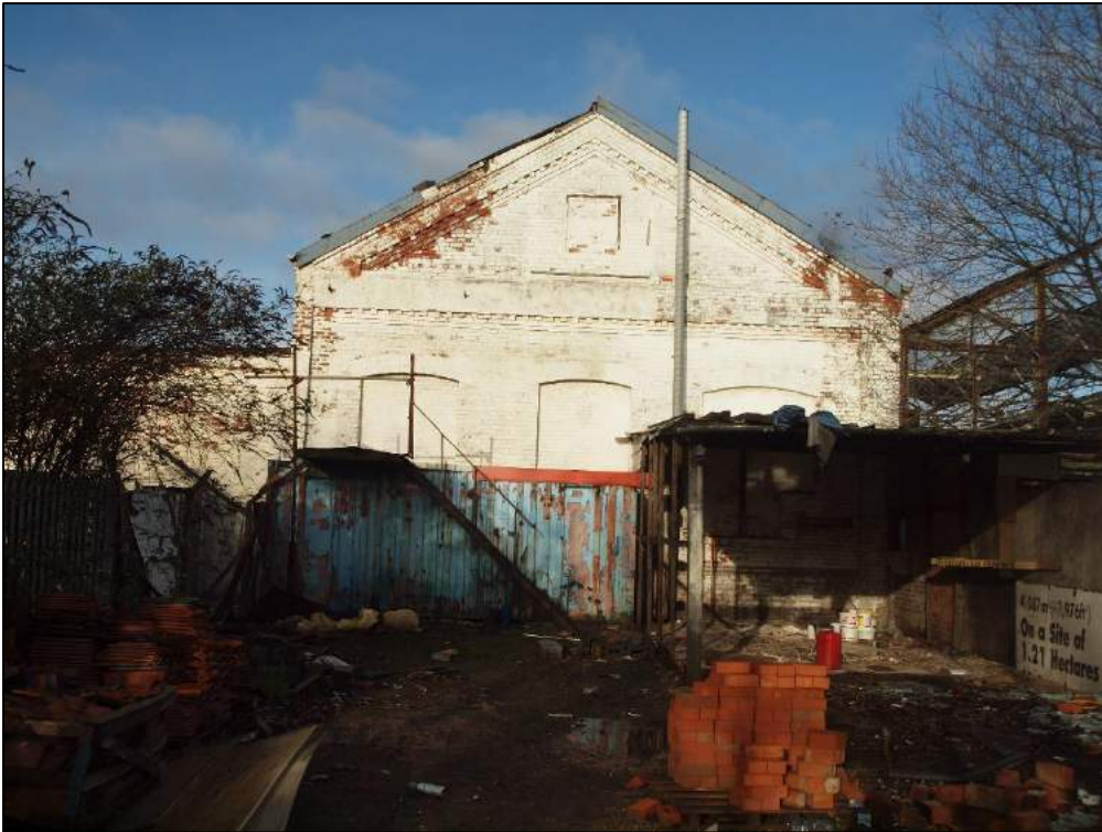
Plate 13: East gable of central building.
