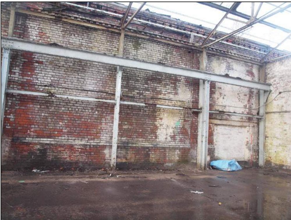
Plate 26: Brick recess with window and inserted loading bay to right.
