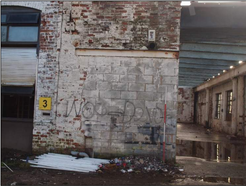
Plate 7: Detail of blocked opening.
