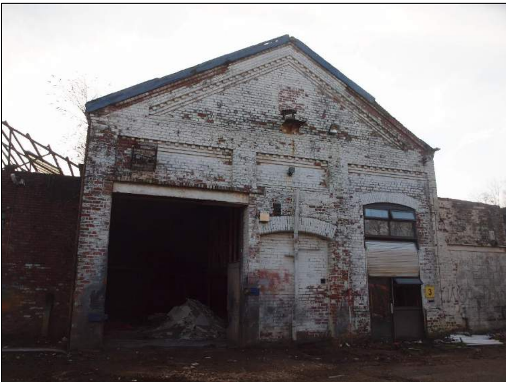
Plate 2: Western gable of central building.
