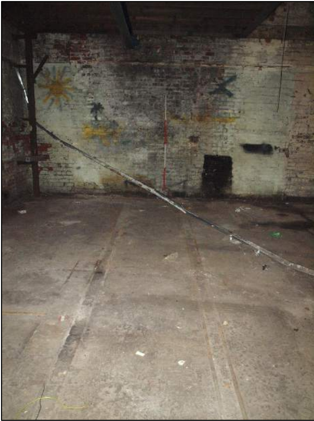
Plate 37: Runners in relation to large blocked opening in south wall.
