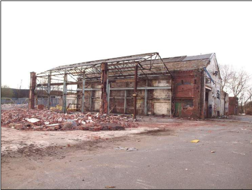
Plate 45: North elevation of original central building.
