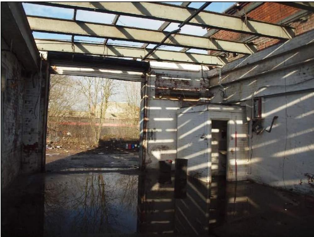
Plate 44: Inserted toilet block to northwest corner.
