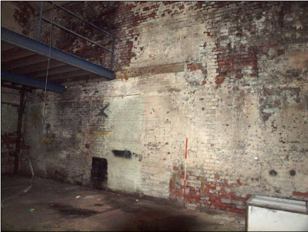
Plate 31: Large blocked opening to east end of southern wall.
