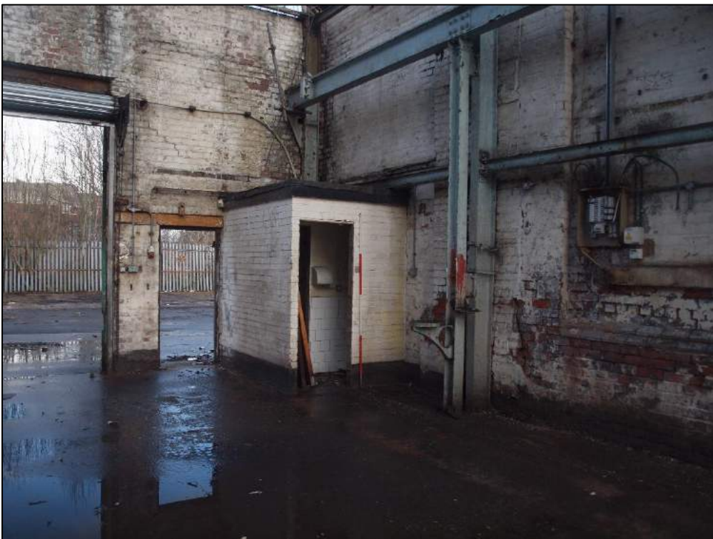
Plate 28: Inserted toilet block to northwest corner.
