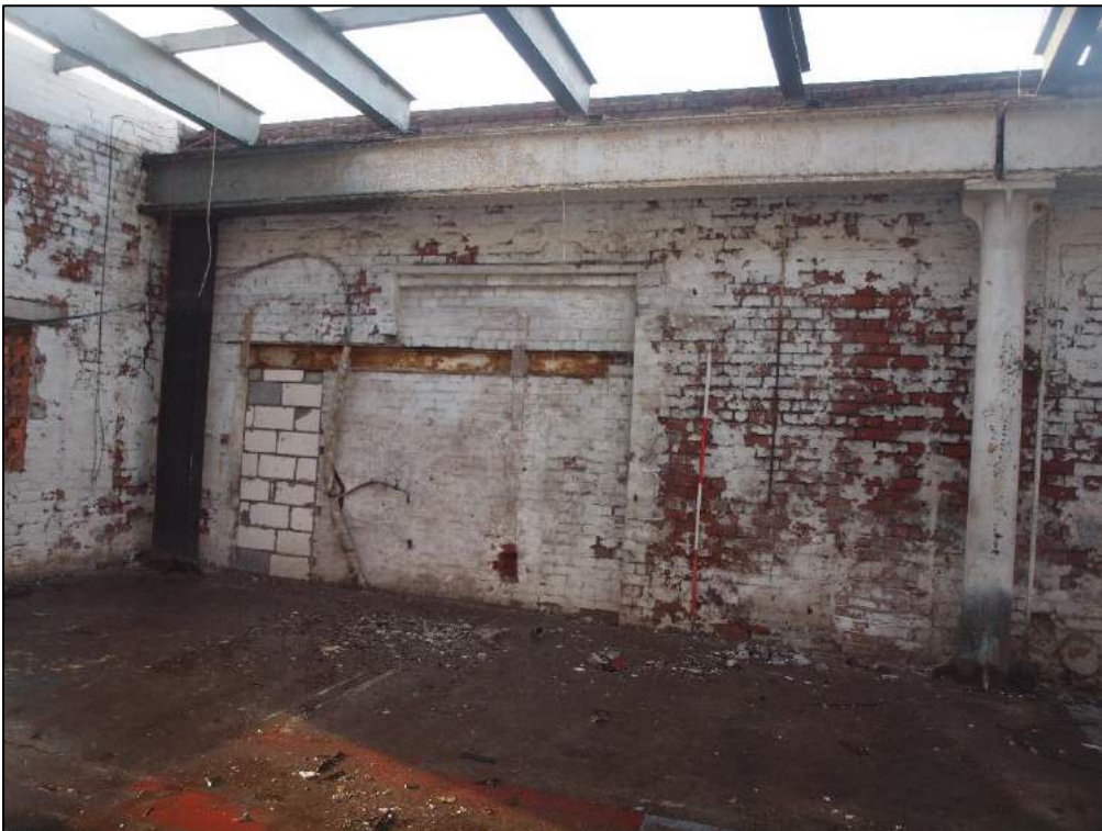
Plate 40: Blocked openings in east end of south wall.
