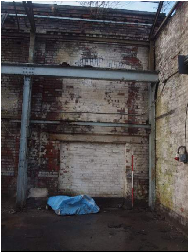
Plate 27: Detail of blocked window with inserted loading door shown above.
