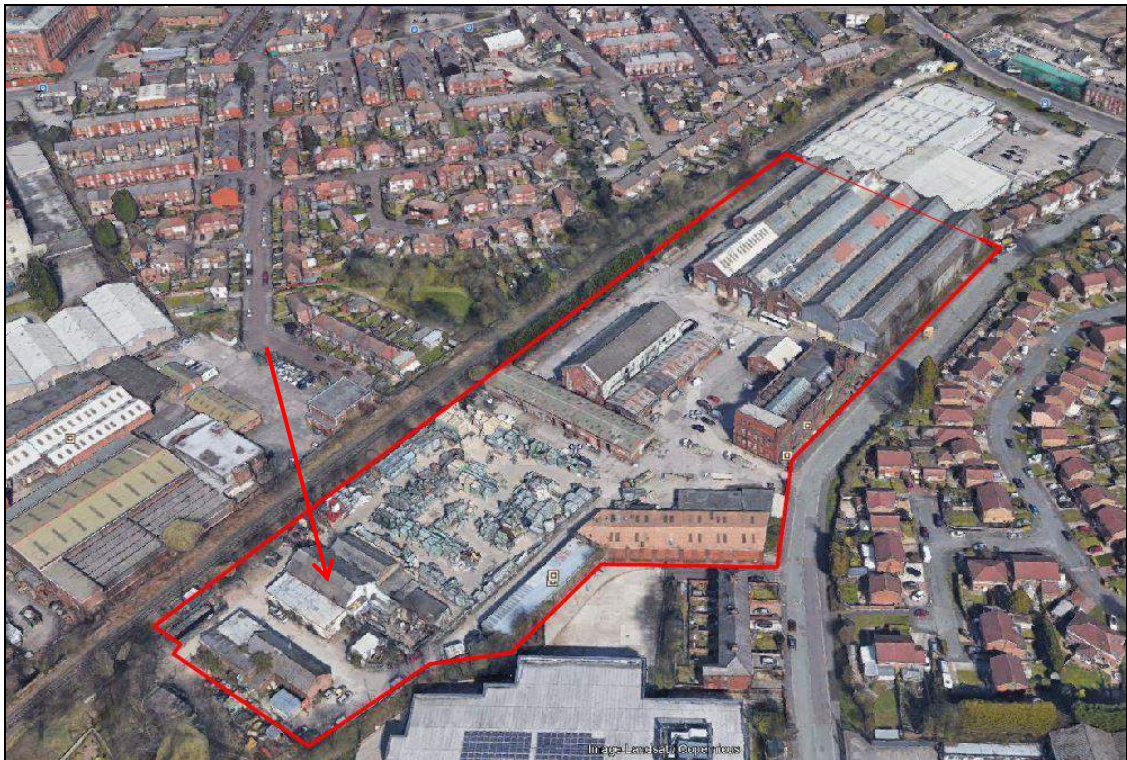
Figure 7: Google earth image showing site with building 3 shown with arrow
