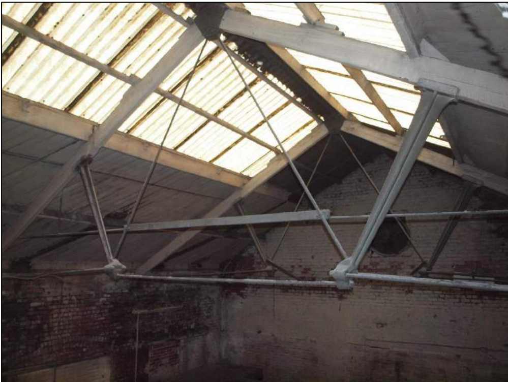
Plate 50: Truss detail of central building.
