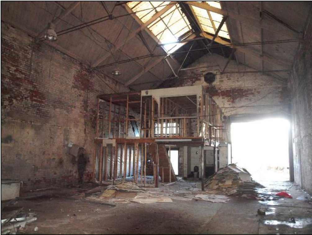
Plate 33: Interior looking west.
