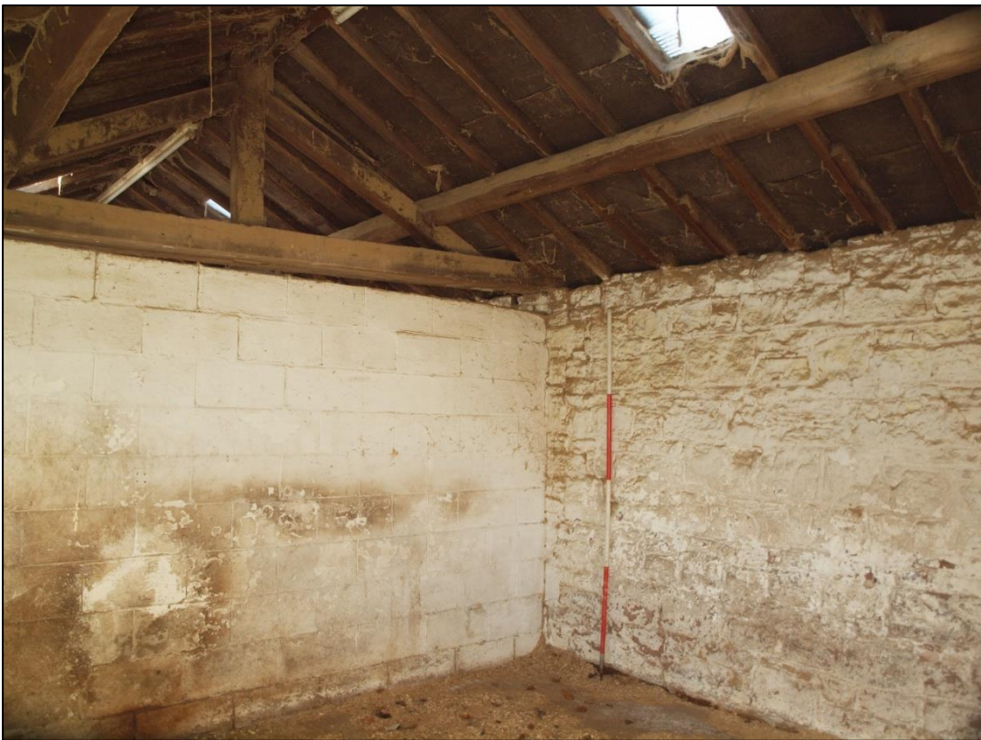
Plate 102: Inserted dividing wall below truss
