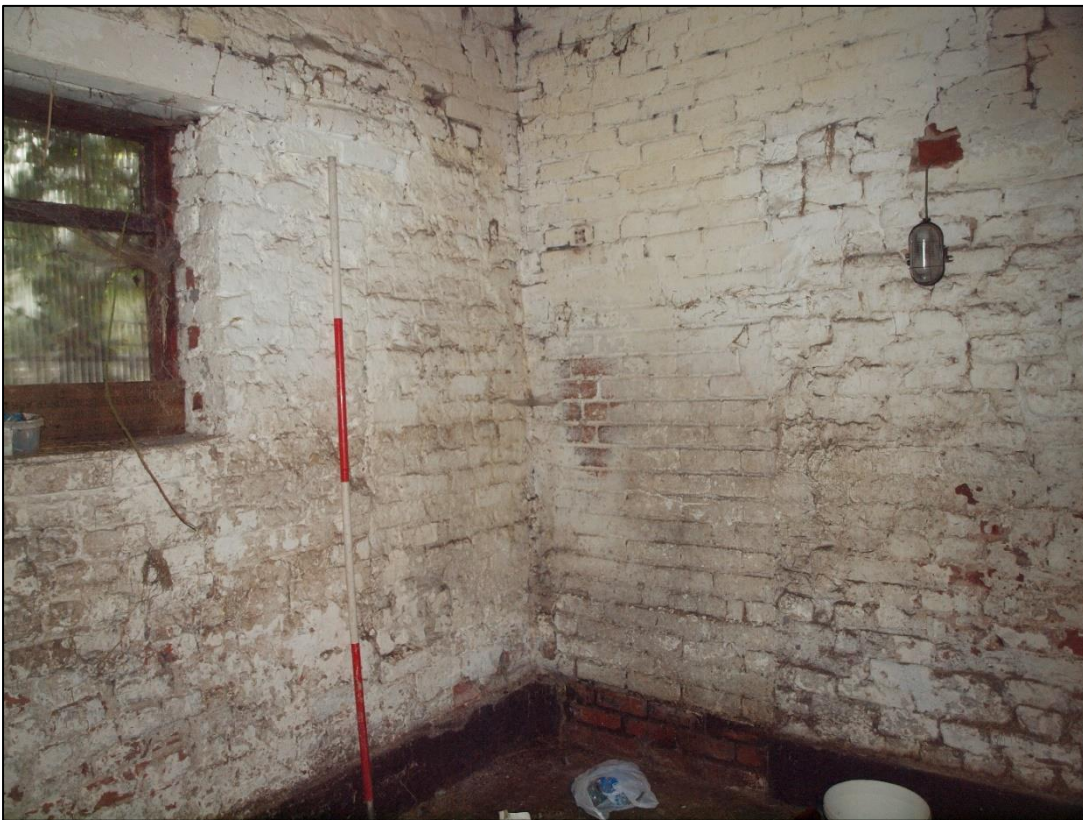
Plate 124: Pair of blocked doorways in southern corner of room
