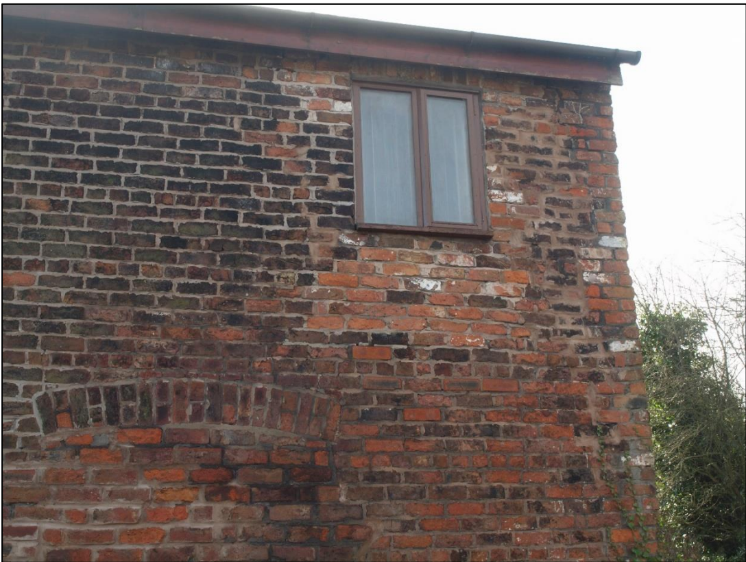
Plate 62: Inserted first floor window
