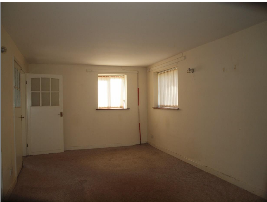
Plate 76: As above looking towards the southeast
