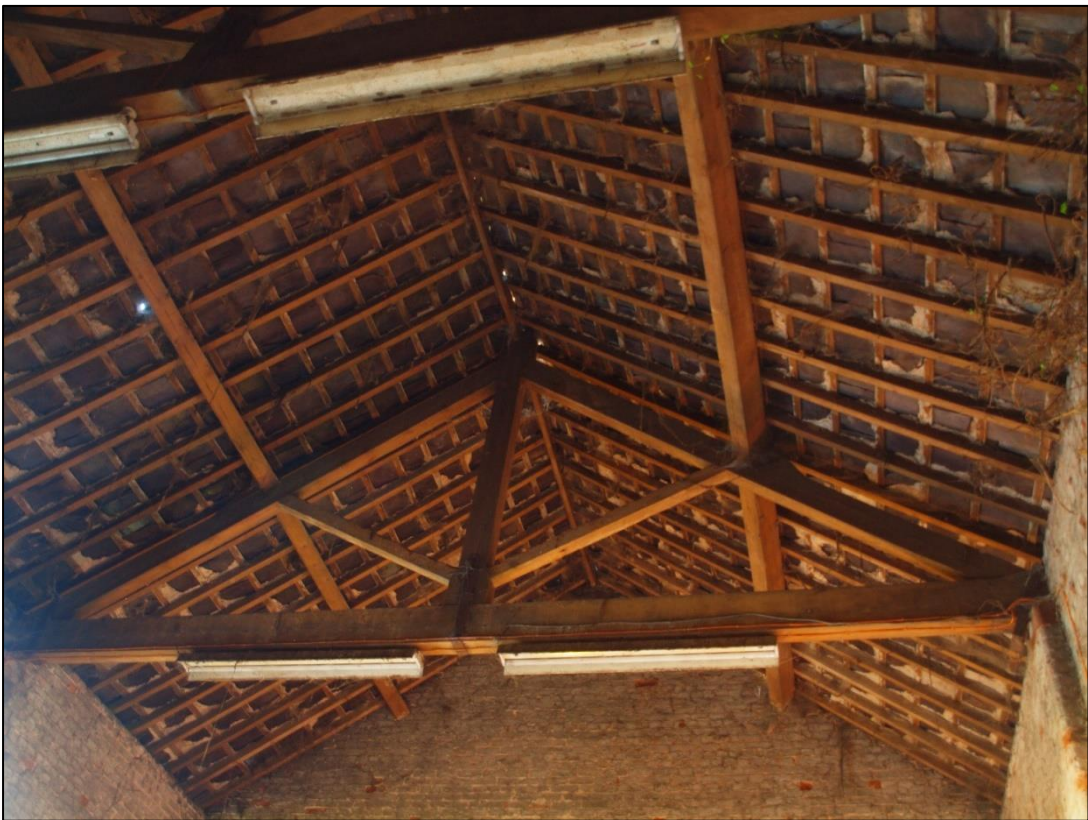
Plate 24: King post truss and roof detail
