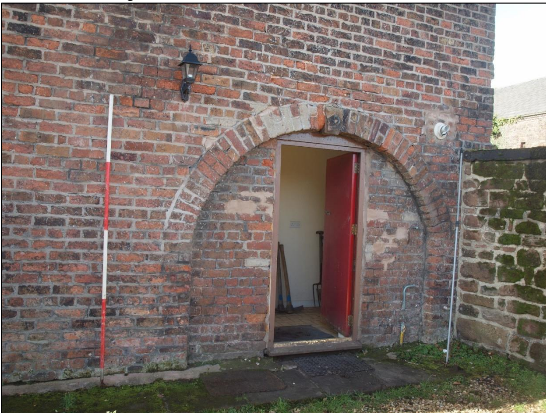
Plate 56: Blocked arched opening with doorway inserted
