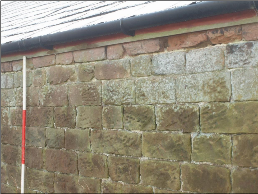
Plate 133: Detail of stonework to northwest elevation
