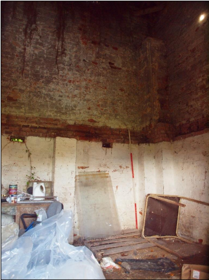
Plate 45: Interior showing brick pillar to ground floor
