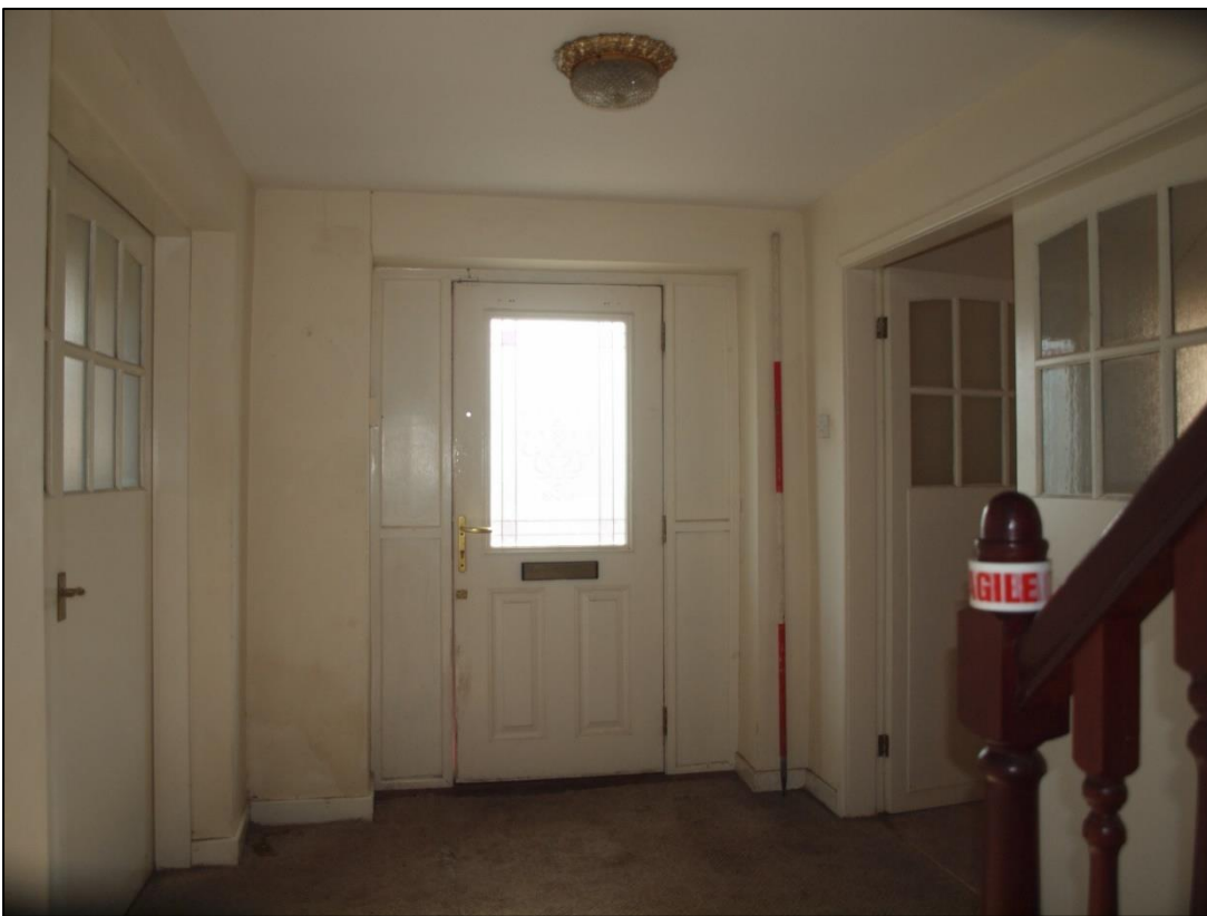
Plate 72: Hallway and staircase showing doorway to southeast elevation
