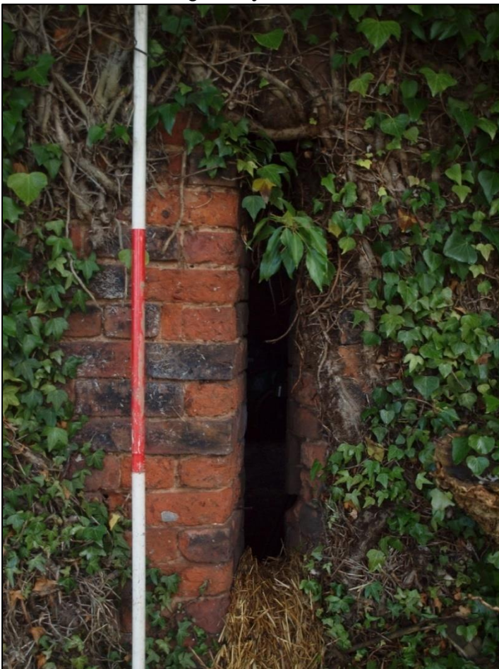
Plate 14: Detail of ventilation slot
