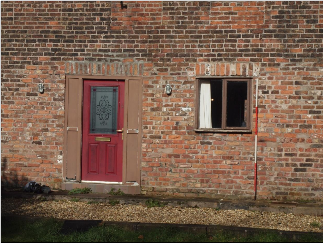
Plate 51: Rebuilt ground floor section of wall
