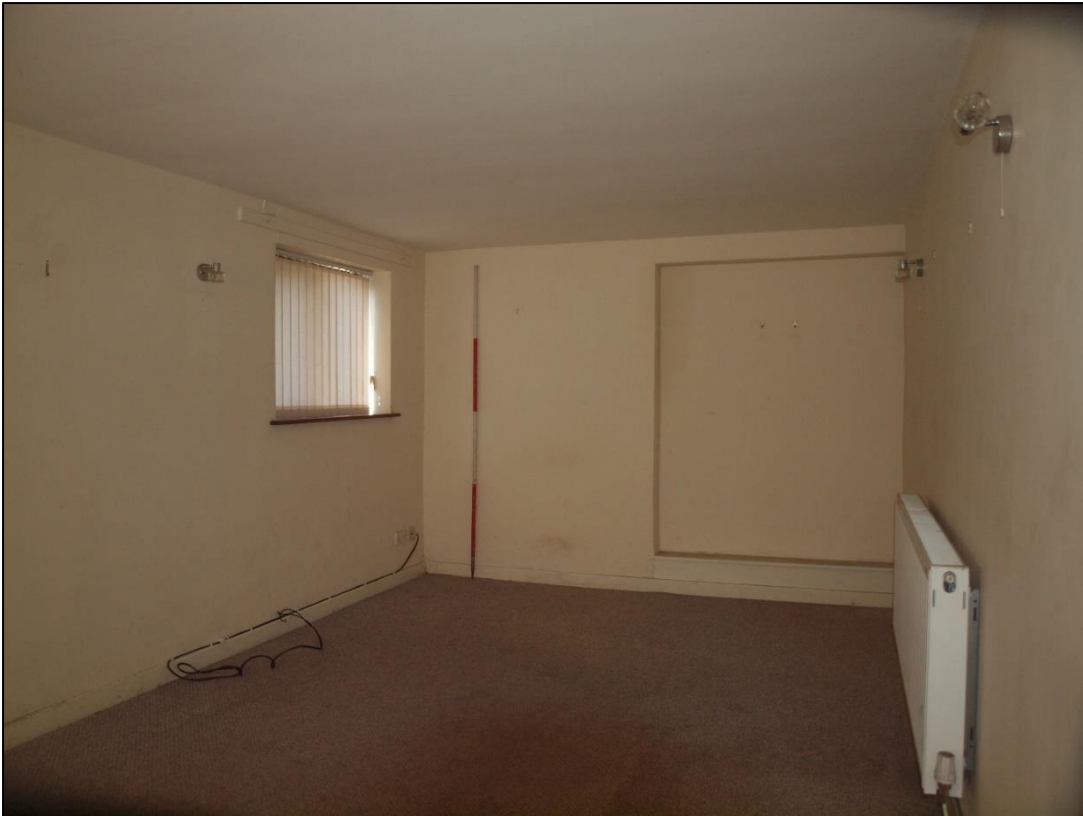
Plate 75: Western room showing recessed blocked opening of former doorway
