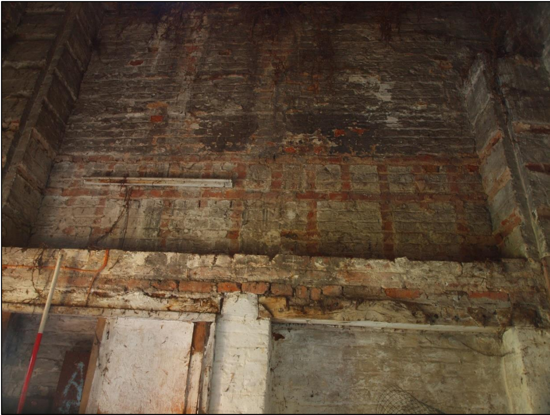
Plate 47: Whitewash showing pattern of removed boxes
