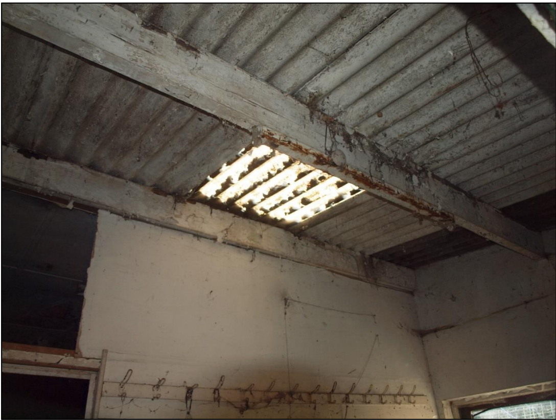
Plate 126: Detail of ceiling
