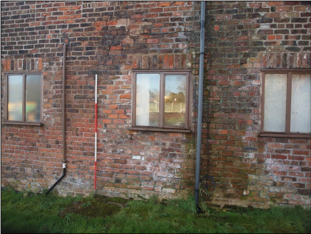
Plate 65: Ground floor windows
