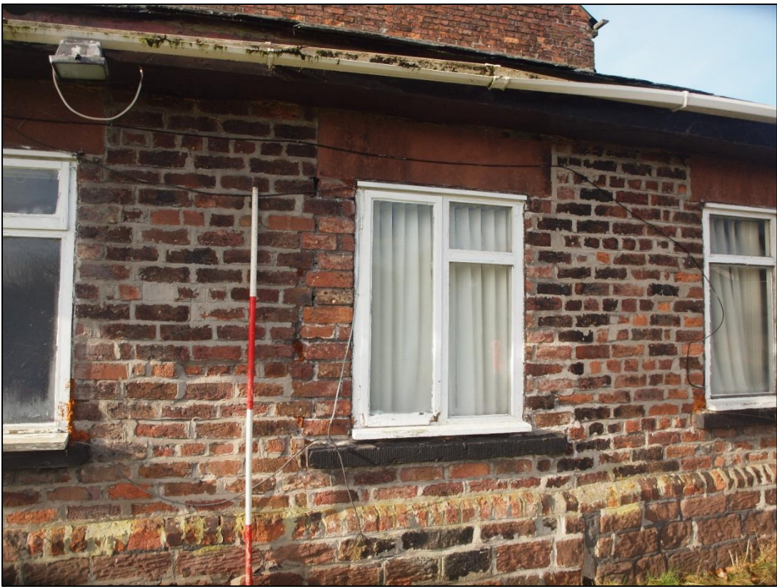
Plate 18: Detail of blocked doorway
