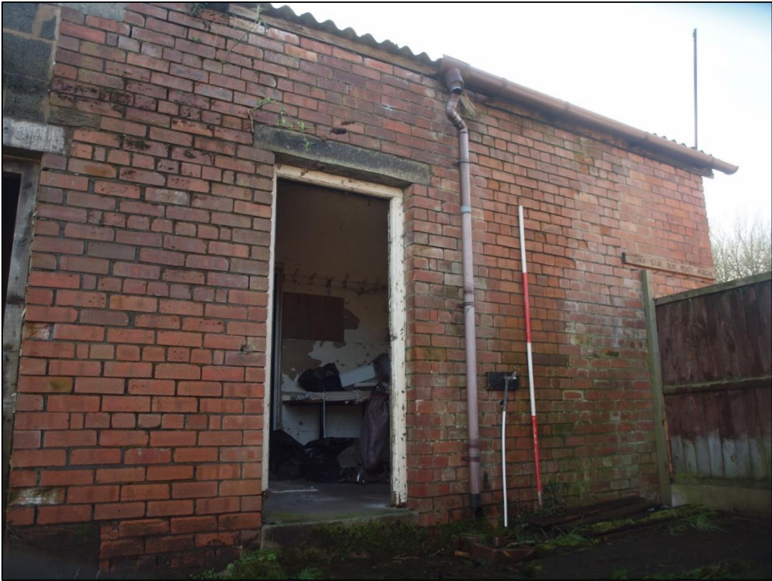
Plate 109: Western end constructed of modern brick
