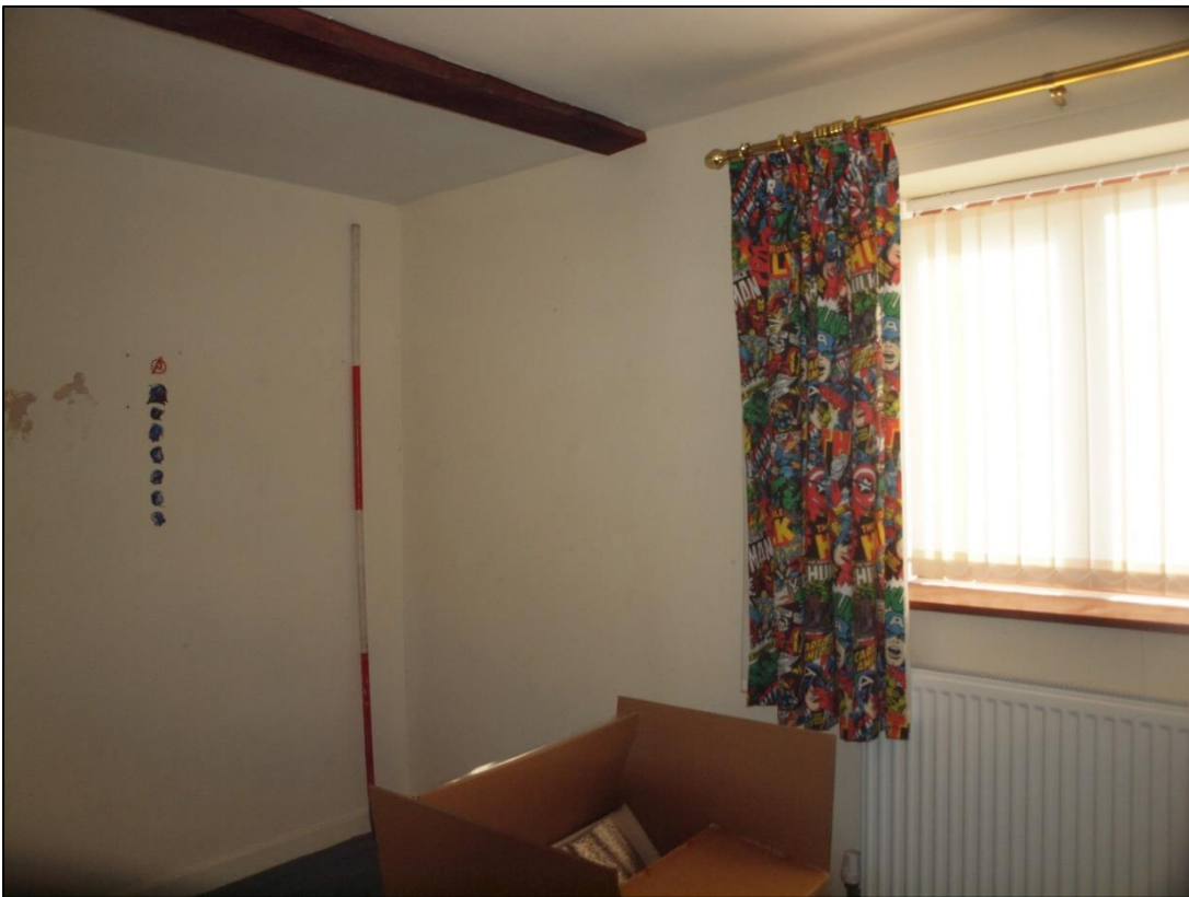
Plate 82: Room to south side of corridor showing base of truss
