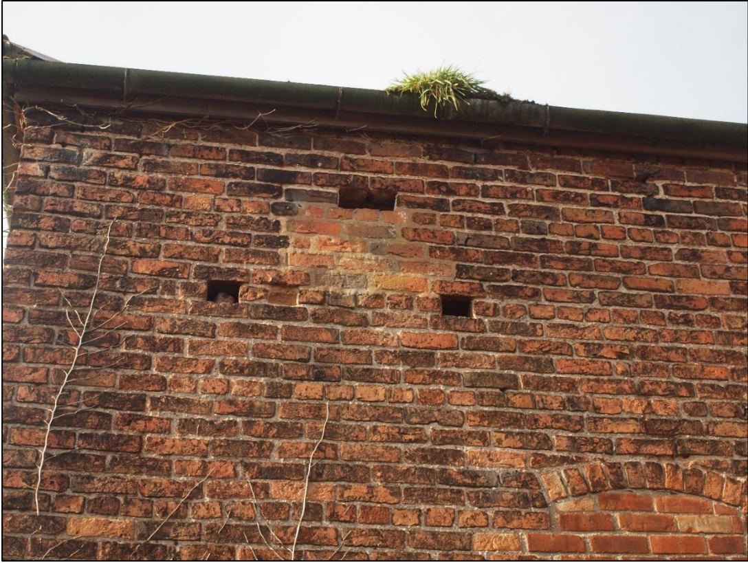
Plate 39: Blocked opening high in the face
