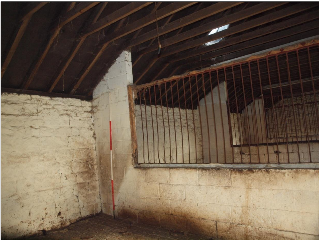
Plate 136: Interior showing inserted cross walls
