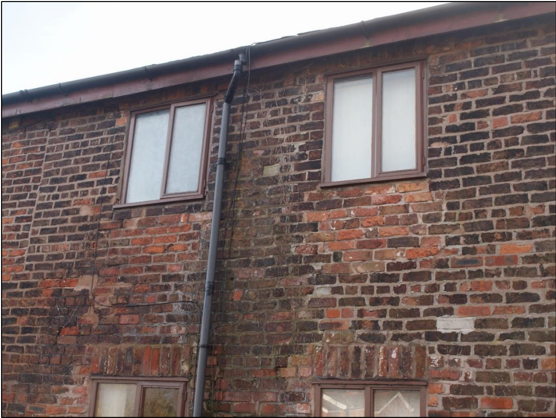
Plate 63: Inserted first floor windows
