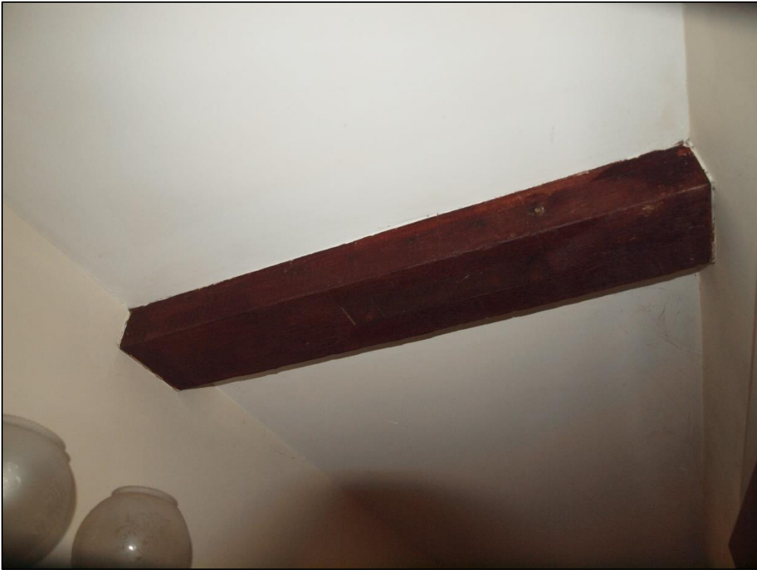
Plate 87: Base of truss visible in corridor
