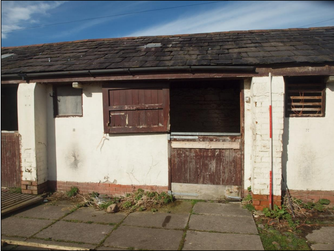
Plate 91: Inserted wall, brick piers and doorway detail
