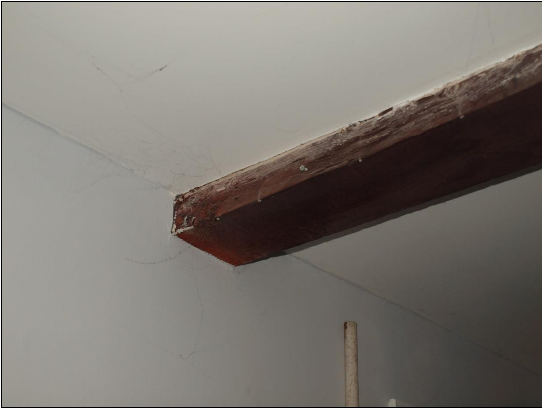
Plate 81: Base of truss detail
