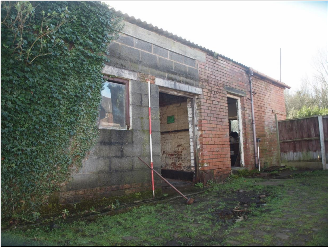
Plate 107: Central section built in concrete block
