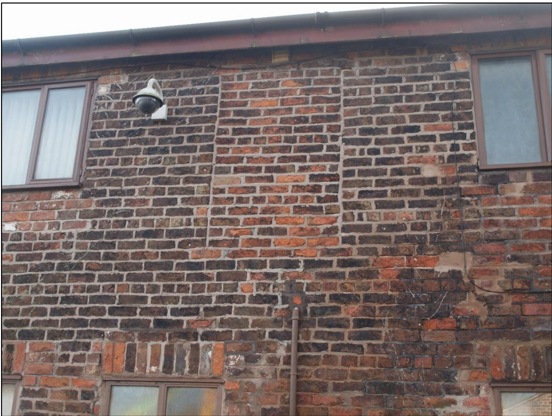
Plate 64: Blocked window detail
