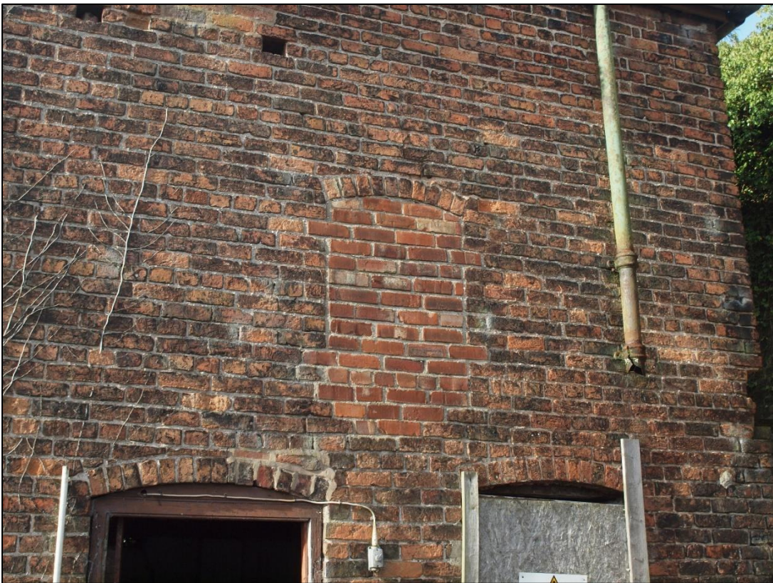
Plate 38: Blocked window at first floor level
