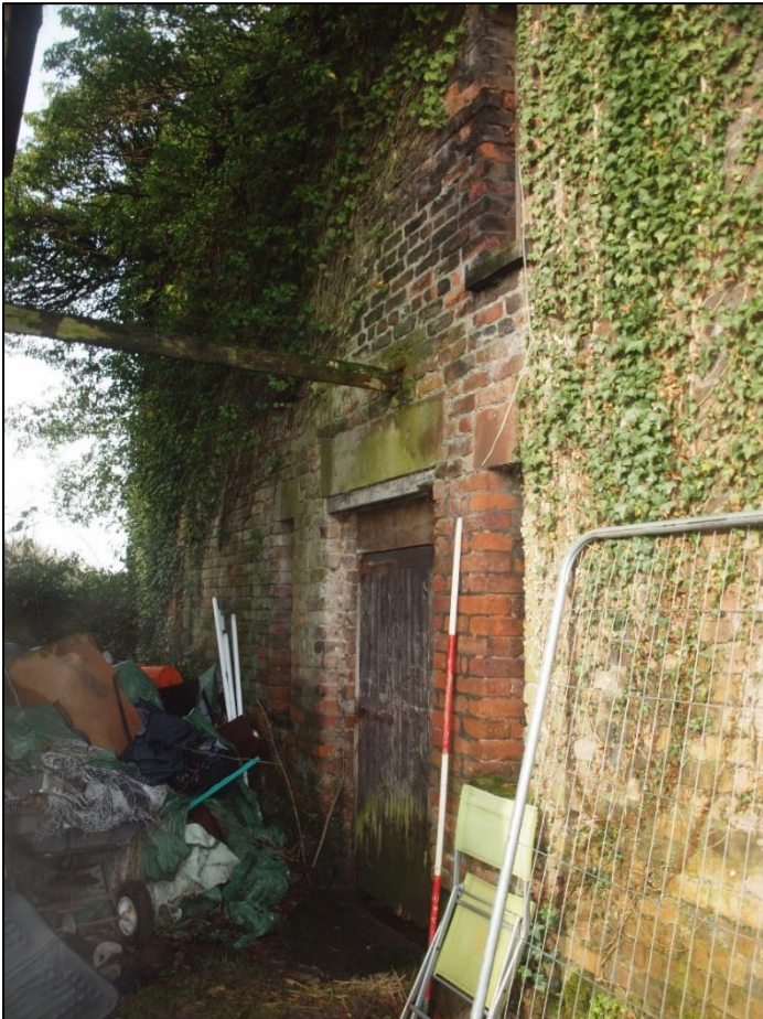
Plate 16: As above showing winnowing doorway
