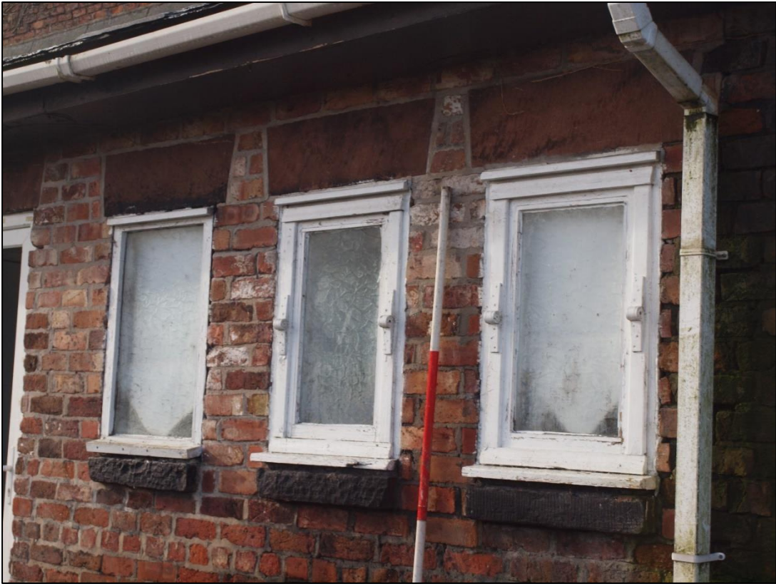
Plate 21: Inserted windows detail
