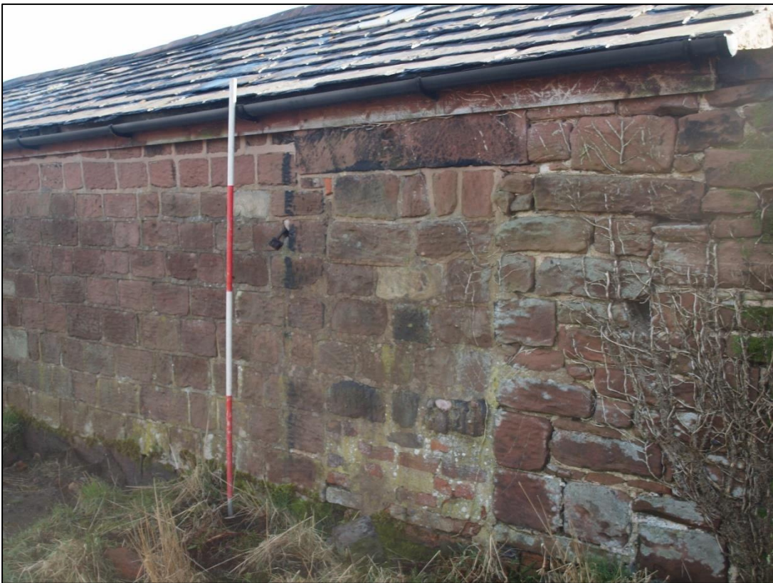
Plate 96: Blocked doorway detail
