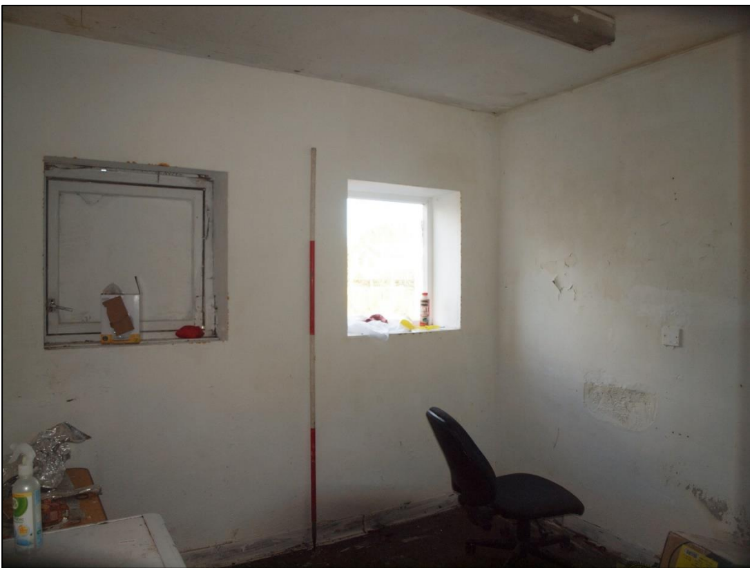
Plate 30: Room to east of barn door
