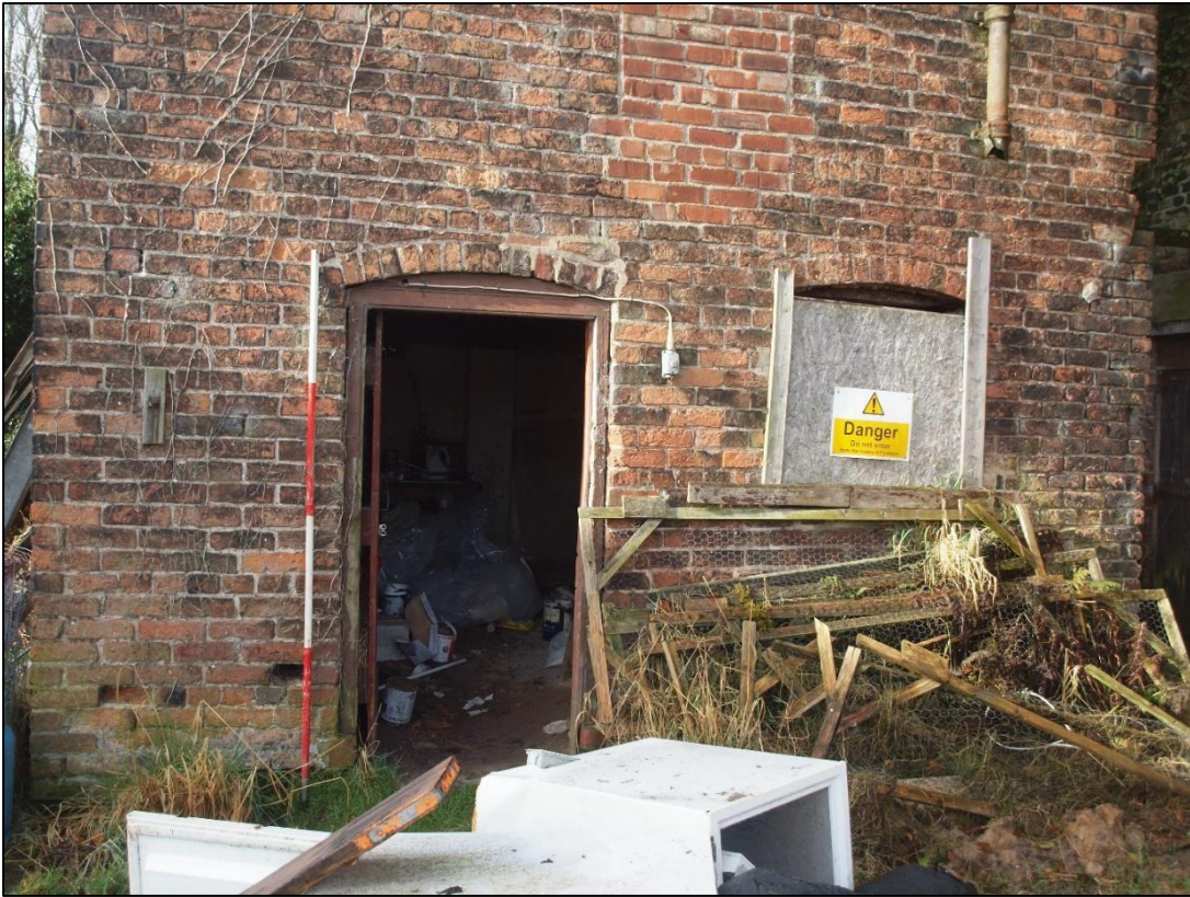
Plate 37: Detail of ground floor of northeast elevation
