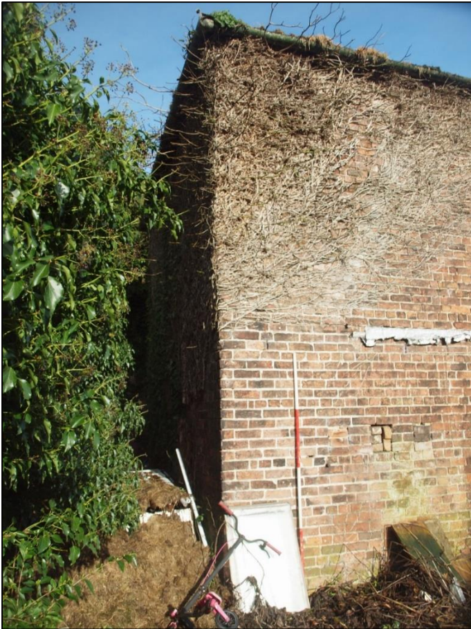
Plate 42: Southeast and southwest elevations
