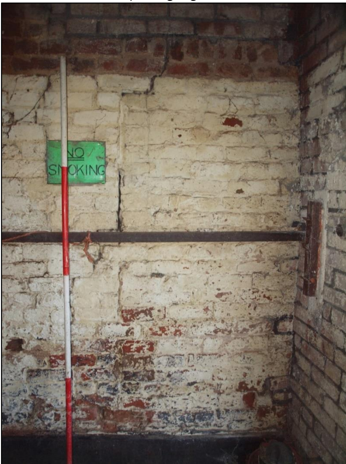
Plate 122: Blocked doorway directly below above
