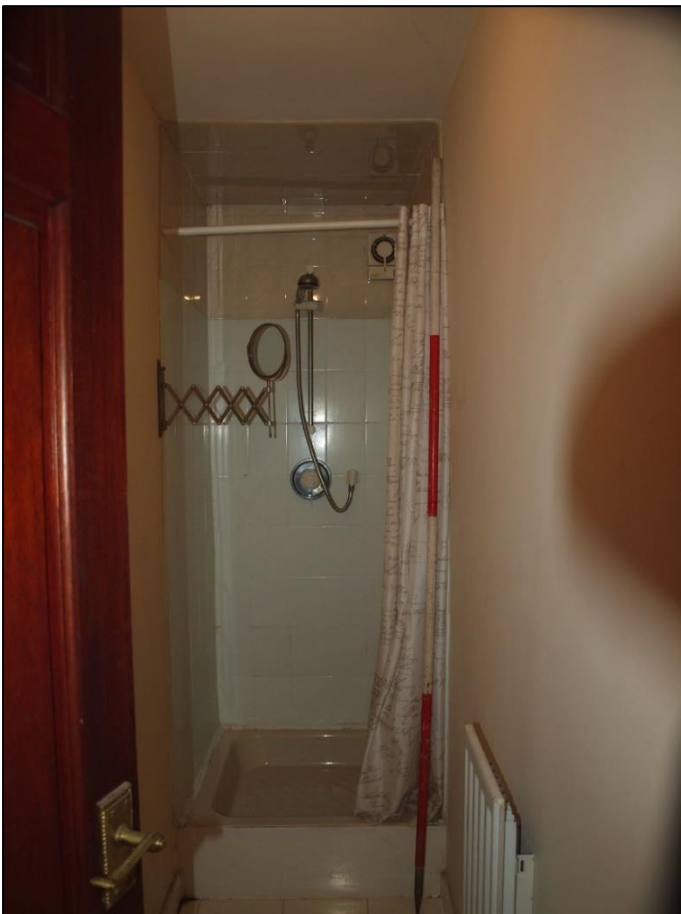
Plate 84: Inserted shower room
