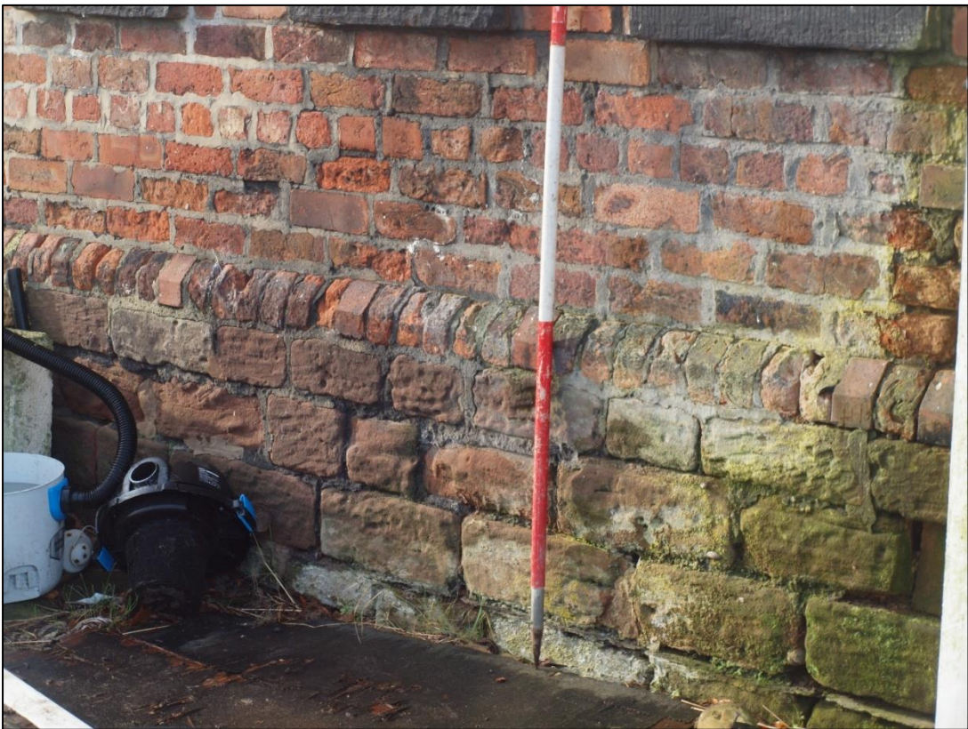
Plate 20: Stone and brick plinth detail
