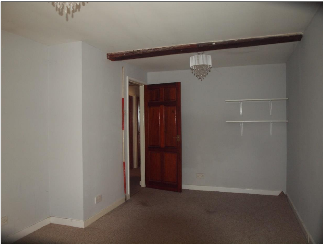
Plate 80: As above showing base of truss
