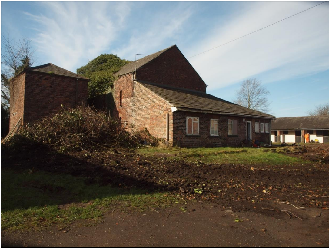
Plate 1: General shot showing (left to right) Buildings 2, 1 and 6
