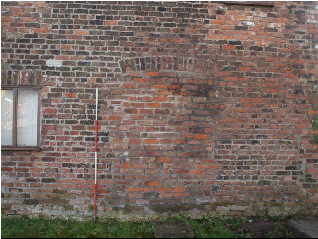
Plate 61: Blocked doorway detail
