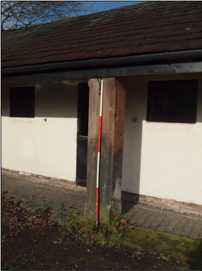
Plate 129: Detail of sandstone pier
