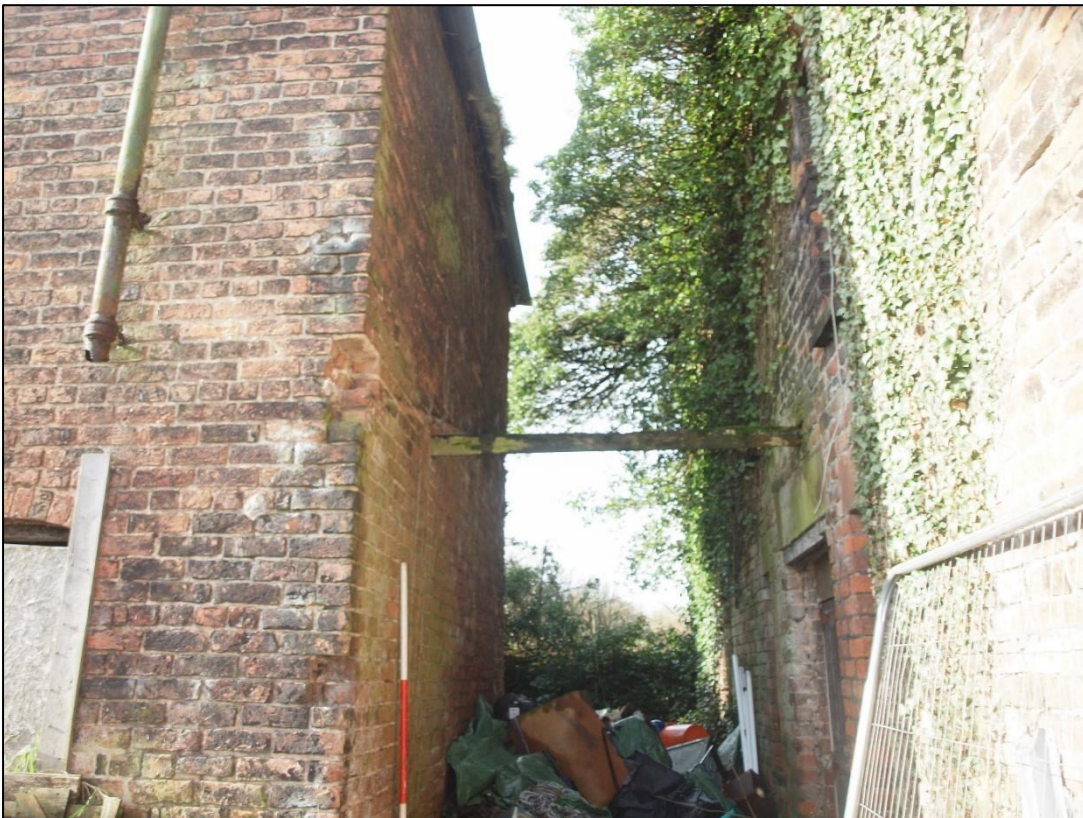
Plate 44: Relationship between building 1 and 2
