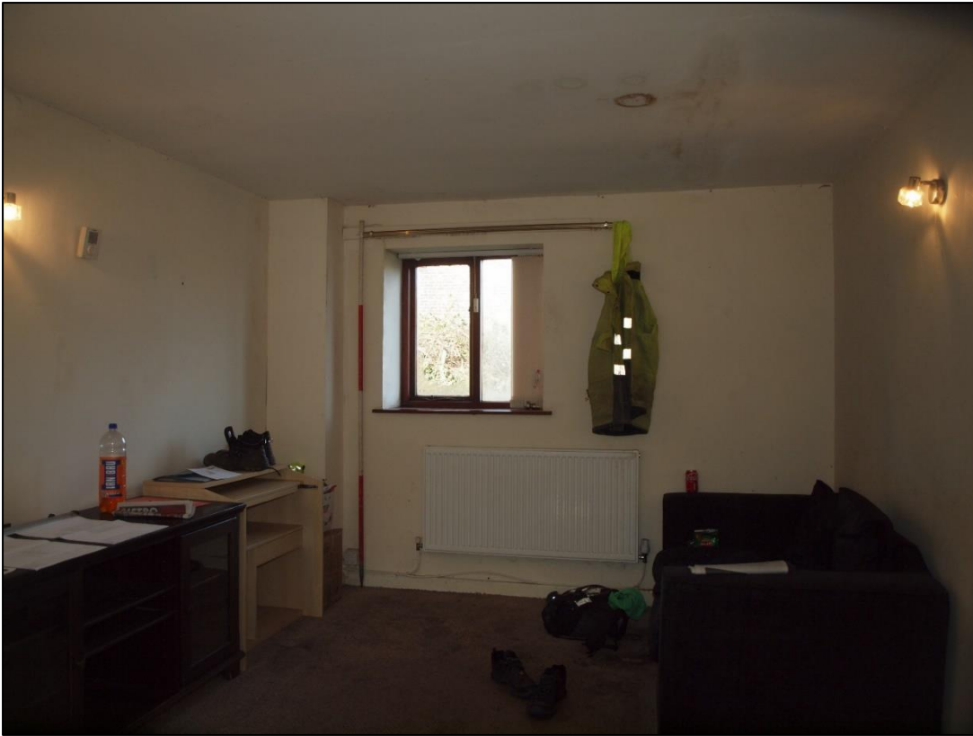
Plate 69: Room to the west of kitchen
