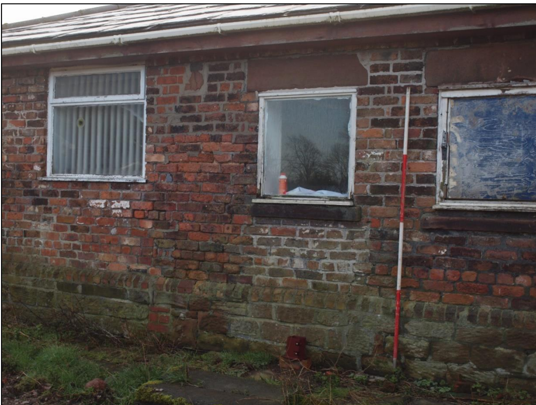
Plate 4: Blocked doorway detail
