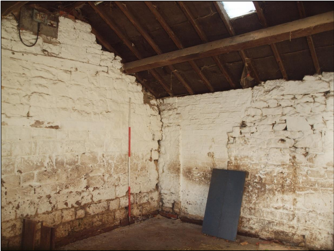
Plate 99: Interior showing blocked doorway in northwest elevation
