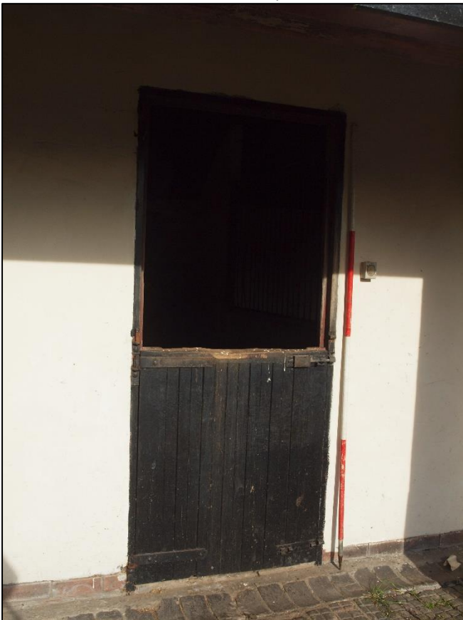
Plate 130: Doorway in inserted wall detail
