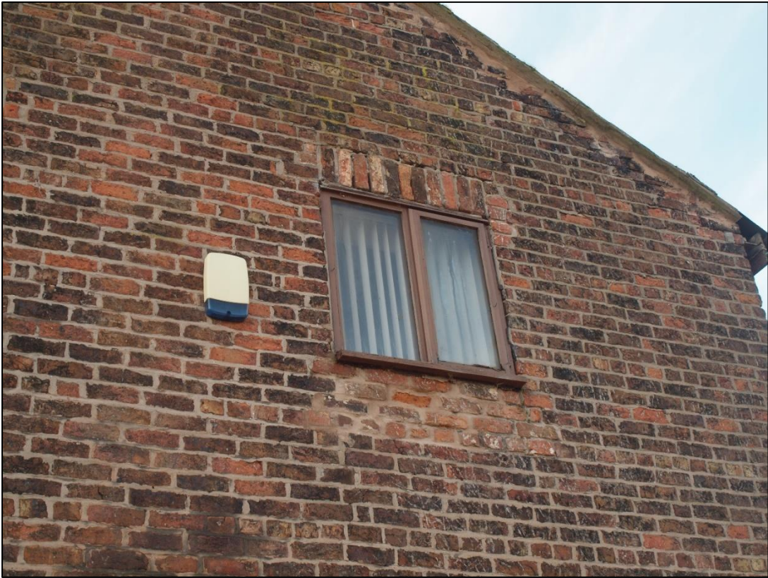
Plate 57: Inserted first floor window
