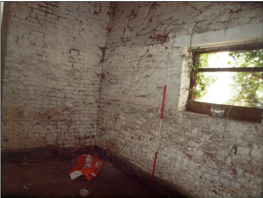
Plate 118: Blocked doorway in east end of southeast wall
