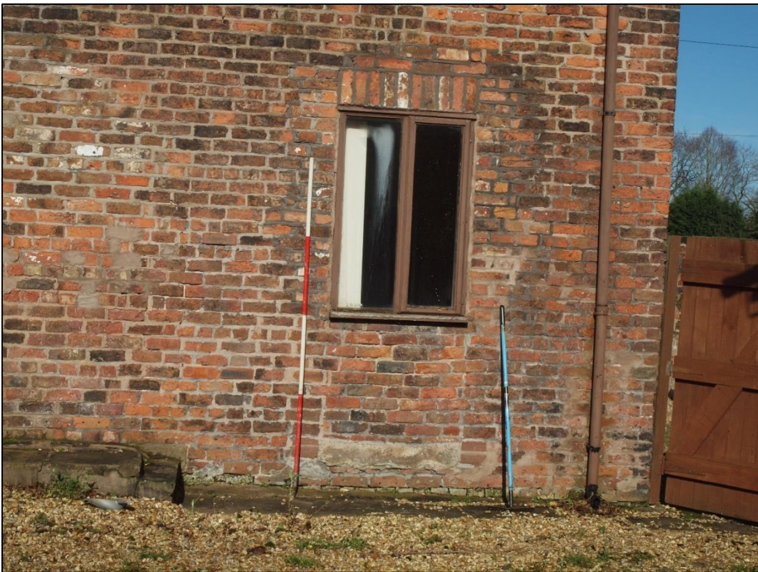
Plate 54: Blocked doorway with window inserted
