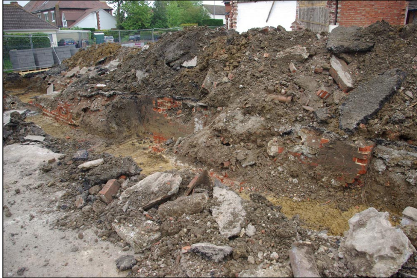
Figure 7 The brick foundations, looking north-west.
