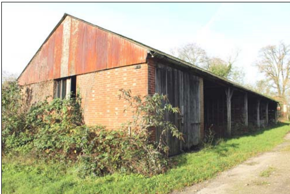
Figure 4 The barn from the south-west
