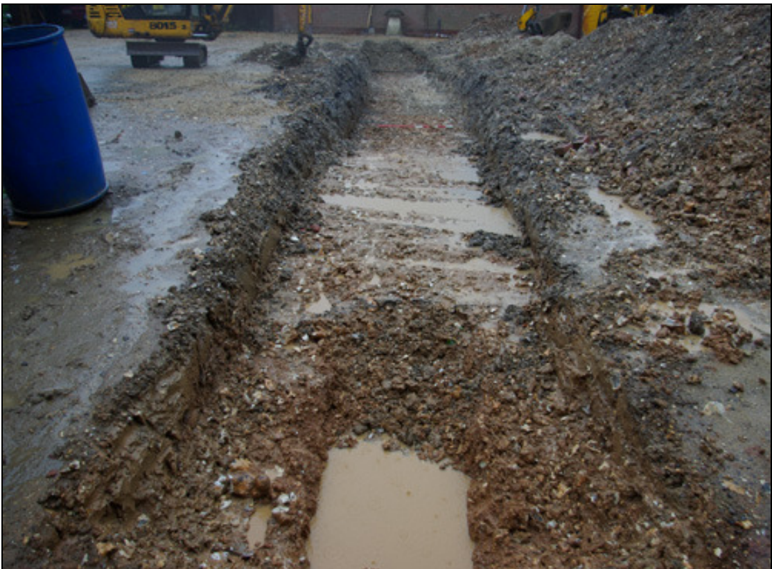
Figure 5 The evaluation trench looking south.
