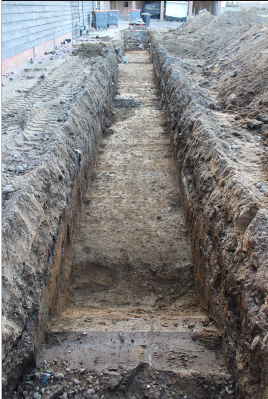
Figure 5 Trench 2, looking west
