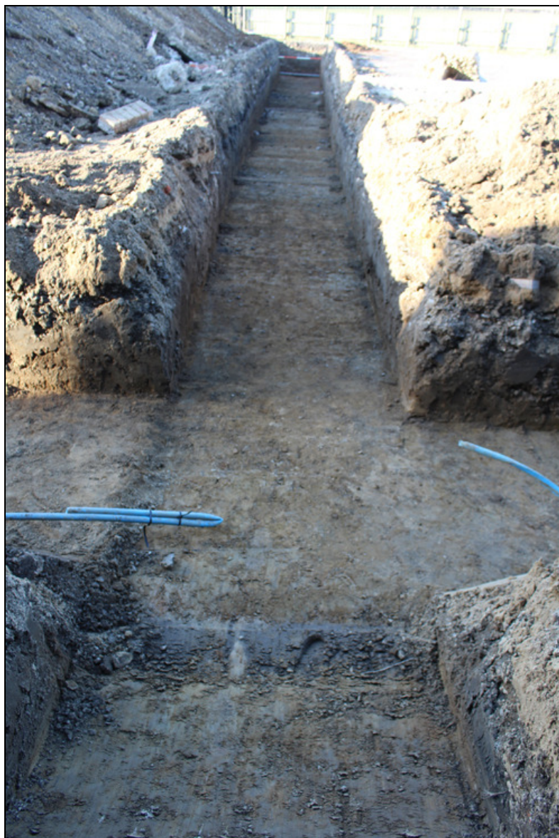
Figure 4 Trench 1, looking north
