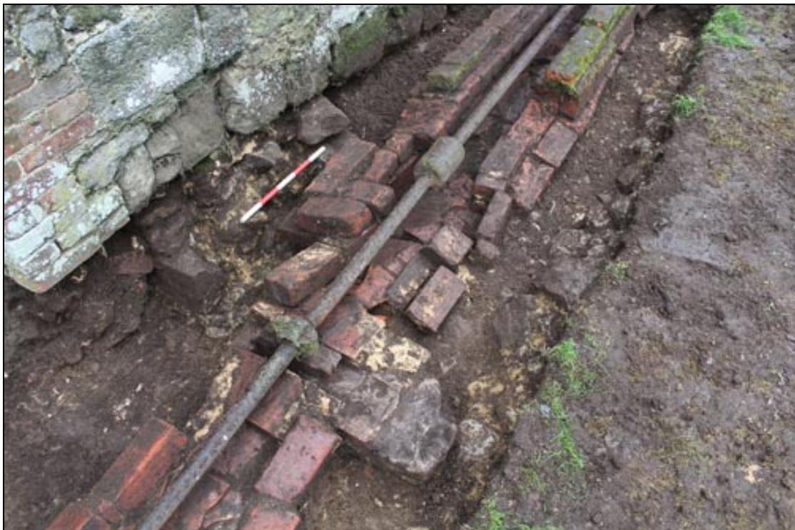
Figure 33 Trench 18, Foundations 51 (under the scale) & 81 (against the right baulk of the trench), looking north-west
