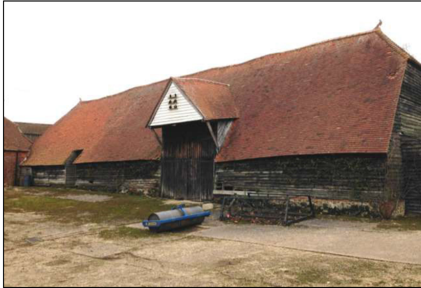
Figure 46 The threshing barn before works, looking north-east
