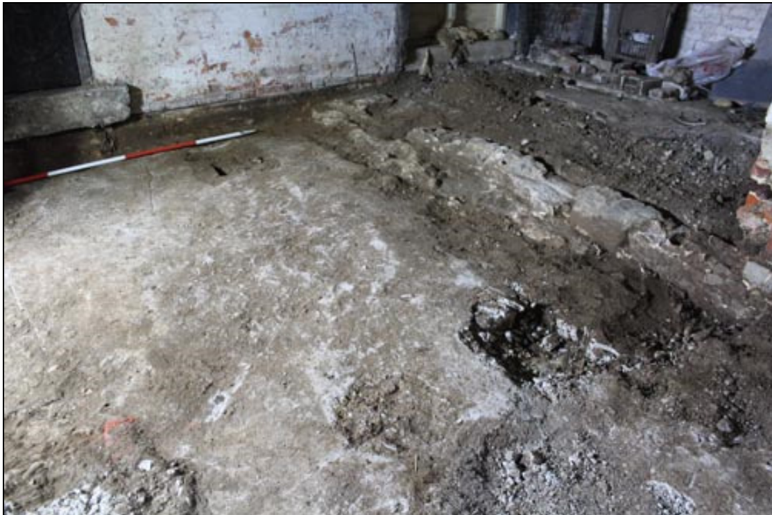
Figure 60 The surviving section of the north aisle foundations at its north-west corner, with the late 19 th century cowshed behind, looking north-west
