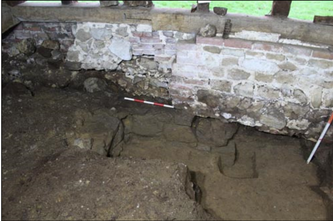
Figure 25 Trench 7, Foundations 26 & 28, looking east
