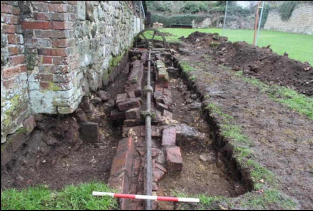
Figure 58 Trench 18, the external drive shaft (80), looking north
