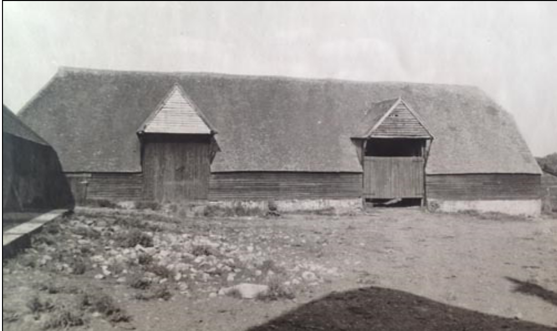
Figure 61 The west side of the barn before the removal of the north door, taken in the 1940's (Historic England Archive)
