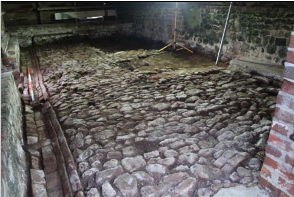
Figure 59 The floor of the lean-to, looking north-west
