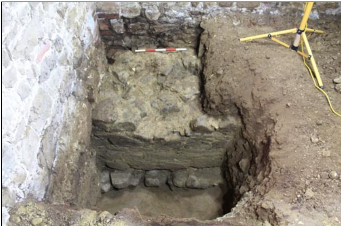
Figure 32 Trench 10, Foundation 15, looking south
