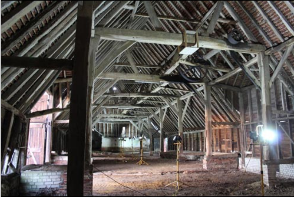
Figure 54 The interior of the barn, looking north. The two cast iron wheels can be seen in the roof space to the right, over the southern threshing bay
