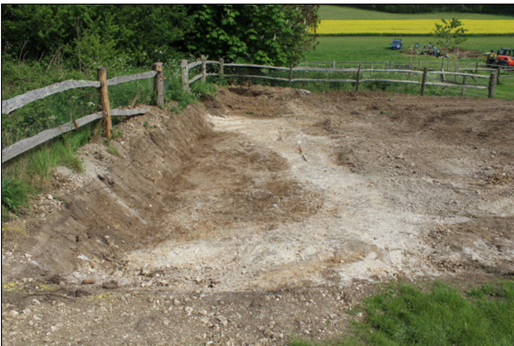
Figure 5 The two pits [26 & 28] within the Summer House watching brief trench, looking east
