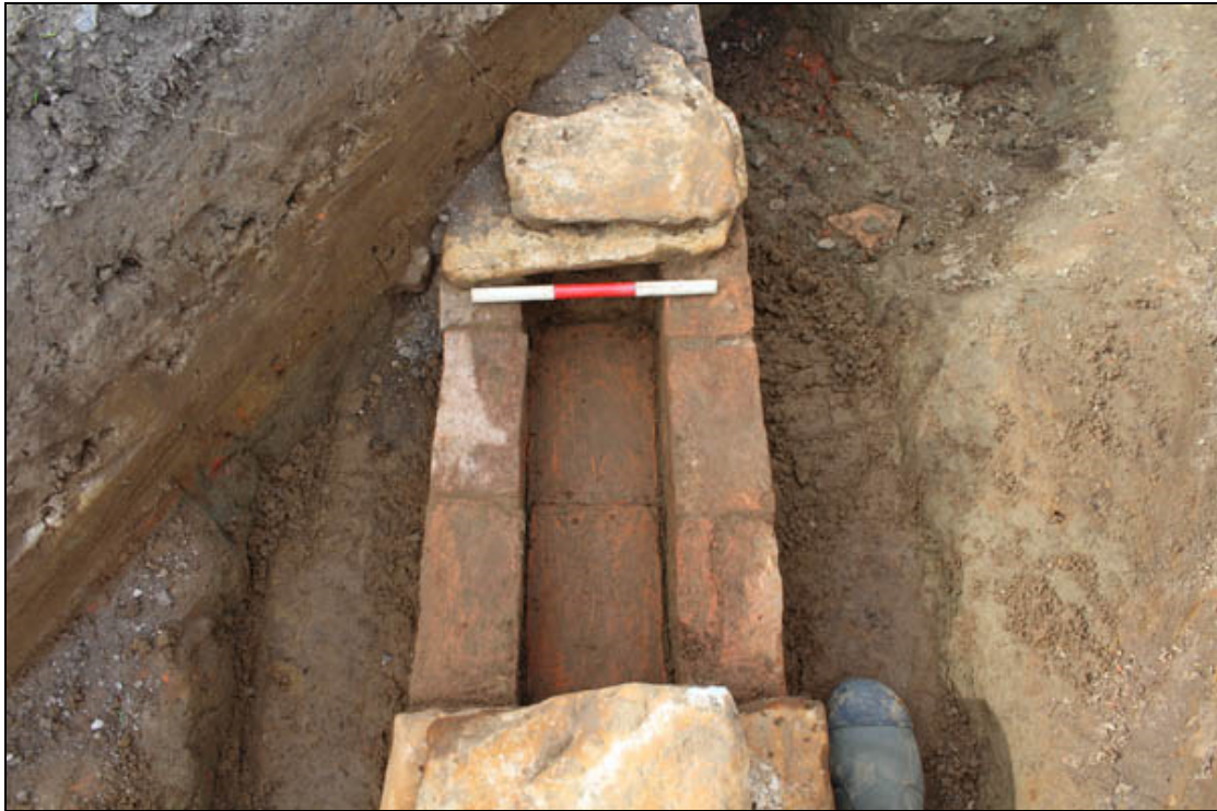
Figure 12 Detail of the brick and stone culvert in Trench 2, after the capping stones have been removed, looking north-west
