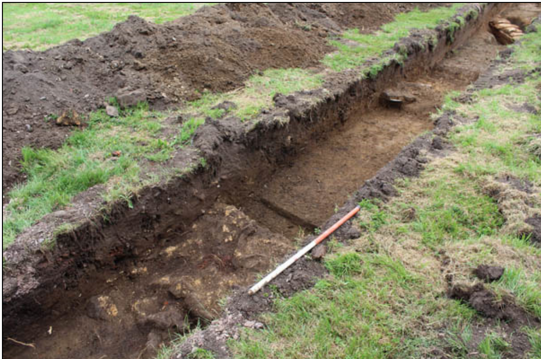
Figure 9 The wall foundation (1), the spread of stones and mortar (4) and the brick and stone culvert (8) in Trench 2
