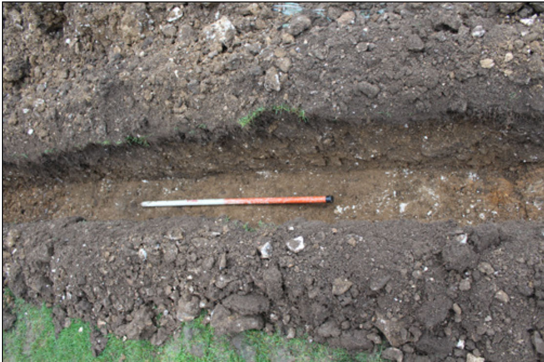
Figure 5 The pit/ditch within the water pipe trench, looking south-west. The 1m scale lies over
