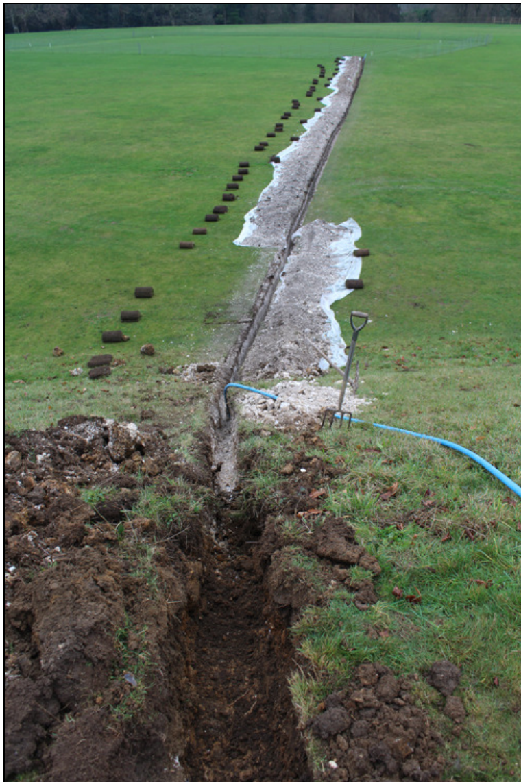
Figure 2 South end of the new water pipe trench, looking south
