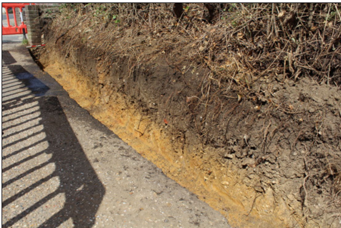
Figure 4 The excavated trench, looking west
