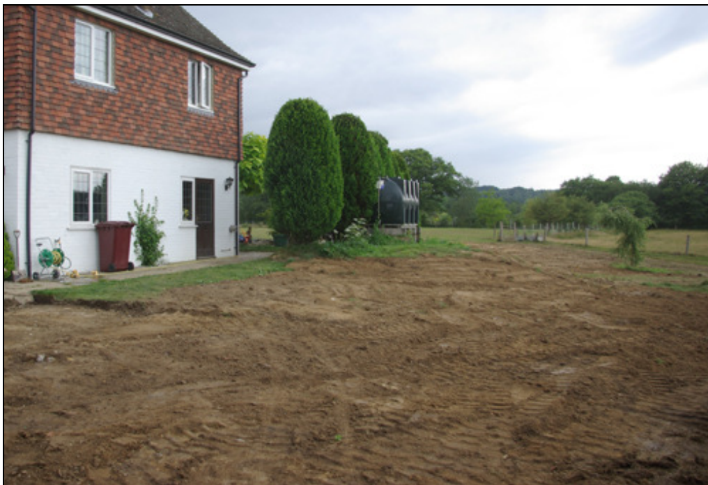
Figure 5 Area 1 after grading, looking west
