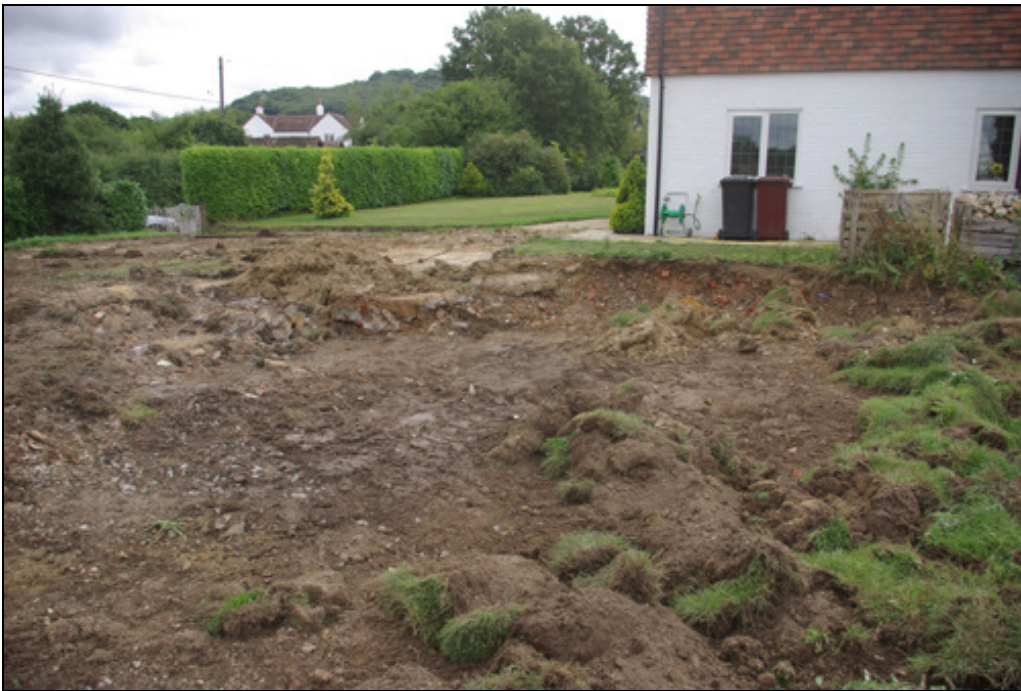
Figure 4 Area 1 after the removal of modern building rubble, looking south
