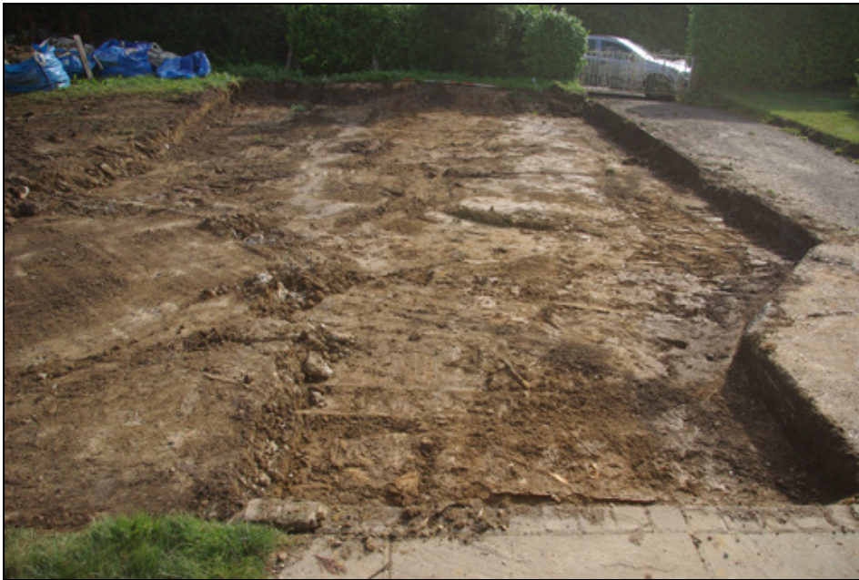
Figure 6 Area 2, looking east
