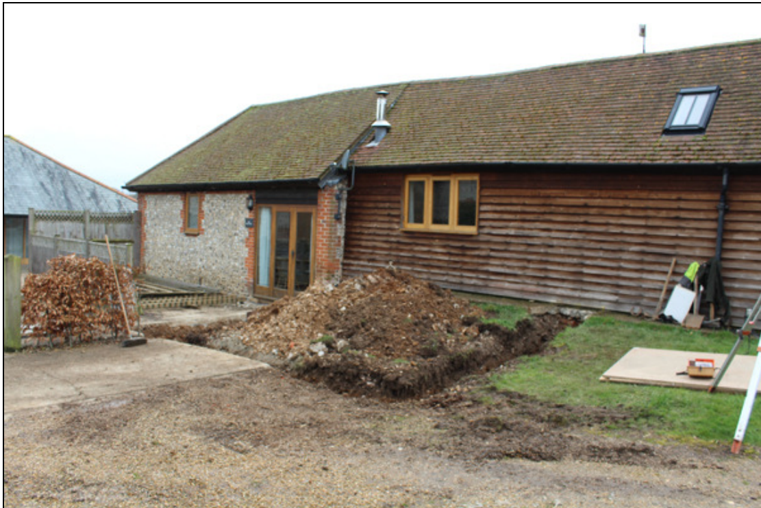
Figure 4 The excavated trench, looking south-west
