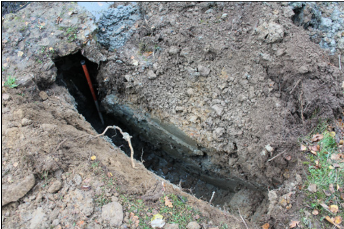
Figure 5 The western trench, looking south-west
