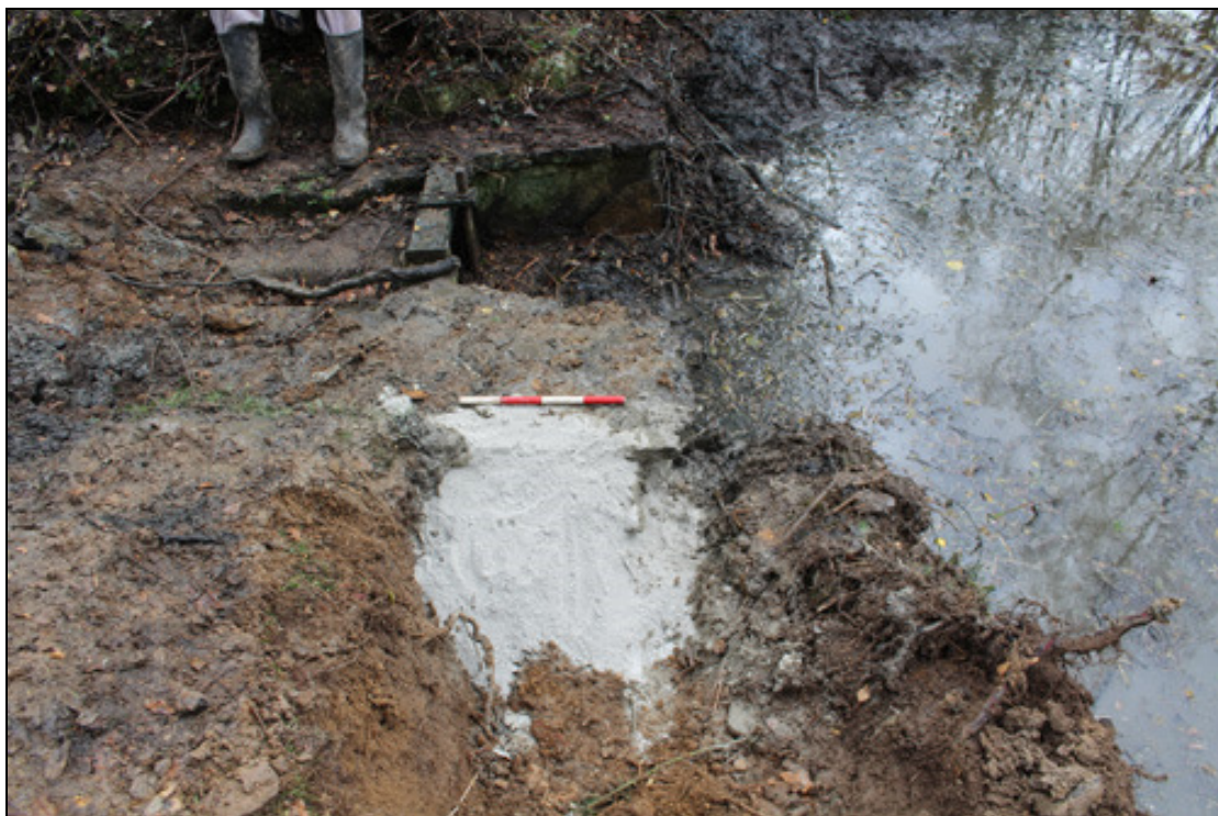
Figure 6 The western trench after sealing and backfilling, looking south towards the sluice
