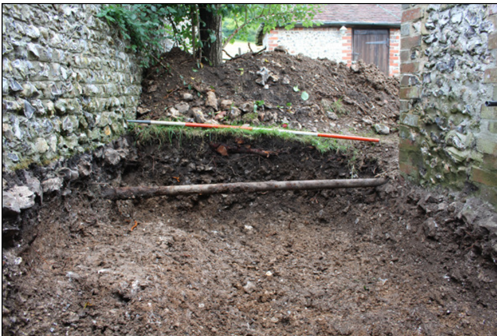
Figure 5 The east face of the Investigation trench, showing the flint retaining wall to the left
