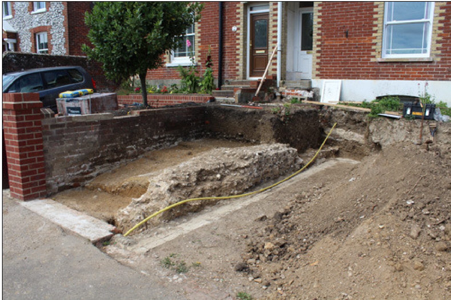
Figure 9 The wall foundation (8) of the Flavian Palace's west wing, looking north-west
