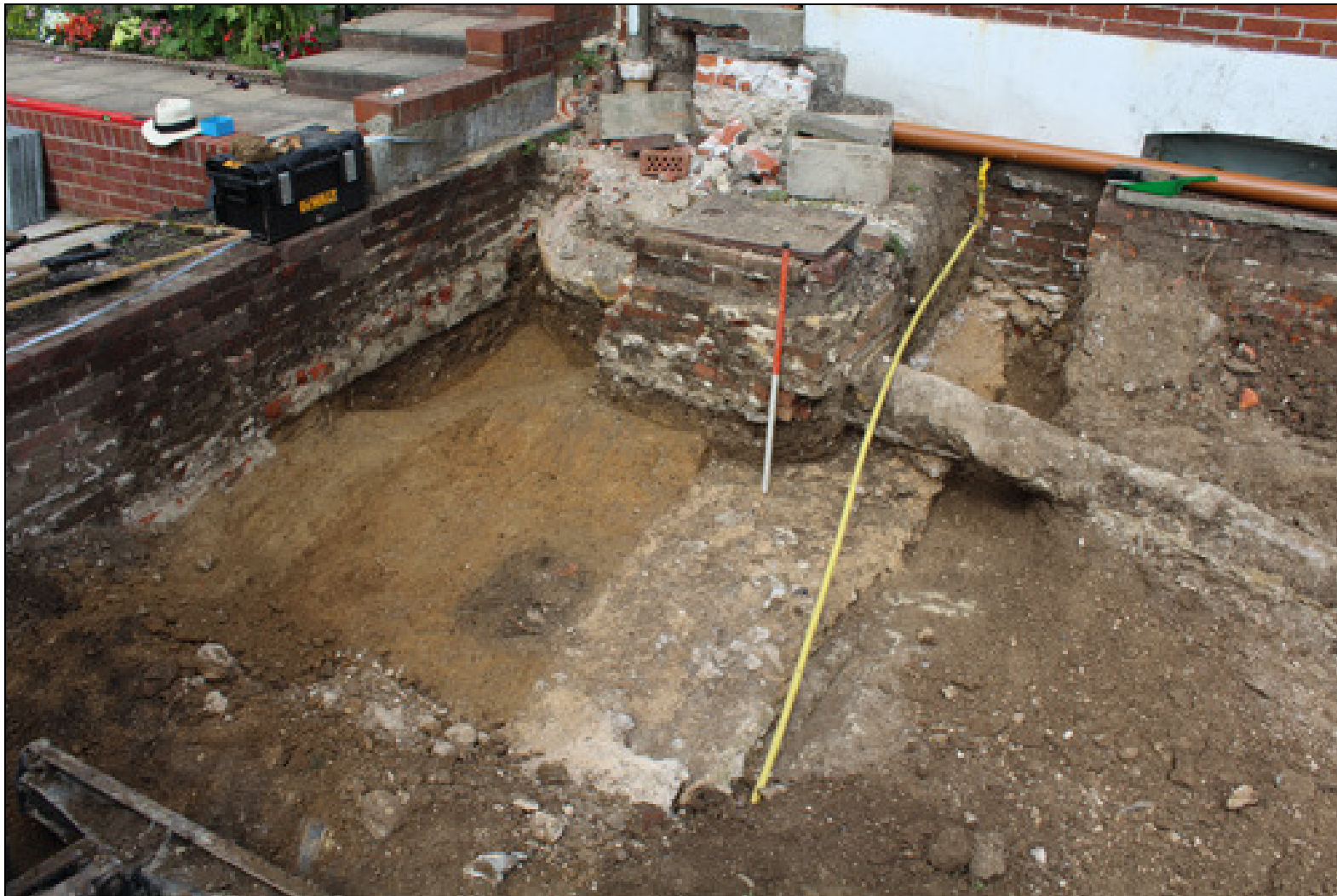
Figure 5 The northern part of the excavated trench, looking north-west and showing the pit [14] and post-hole [12]
