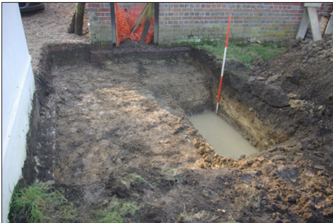
Figure 5 Trench 2, looking west. The scale is 2m.
