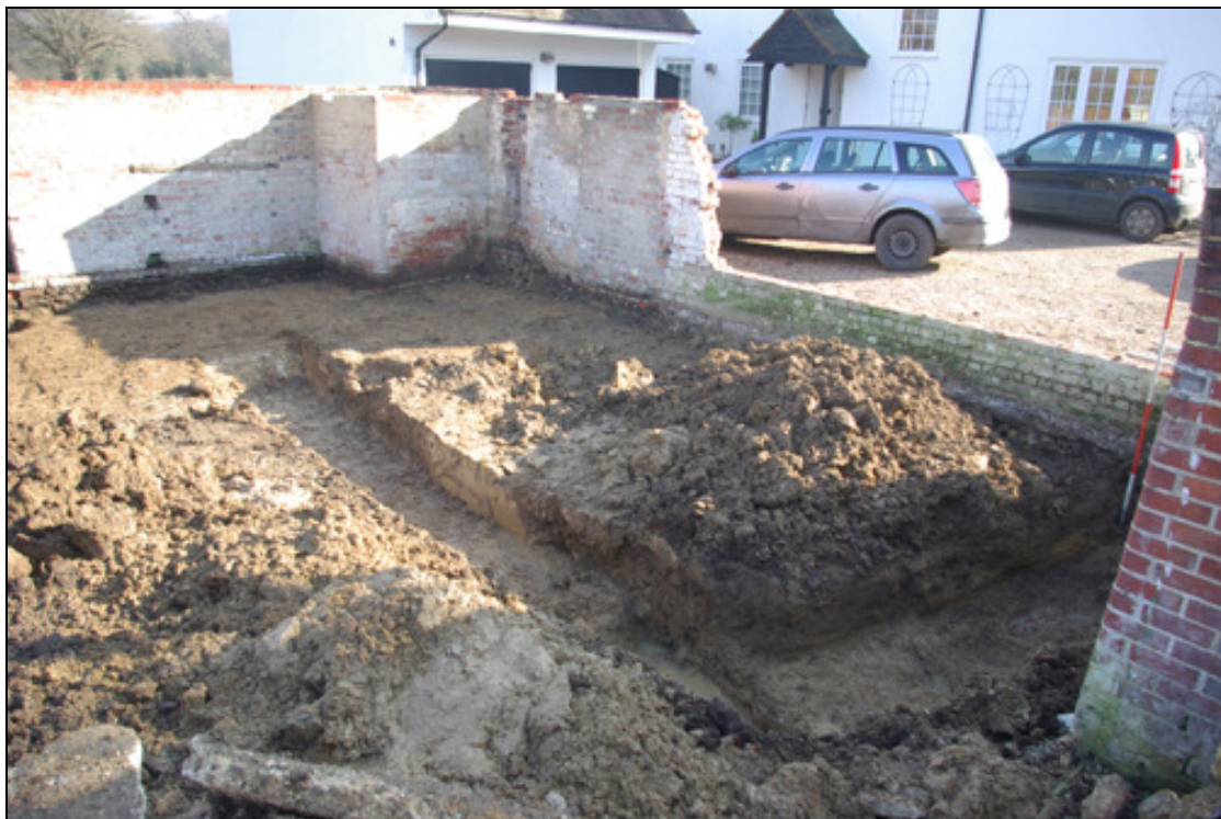
Figure 3 Trench 1, looking south-east. The scale is 2m.
