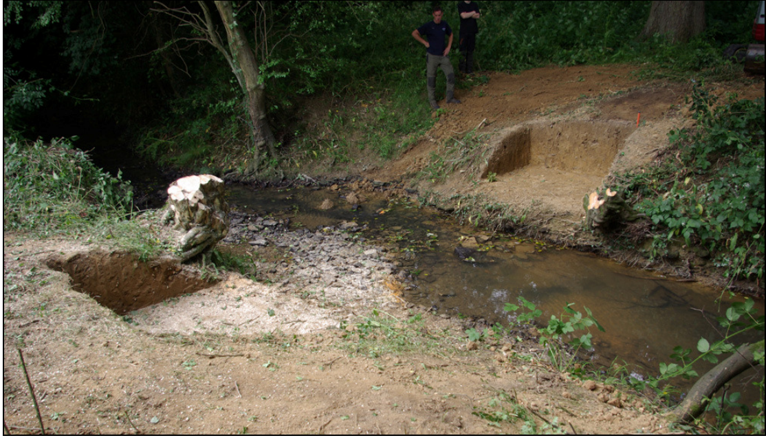
Figure 4 Bridge 1 looking south. The scale is 1m.
