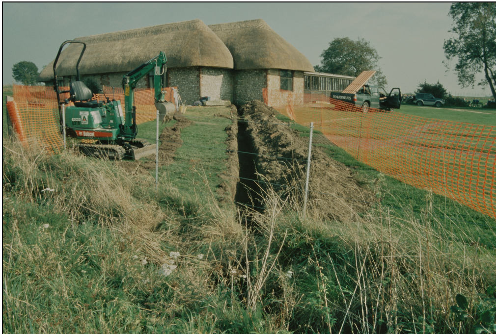
Figure 12 The drain trench, looking towards the cover buildings from the south-west.
