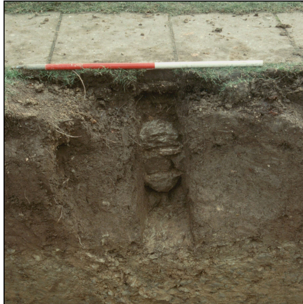
Figure 11 The south wall of Room 13 seen in the extension to the soak-away trench, the scale is 1m.
