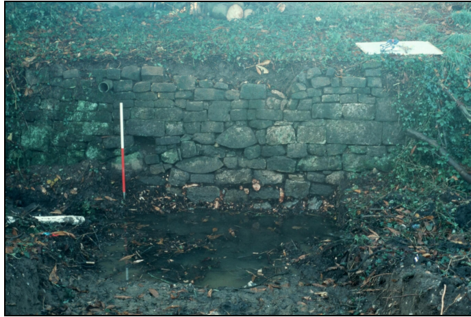
Fig.16 Photograph of the ha ha wall in trench 5, looking west. The scale is 1m.
