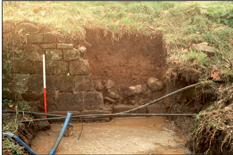
Fig.10 Photograph of the ha ha wall in trench 3, looking west. The scale is 1m.
