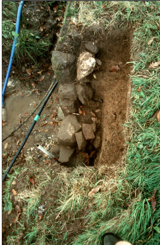
Fig.15 Photograph of the ha ha wall in trench 4, looking south, showing the original construction. The scale is 1m.
