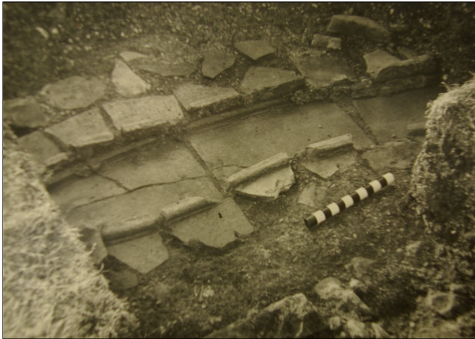
Figure 5 The tile culvert in Cunliffe's Trench 64, looking north-west, the scale is 1 foot. (FRP photo ref: FB61-23-14).
