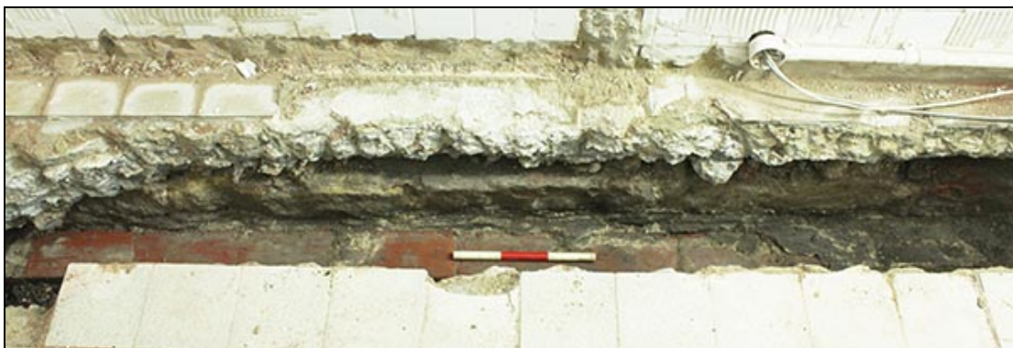
Figure 6 The early 19 th century stone wall (behind the scale) and brick sleeper wall (under the scale) in the western trench, looking north-west
