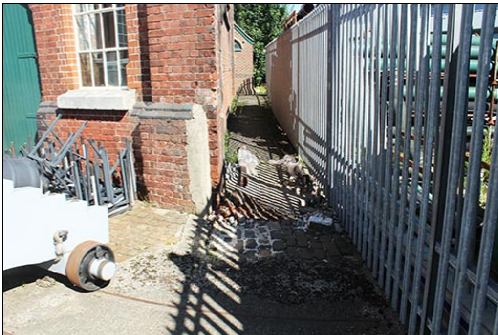
Figure 6 Post-holes 11 & 12 either side of the passageway running north-west alongside the Boiler House
