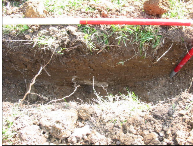
Fig.7. Photograph showing the remains of the wall foundations 102 , looking south. The extreme narrowness of the trench made it difficult to get good photographs of any of the sections.
