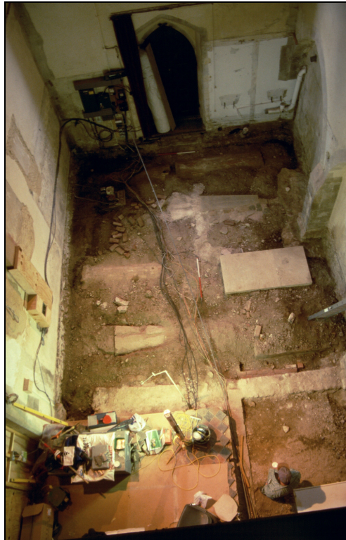
Fig. 8 Photograph of the North Transept looking north from the tower.
