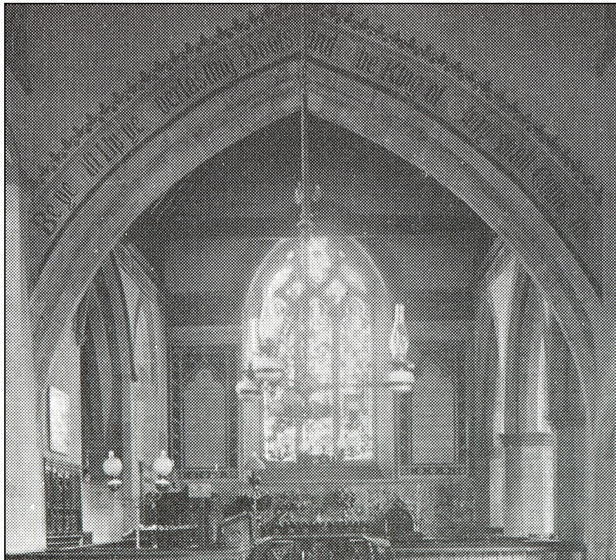
Figure 6 19th century photograph of the chancel, showing the wall paintings.
