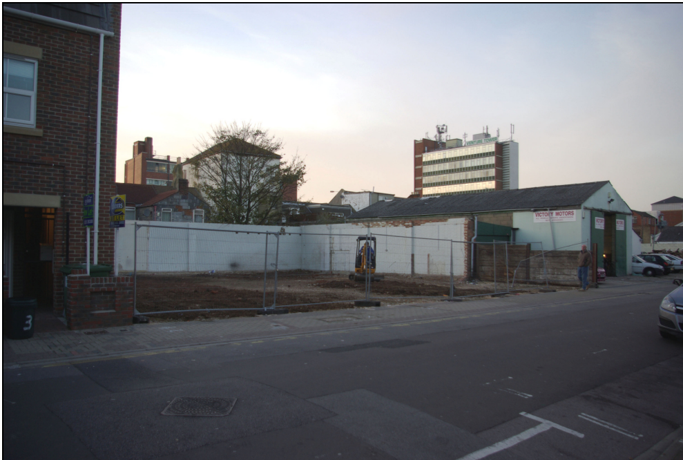
39 – 47 Claremont Road, Portsmouth, looking north-west.
