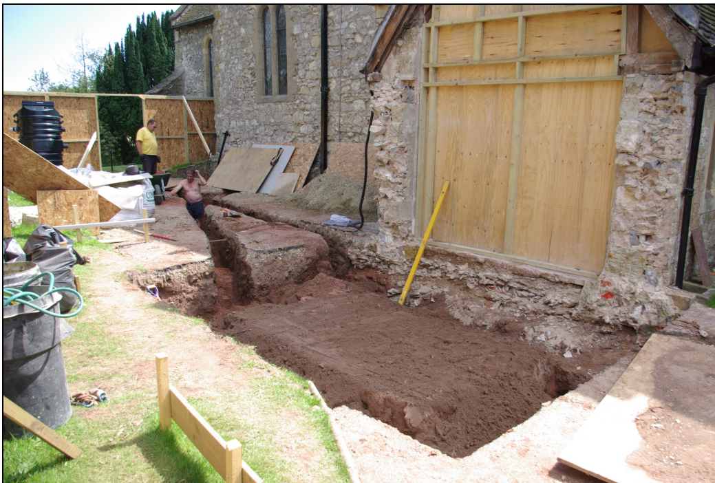
The excavated area, looking south-east.
