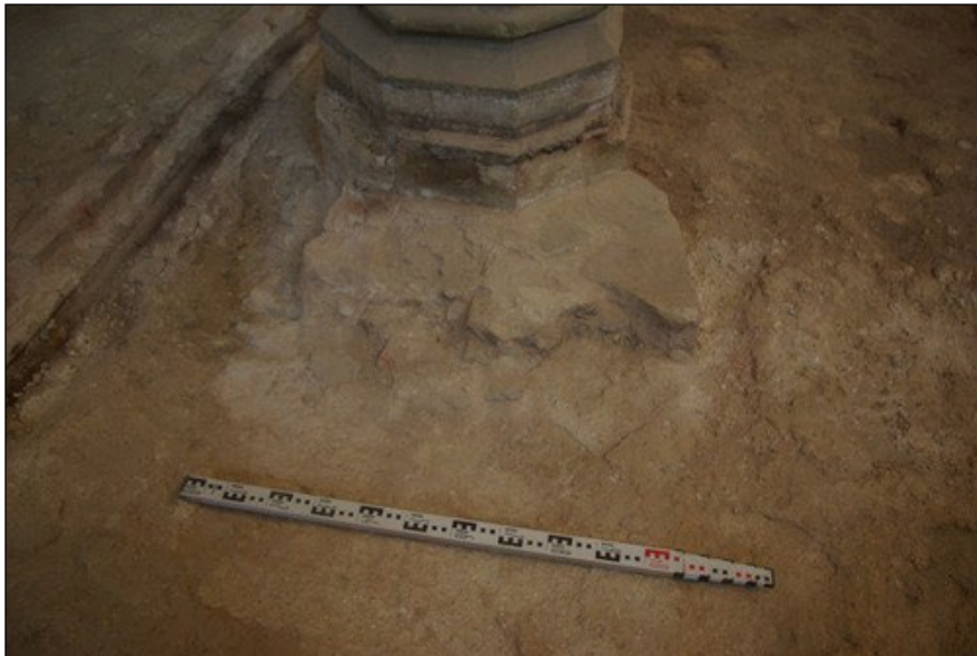
Figure 7 Base of the north-west column within the nave, showing the earlier stonework, looking east. The scale is 1m.
