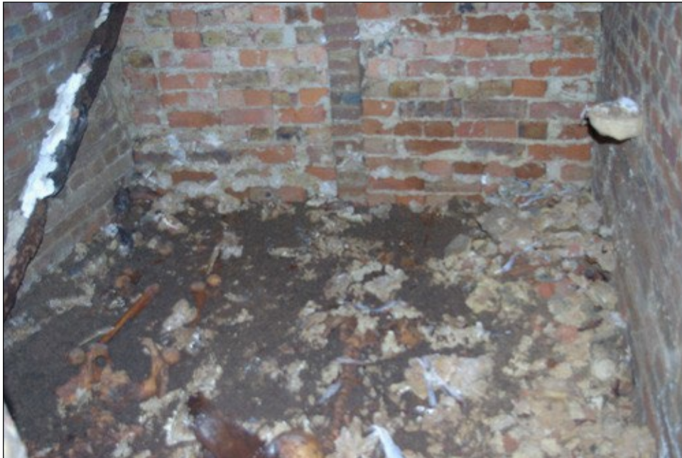
Figure 10 The interior of the De La Warr vault.
