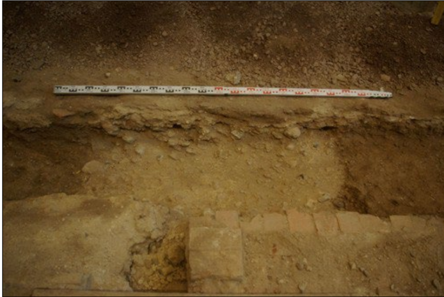
Figure 6 Wall foundation in the southern beam trench, looking south. The scale is 2m.
