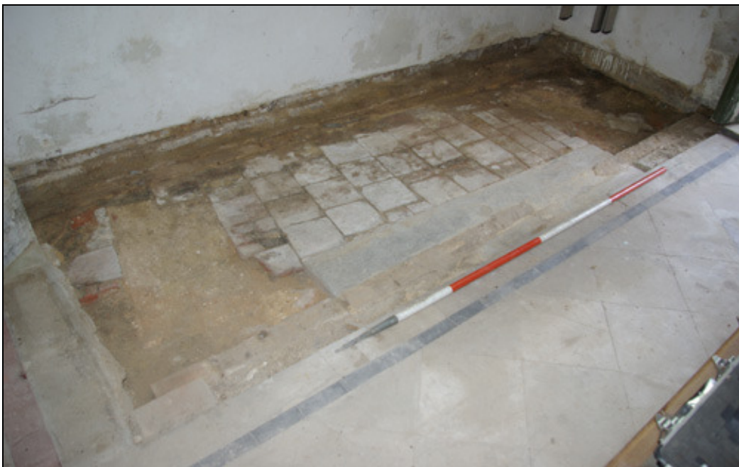
Figure 17 The southern trench in the tower, looking south-west. The scale is 2m.
