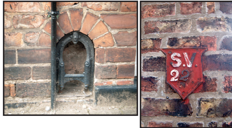
Surviving boot scraper from Acomb terraces (left) and sluice valve marker from Poplar Street (off Poppleton Road).
