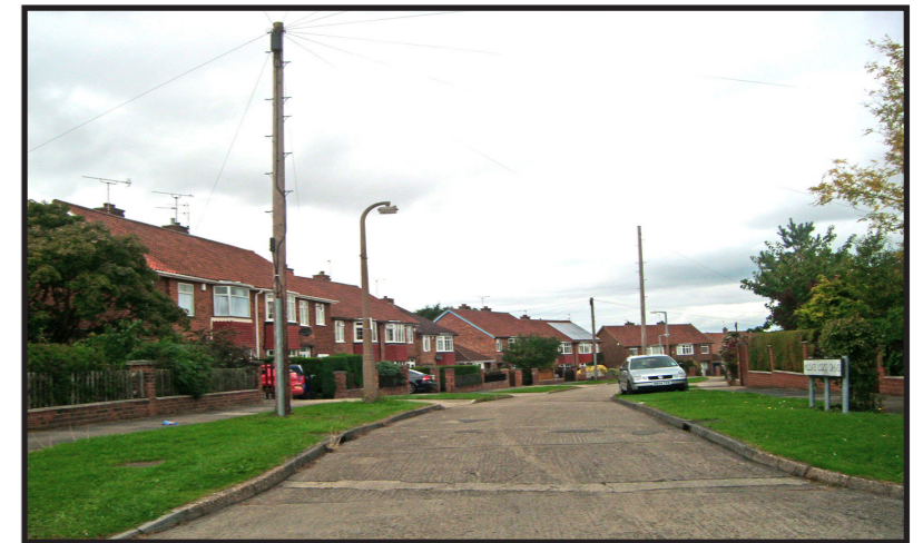
Post-war housing on Holgate Lodge Drive
