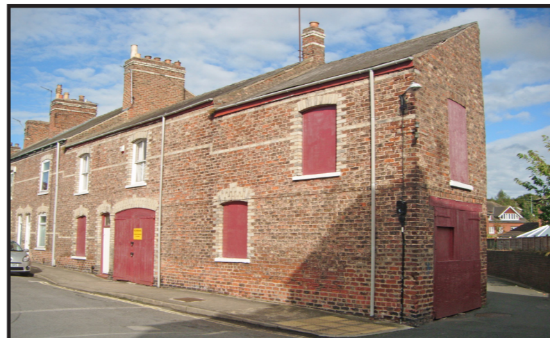
Old loading building in Acomb Terraces
