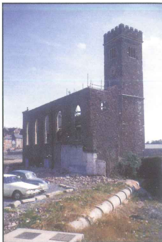
St Edmund's church prior to final demolition, c.1974.
