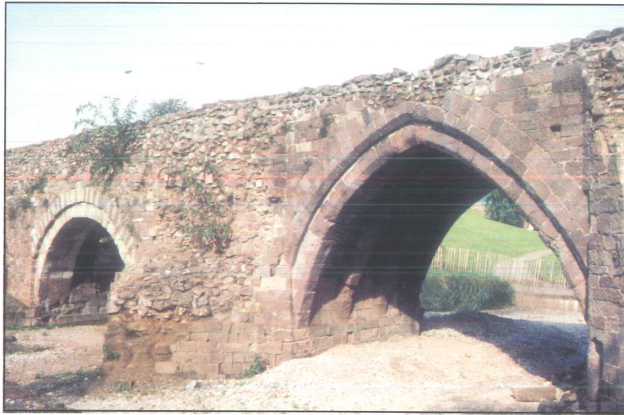
Alternating pointed and round arches, showing their different forms.
