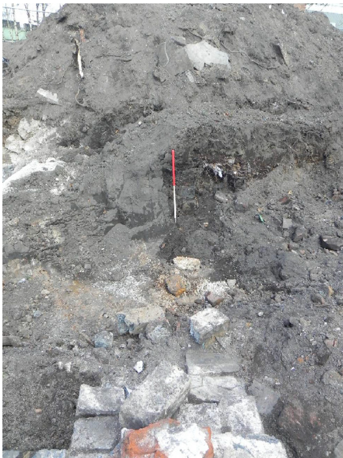
Plate 13. Continuation of wall foundation 8 showing damage by drainage system mid-section and in situ slag block in far eastern trench section (marked by ranging rod). From the west.
