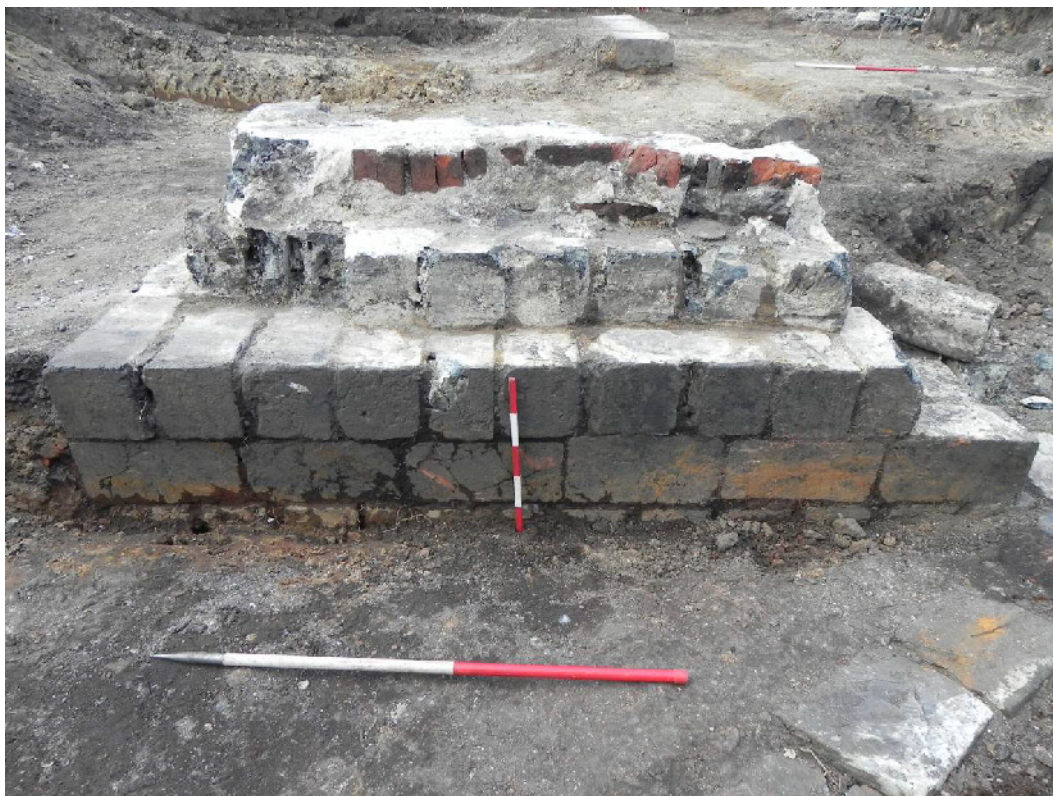
Plate 11. Stepped, rectangular foundation block showing contexts 8 and 9, external facing. From the south.
