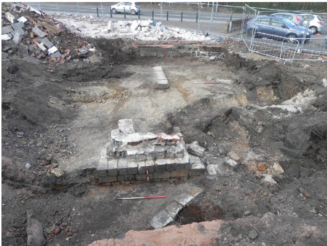
Plate 1. Area of excavation after the removal of context 1 showing slag block foundations and northern extent of the fishpond marked by curving line of blocks at the foreground. View from the south.
