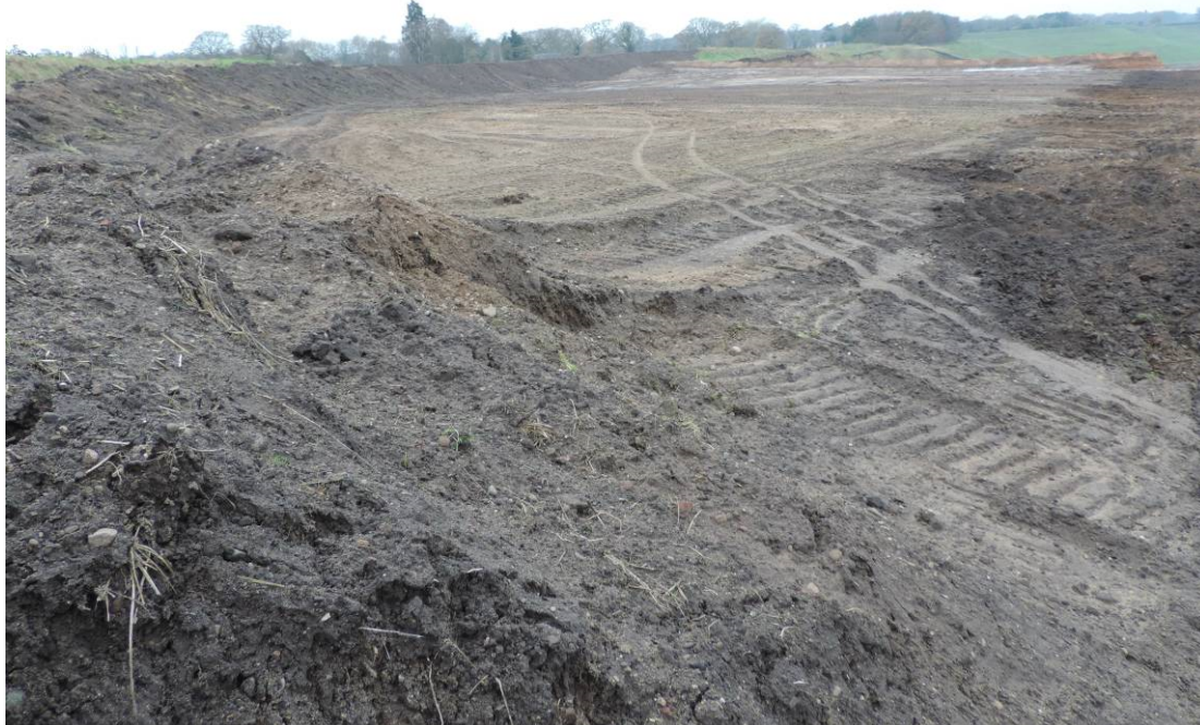
Plate 14. Far south-eastern corner of topsoil stripped area. From the north-east.
