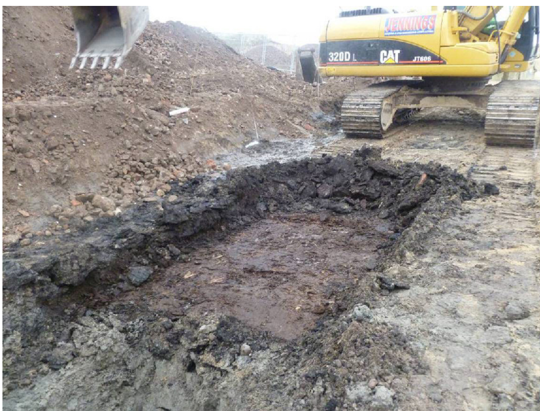
Plate 4. Machine excavating through peat, when initially exposed observed as a very compact dark reddish brown fibrous deposit before rapidly oxidising to black. From the north-west.
